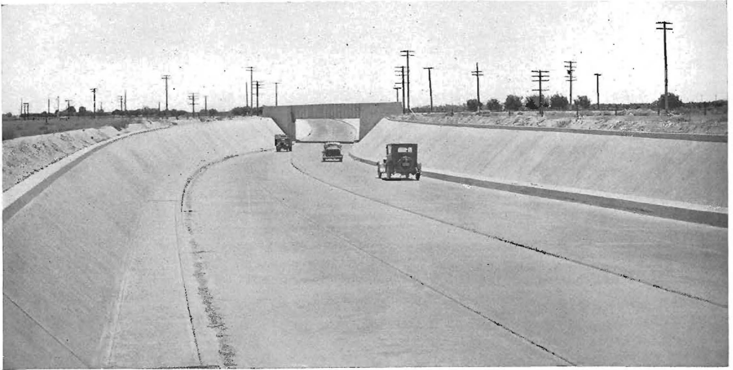
Delano Underpass recently opened to traffic on U. S. 99 provides four 10-foot traffic lanes.
