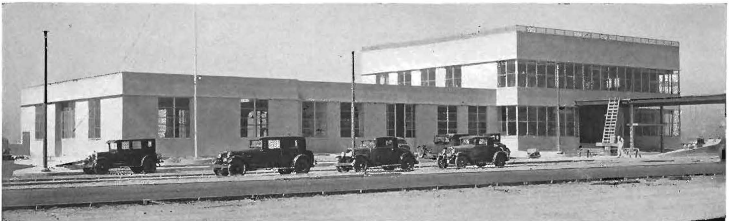
Headquarters for Bridge Patrol, executive offices and a garage are housed in 3-story and basement Administration Building 185 feet long by 70½ feet wide, built entirely of concrete, steel and aluminum.
