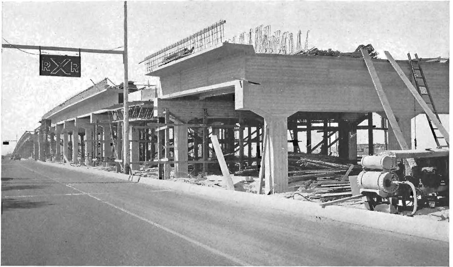
Grade separation under construction at Calwa, near Fresno, on U. S. 99, is 1740 feet over all with cantilevered sidewalks.
