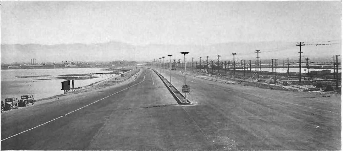
This view of section of East Bay approach to San Francisco-Oakland Bay Bridge shows one type of divided highway where a central raised strip is used for illumination standards.
