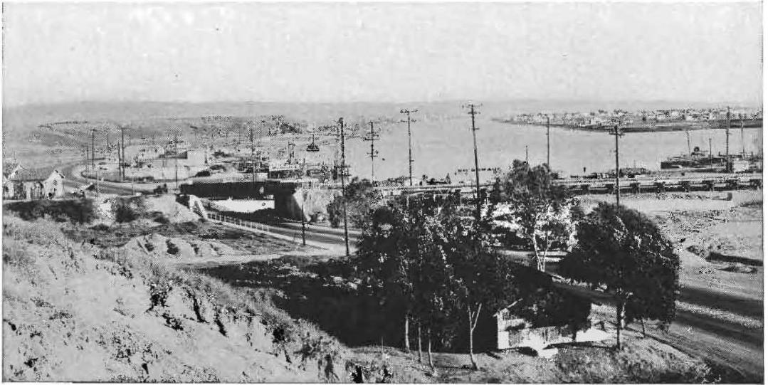
GRADE SEPARATION SITE of Newport Beach project. The Coast Highway passes building in foreground and extends southerly around Newport Bay. Santa Ana road crosses just beyond railroad overhead.
