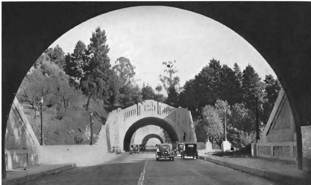
Tunnel Vista showing three completed Figueroa Street bores through park.
