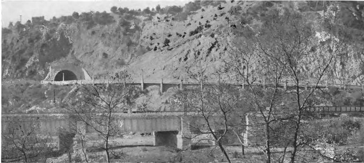
Tunnel Portal at Elysian Park and Riverside Drive where viaduct will connect.
