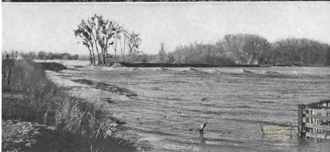
OVER THE TOP of a low levee and through a resulting breach went flood waters of the Sacramento River near Colusa in the January storm. The levee had not been completed to grade and was weakened by rodent holes. In top picture State Engineer Edward Hyatt (left) and Col. A. M. Barton, manager of State Reclamation Board are examining the break, of which different views are shown below.
