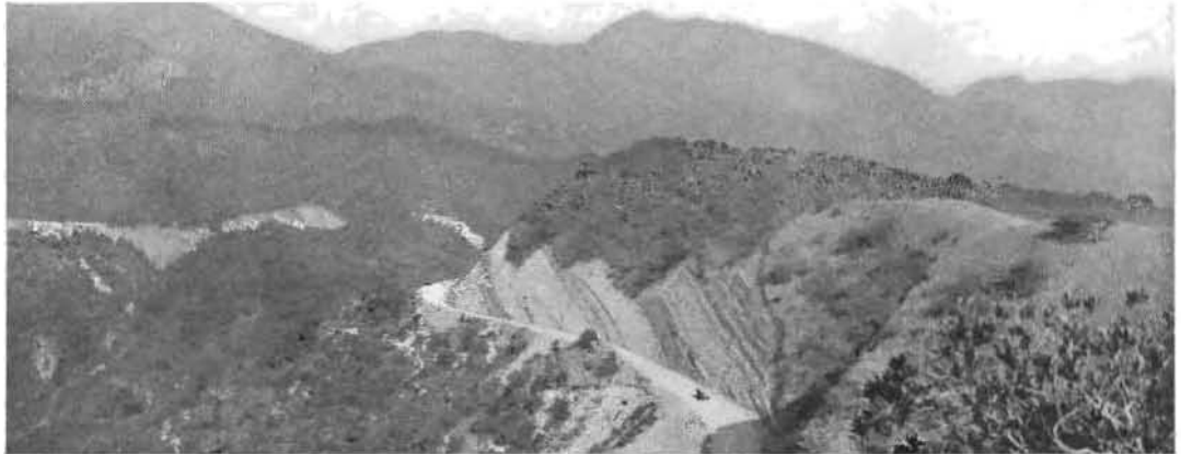
HEAVY SIDE HILL CUT one of several that permitted elimination of hairpin turns and steep grades.
