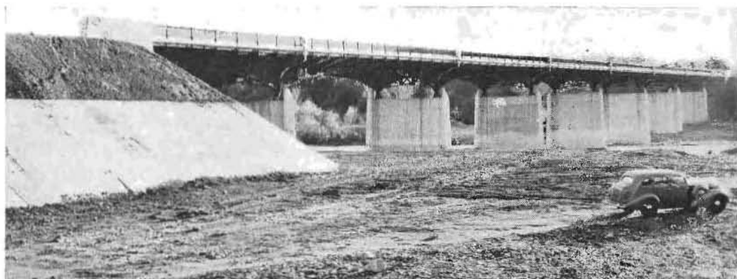
RIVER VIEW of the new steel girder type bridge consisting of six 108-foot continuous plate-girder spans and two 45-foot cantilever end spans on concrete piers.
