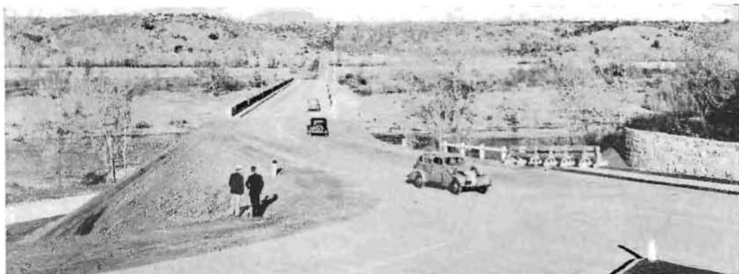
STRAIGHT ACROSS THE SACRAMENTO at Redding goes the realigned State highway over a new 795-foot bridge with a 34-foot roadway and wide, easy approaches.
