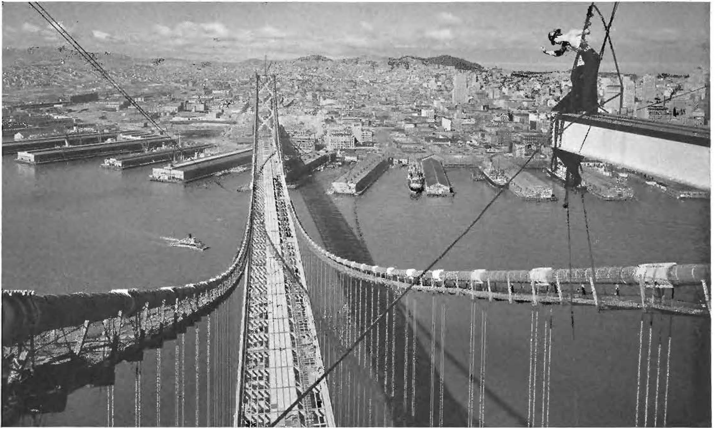
View of West Bay Crossing of San Francisco-Oakland Bay Bridge looking toward San Francisco showing paving laid on center lane.
