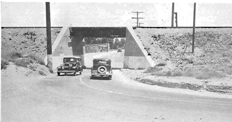
Old subway built on reverse curve alignment and too narrow for two trucks to pass.
