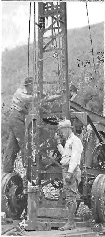
Cuesta Grade Realignment Project. No. 1—Existing highway showing numerous sharp curves. Nos. 2-3—Traffic congestion behind slow moving vehicles. Nos. 4-5—Boring and testing to determine earth structure on new alignment.
