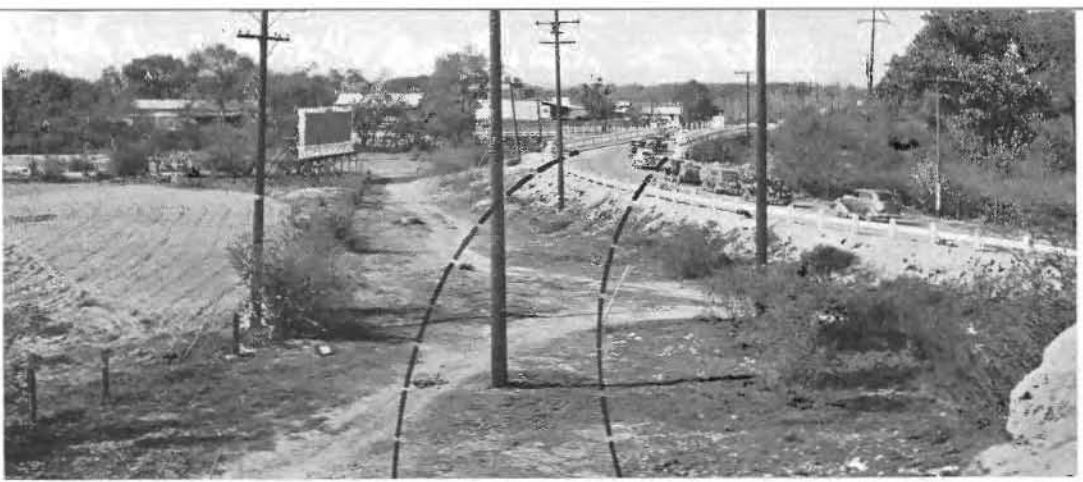
DANGEROUS CURVE at south end of Santa Ana River bridge east of Colton to be replaced by a sweeping, easy curve as shown by dotted lines.
