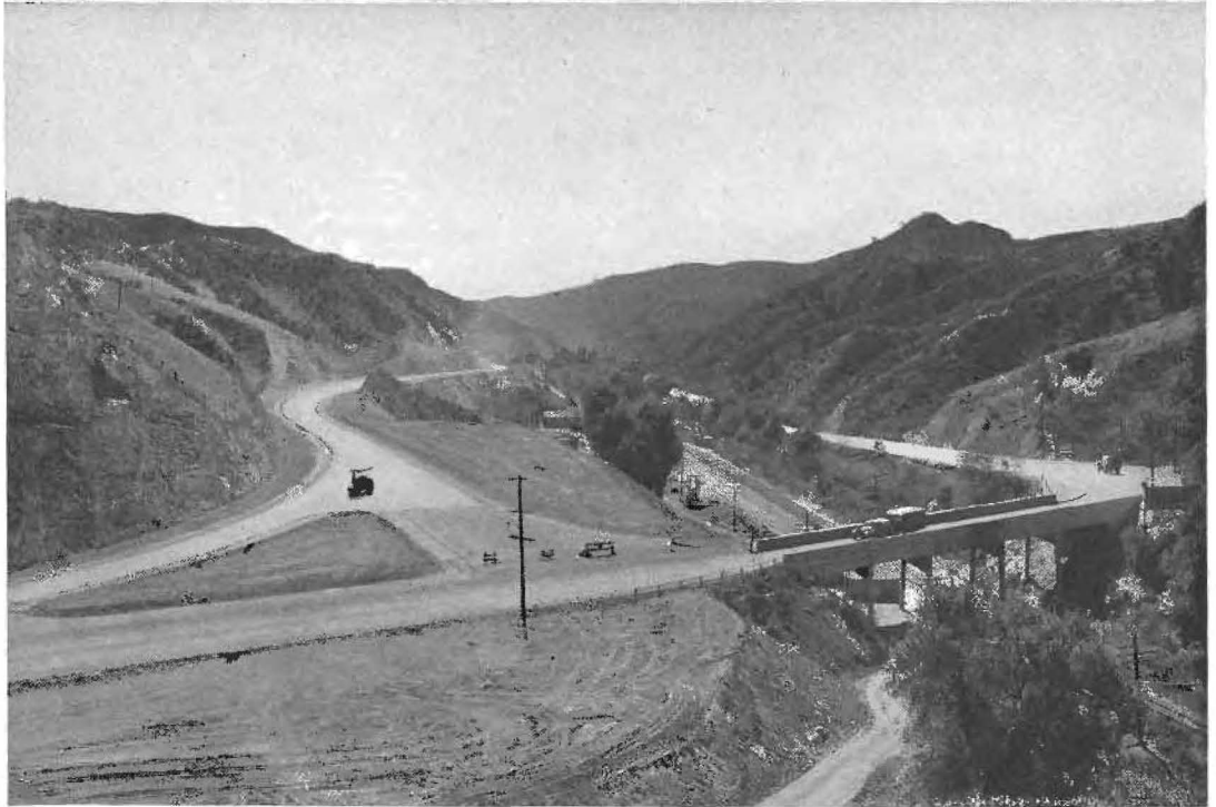
AN IMPORTANT BRIDGE RECONSTRUCTION PROJECT recently completed at Tunnel Station on State Route 4 connects this Los Angeles-Sacramento main highway near its entrance to Weldon Canyon with the Newhall-Saugus route and the Foothill Boulevard cut-off near San Fernando. The widened rebuilt structure is shown at top and below the narrow old structure.
