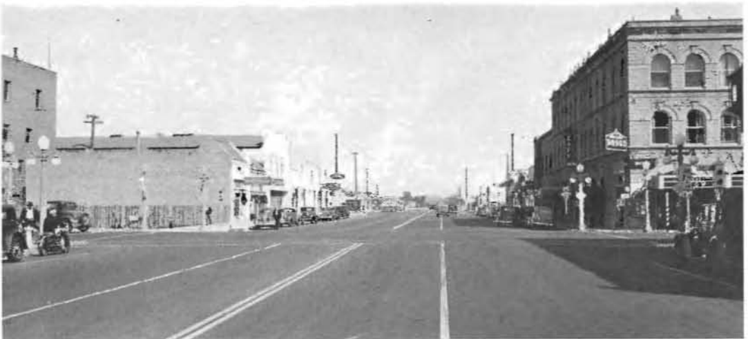
THROUGH CITY OF COLTON , the State Highway follows I street, which has recently been widened to provide four traffic lanes in addition to an ample strip for parallel parking.
