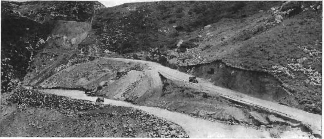
CONEJO GRADE REALIGNMENT —Left foreground, constructing base for big fill which will cover old highway. Upper left, new cut.
