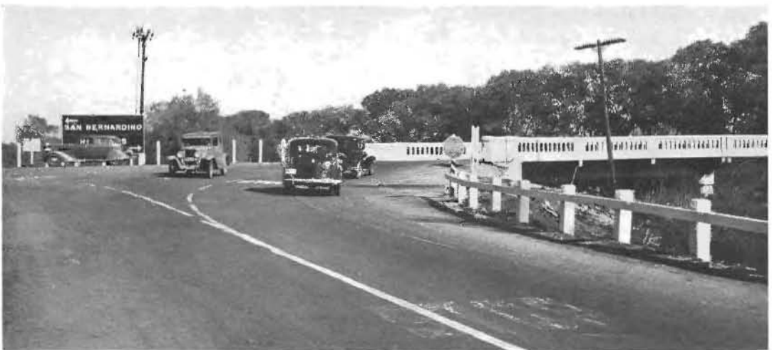
ANOTHER SAFETY FEATURE of the Redlands-Colton relocation will be elimination of this sharp turn at the north end of Santa Ana River bridge, leaving a straight approach for traffic from San Bernardino.
