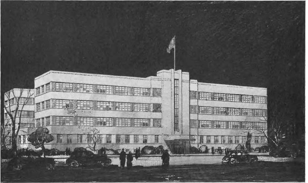
DIGNITY AND BEAUTY characterize the simple modern design of the new Public Works Building under construction in Sacramento, a 4-story reinforced concrete structure with provision for a fifth story. Drawing by A. W. Eichler
