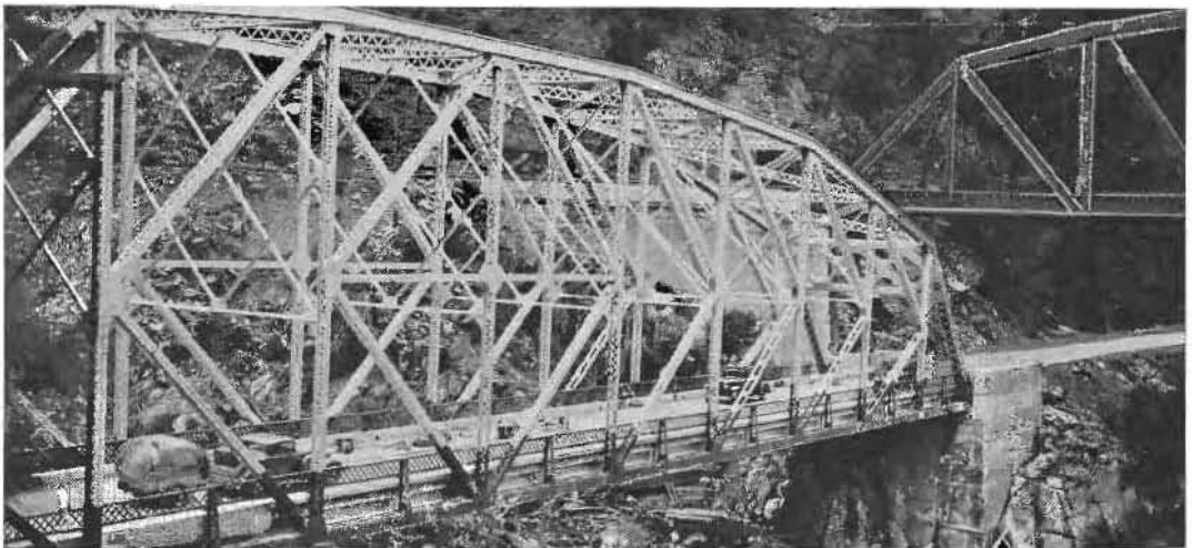
TOBIN BRIDGE , dwarfed in above picture, is larger than railroad structure, being 290 feet long, 24 feet wide.
