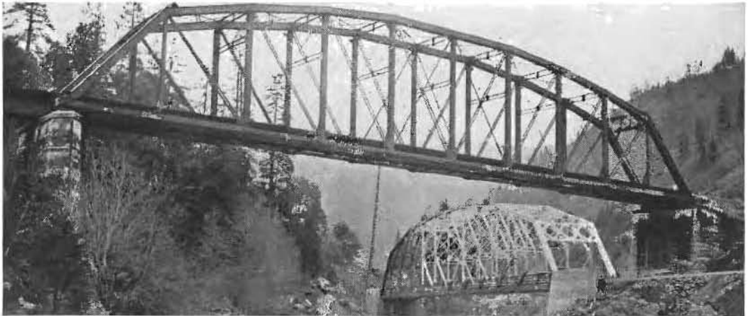
TURN ABOUT FAIR PLAY —Recently completed highway bridge crosses almost below railroad bridge at Tobin, 14 miles away.
