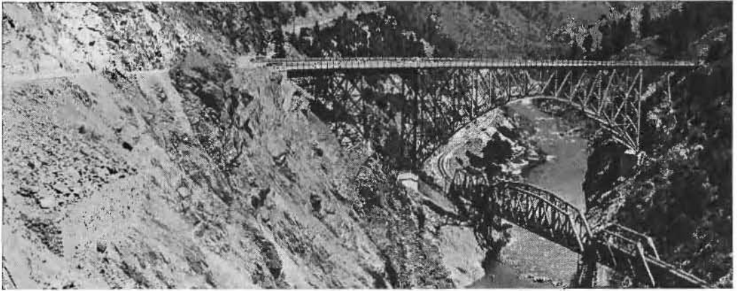
BRIDGES PLAY LEAP FROG —New State Highway crosses Feather River above railroad structure at Pulga.
