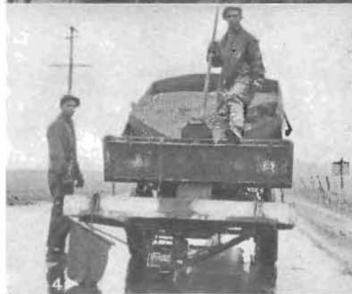
SAFETY FOR ICY PAVEMENTS —No. 1—Stock piles of sand and salt are stored in galvanized shelters at convenient locations. Nos. 2, 3—Disk spreader equipment attached to rear end of truck. No. 4—On the job with distributor actuated by drive-wheel. No. 5—Sand is purchased by the carload.
