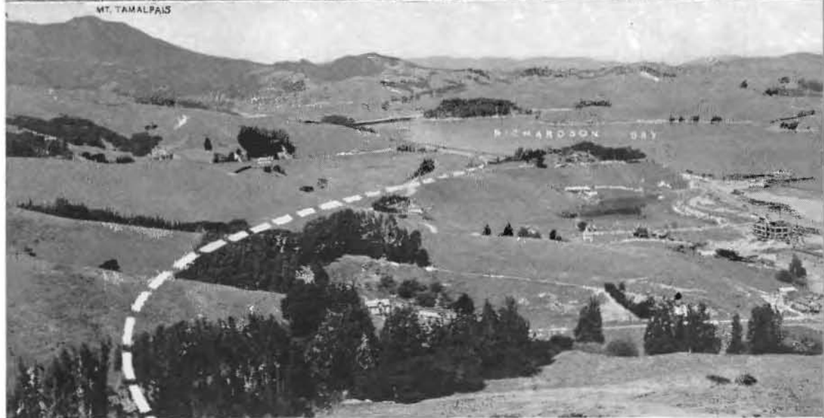
MARIN APPROACH alignment to Golden Gate Bridge through rugged Sausalito hills is shown by dotted lines. At top—Location of tunnel through high ridge. Center—General view of route from Bolinas Street. At bottom—Alignment from present State Highway at Waldo Point and Richardson Bay.
