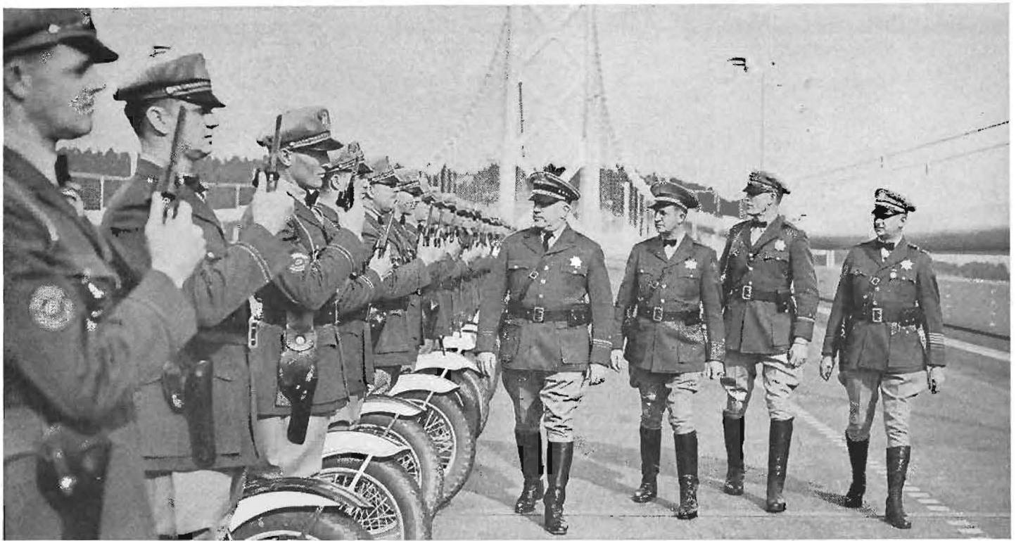
Bridge Detail of Highway Patrol being inspected by (left to right) E. Raymond Cato, Chief of California Highway Patrol, District Inspector A. J. Ford, Captain Rudolph Schmoke and Captain A. Paquette.
