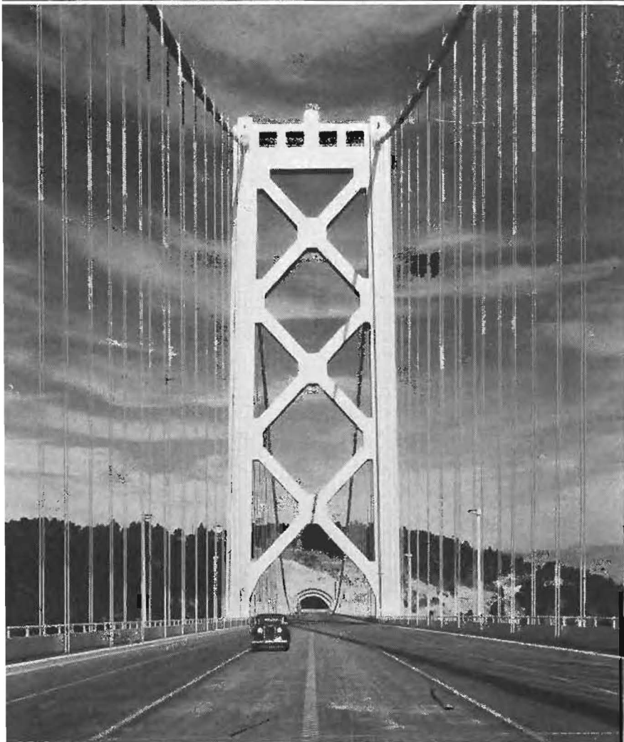
AT RIGHT View of lower deck showing three truck lanes.
