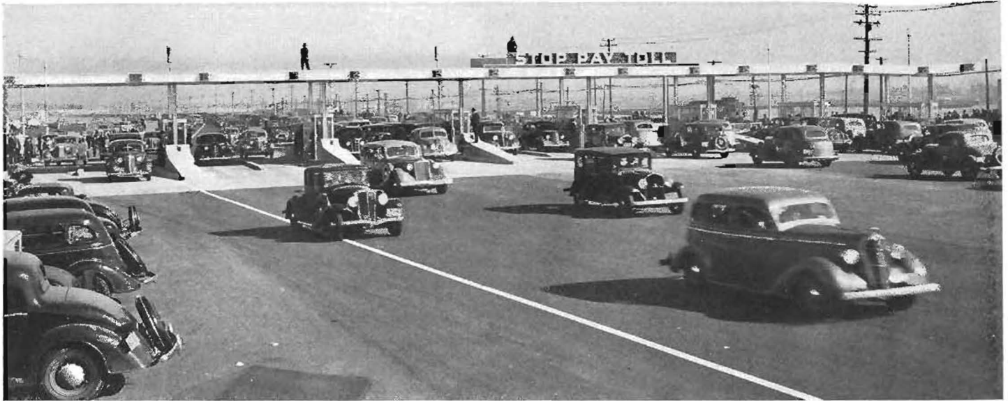
The San Francisco-Oakland Bay Bridge is open for business! Photograph shows automobiles leaving toll station on Oakland side and machines from San Francisco arriving there shortly after President Roosevelt in Washington flashed by wire the "Go" signal on November 12.
