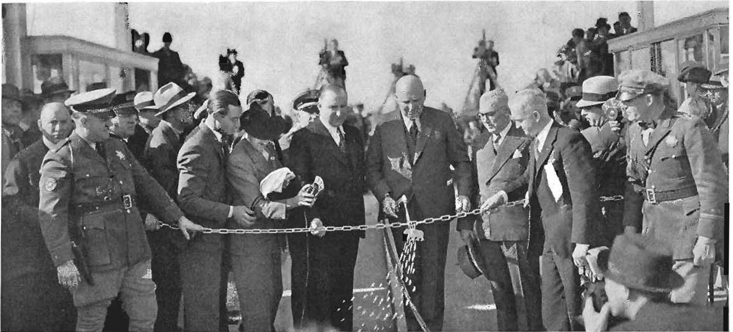
Flanked by Earl Lee Kelly, Director of Public Works (left) and Chief Engineer C. H. Purcell (right), Governor Frank F. Merriam burns first barrier on Oakland side of Bay Bridge.
