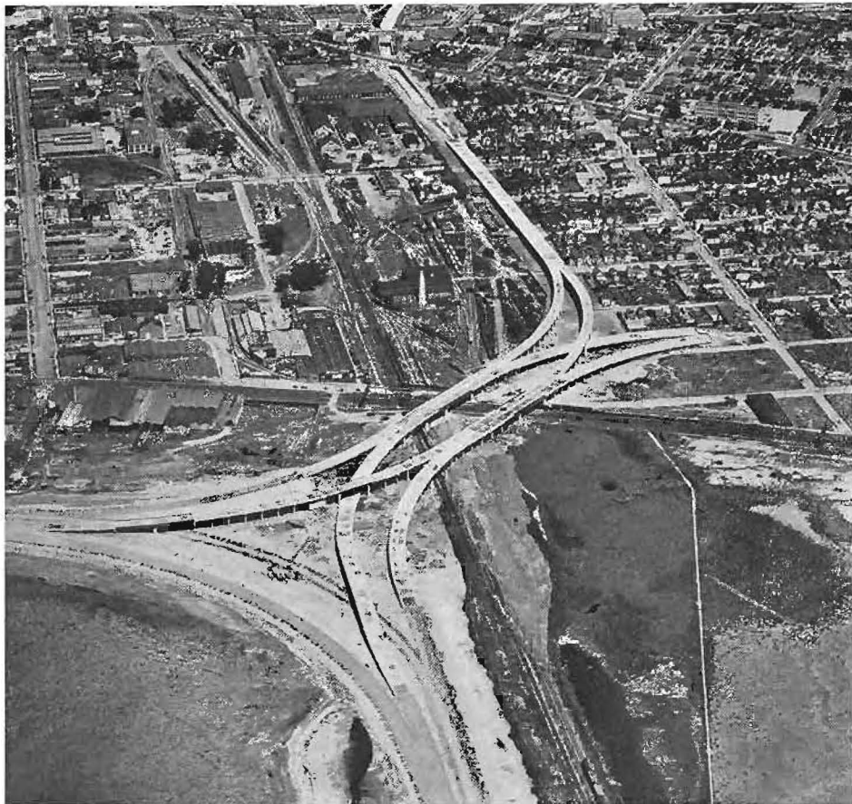
Aerial view of intricate East Bay distribution structure showing how traffic problems were solved. The two roadways leaving the structure in the immediate foreground lead directly to the bridge approach.
