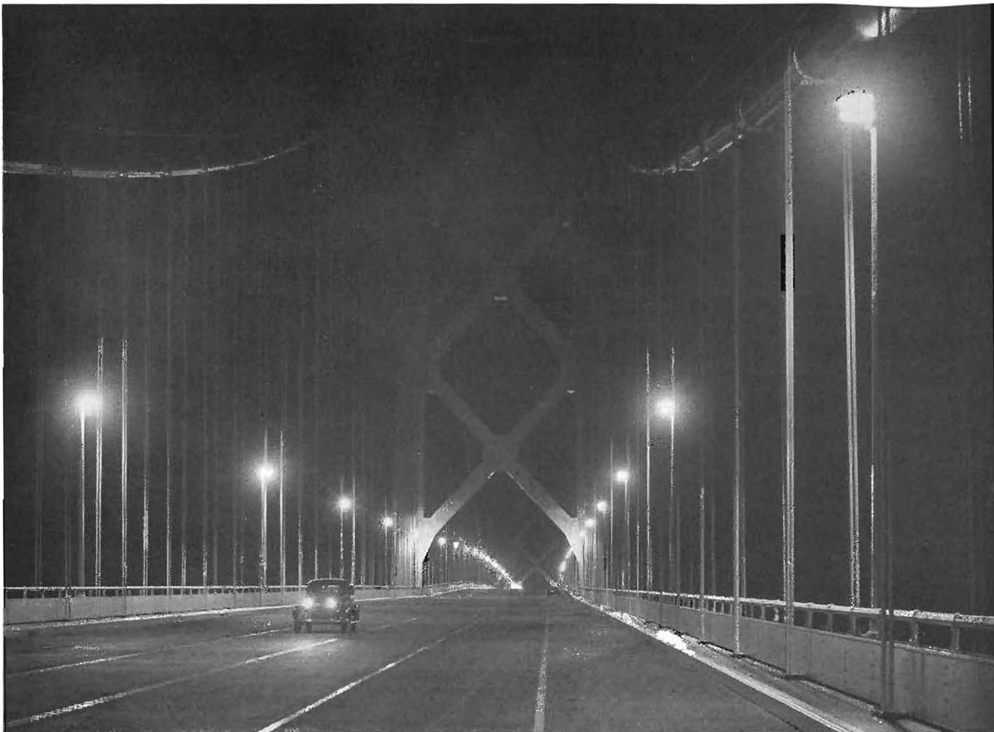
This night photograph shows the excellent visibility afforded under all weather conditions by the new sodium vapor lighting system.
