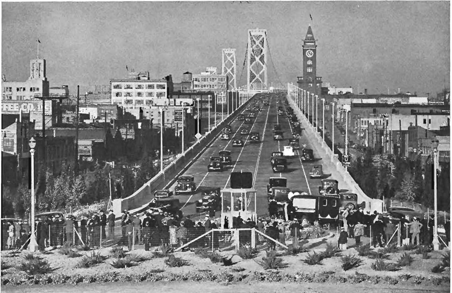
This view looking east on the bridge from the Fifth Street Plaza in San Francisco shows auto traffic coming and going over main western approach.
