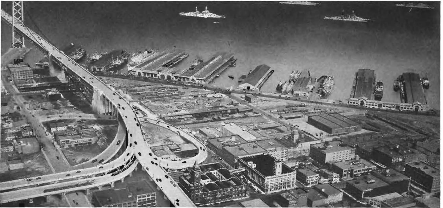
This photograph, looking east from the Fifth Street Plaza in San Francisco, shows the on and off ramps for both upper and lower decks of Bay Bridge. In foreground is the approach to the plaza. The artist has sketched in his conception of interurban trains using the lower deck.
