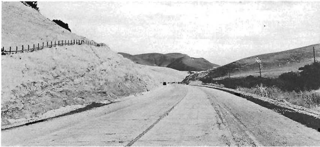
Sweeping view of new American Canyon cut-off between Cordelia and Garquinez Bridge which effects saving of about one hour's driving time to San Francisco from Sacramento City
