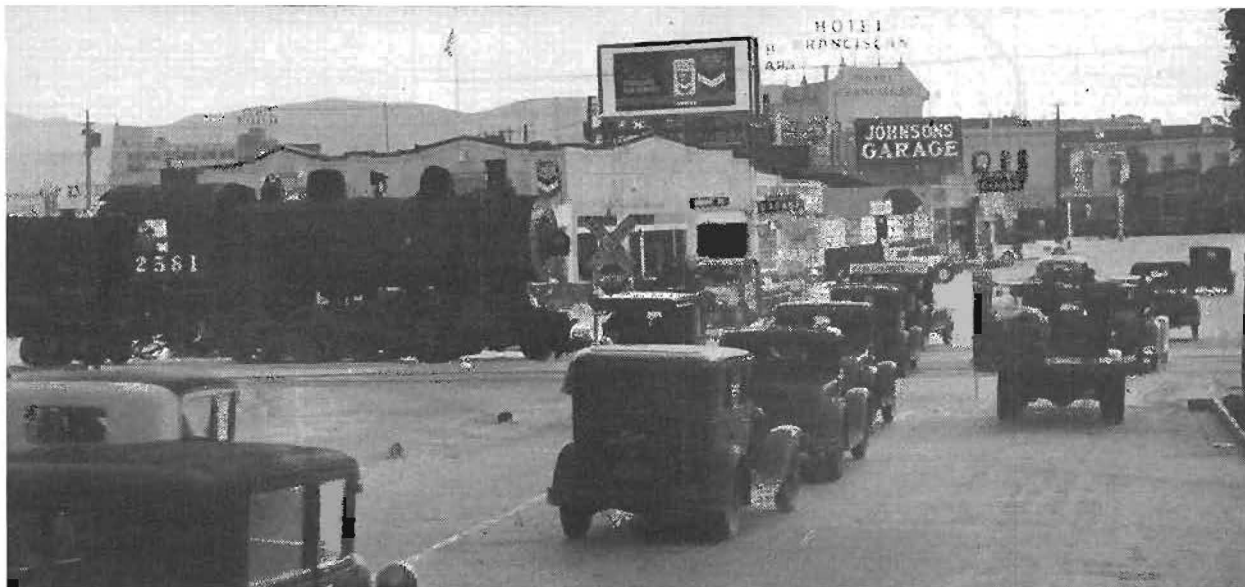
Dangerous old grade crossing in city of Salinas with a daily average record of 35 rail and 7500 vehicular movements across intersection.
