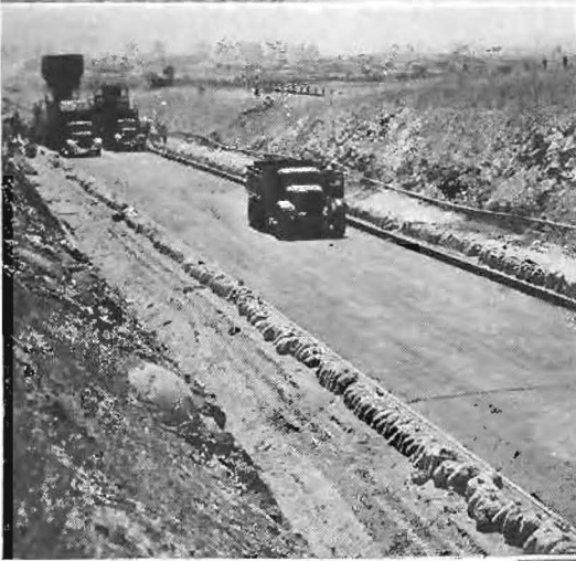
Paving scenes on the American Canyon cut-off relocation of State Highway No. 7 (U. S. 40) from 1 mile East of Carquinez Bridge to Cordelia. The several views show two pavement mixers operating side by side placing a 20 foot width of Portland cement concrete pavement, together with three mechanical tampers in addition to the necessary hand tamping and finishing equipment. A vibrator is being used from each side of the pavement ahead of the first finishing machine. Inset shows subgrade prepared and ready for paving.
