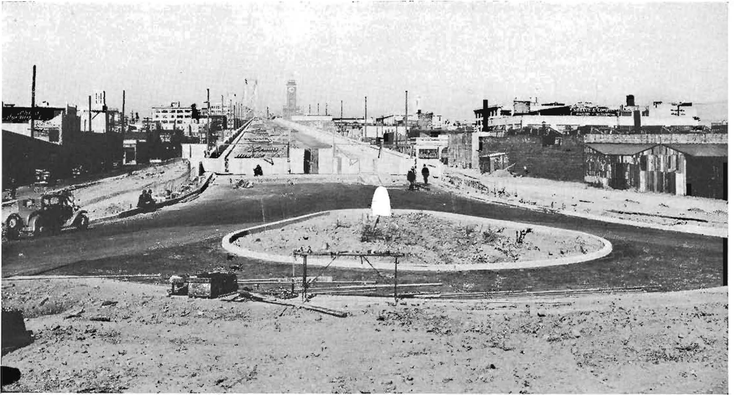
The Fifth Street Plaza terminal of the main San Francisco approach to the San Francisco-Oakland Bay bridge as it is now and as it will look when completed and opened to traffic, on November 12th next is shown in the two pictures presented on this page. The above photograph was taken looking toward the bridge approach across the eastern point of the Plaza triangle for which an attractive landscaping design has been prepared as illustrated below.
