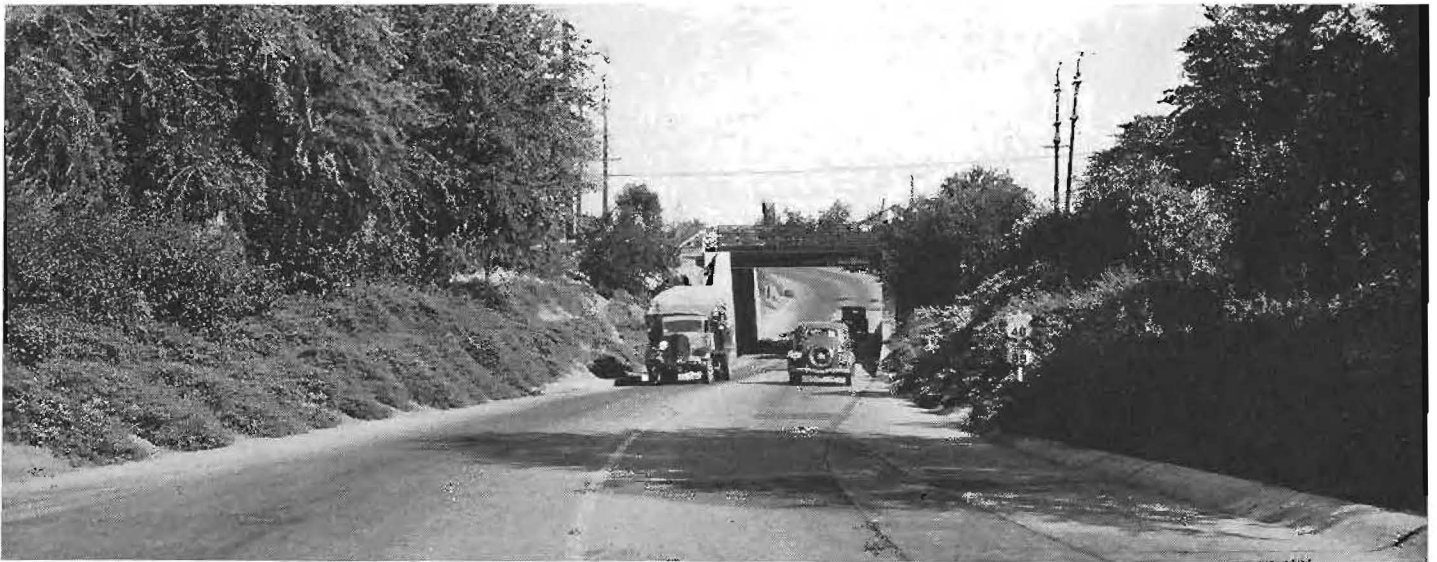
Day photograph of the underpass pictured above shows a wealth of shrubbery and trees on the side slopes presenting a most pleasing arboreal setting as a result of the landscaping of the curved highway approaches over which traffic is guided by the center white line.
