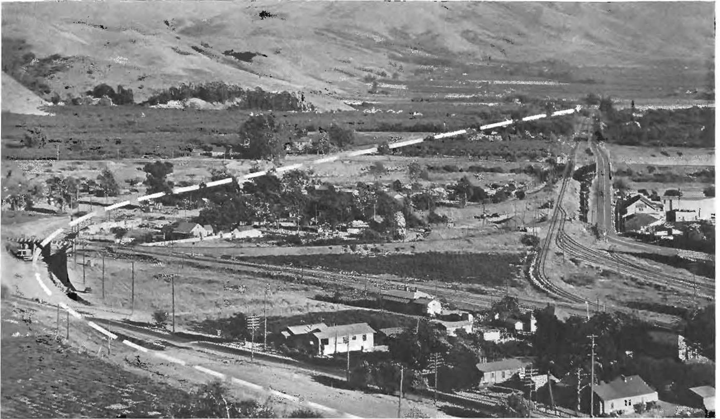
View of Niles area in Alameda County where an extensive grade separation program is under way consisting of six underpasses, a concrete bridge and the relocation of approximately 3 miles of State Route 5, the Santa Cruz-Oakland-Stockton highway as shown by white dotted line.
