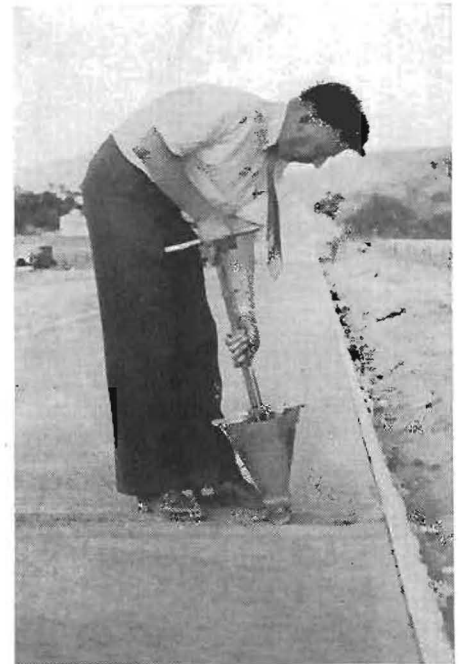
Close-up of one-man pavement joint filling apparatus.
