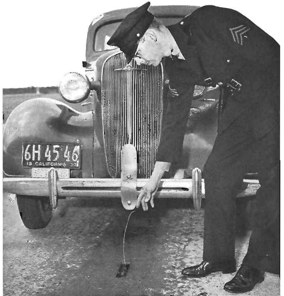
Toll Sergeant J. Y. Borden inspects one of "cat's whiskers" used to reduce electric static in automobiles passing through toll gates of the San Francisco-Oakland Bay Bridge.
