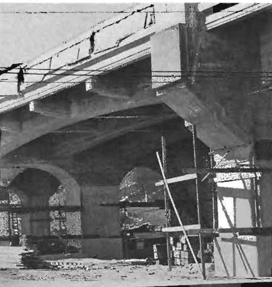
Showing the massiveness of the reinforced concrete construction.
