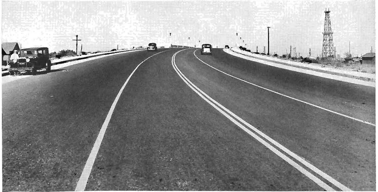
The N and O Street Viaduct in Wilmington in Los Angeles County, shown in upper picture, completes another important link in State Highway 60 and will be an important grade crossing for many years to come. Lower—View of west approach to viaduct showing splendid alignment.
