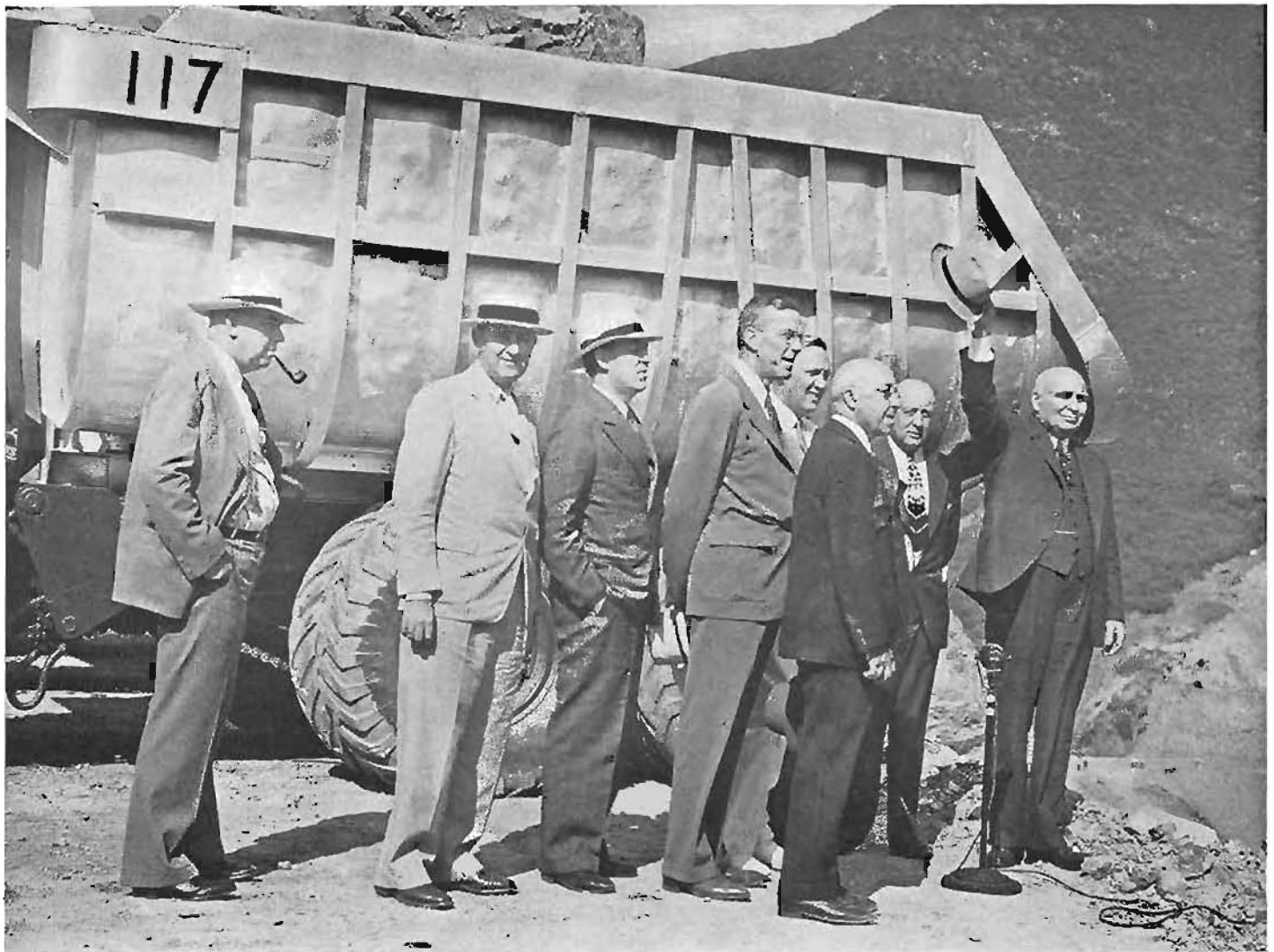
Governor Frank F. Merriam gives signal for dumping of last truckload of rock at dedication of San Gabriel Dam. Left to right: Flood Control Engineer C. H. Howell, Supervisors Leland Ford, John A. Ford, Herbert C. Legg; E. T. Foley and W. A. Rogers, West Slope Construction Co., Supervisor Roger Jessup, Governor Merriam.
