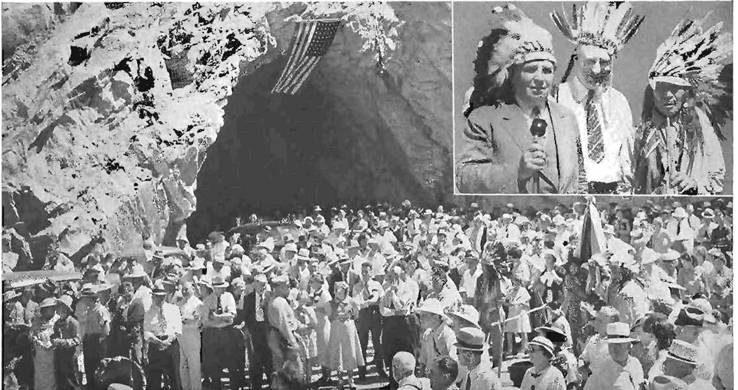
Portion of large crowd of celebrants gathered at portal of Grizzly Dome tunnel to participate in dedication of Feather River Highway—Insert—Governor Merriam, Director of Public Works Earl Lee Kelly and Chief Winnemucca conclude ceremony of smoking pipe of peace.
