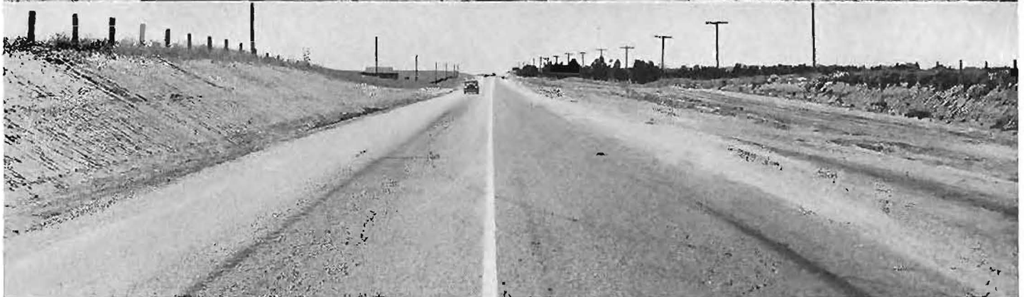
What new jack rabbit trail looks like. Upper—Grade separation overhead at Box Springs near Beaumont. Center left—Deep cut on new highway looking towards Gorgonia Range. Center right—Another view looking towards Beaumont with Mt. San Jacinto in background. Lower—View of realigned highway west of Beaumont.
