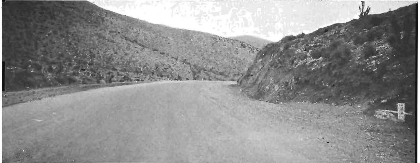
The upper picture shows section of Mountain Pass to Las Vegas route before and after realignment. New road is on the right. Center—Aerial photograph of completed highway through Mountain Pass. Note old road meandering along creek bottom. New highway is on higher ground where it will be safe from floods. Lower—Another view of finished highway.
