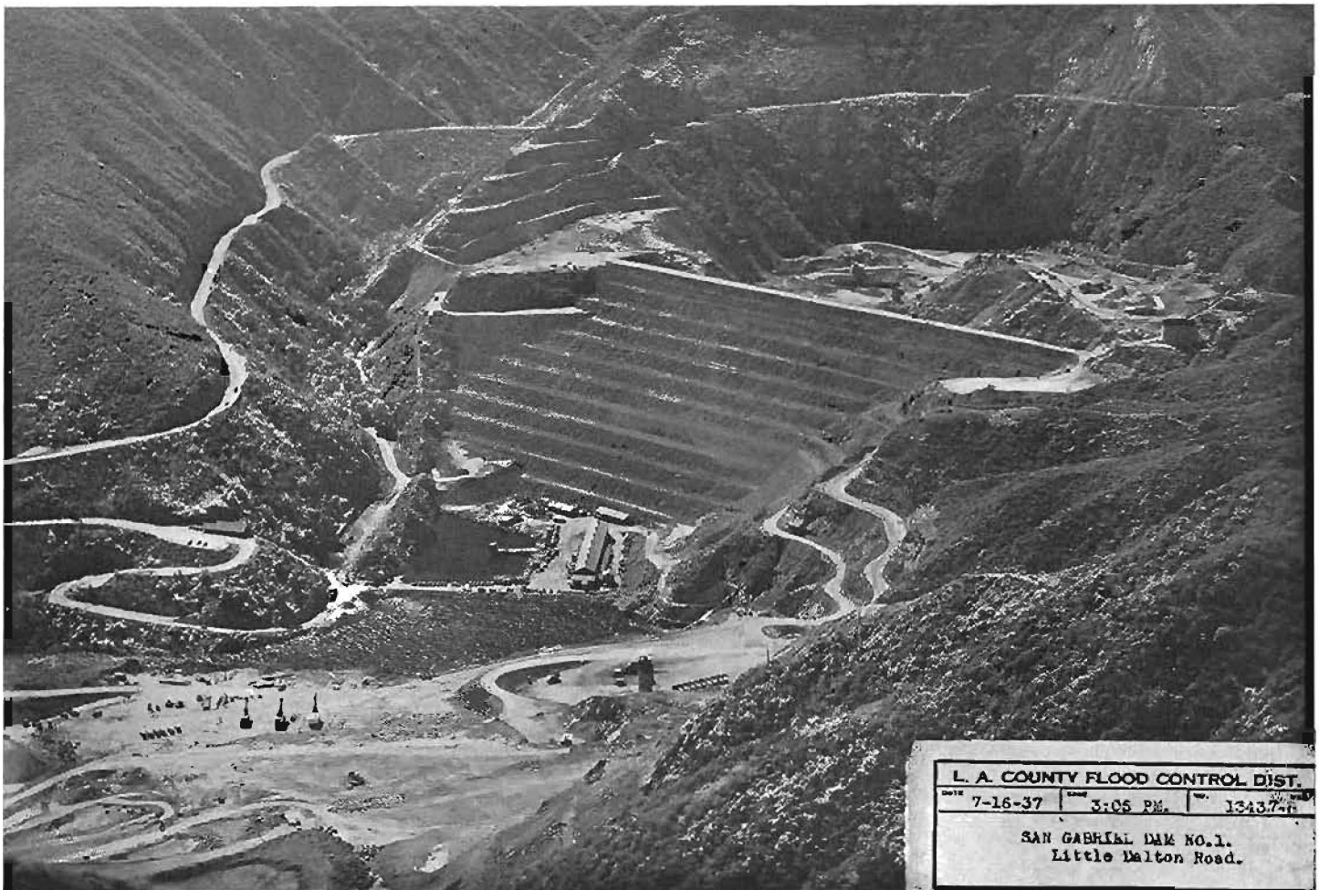
View of San Gabriel Dam No. 1 showing stepped face of dam. This picture shows magnitude of this flood control project, largest earth and rock fill dam of its type in the world.
