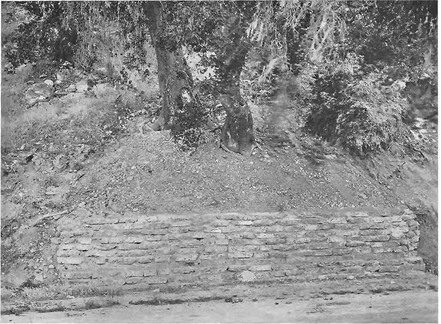
This picture shows how oak trees on highway in Monterey County were protected from erosion by state road builders.
