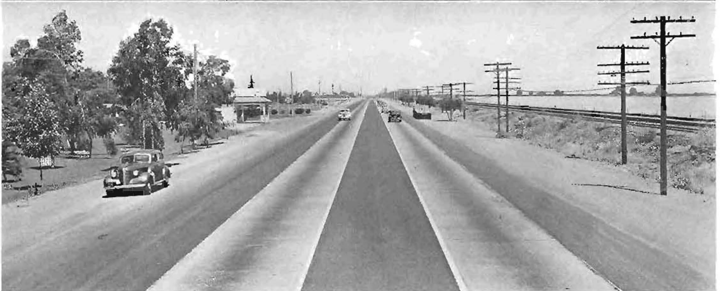
Upper picture shows newly improved section of Route 4 at the north boundary of the city of Fresno. An added safety factor is offered by contrasting colors of the three 10-foot pavement lanes. The two outside stripes are of Portland cement concrete while the center passing lane is of black asphaltic concrete. Lower—Typical section of completed highway between Fresno and Herndon.
