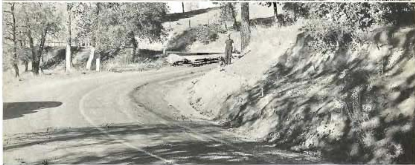
On Placerville project. Upper left—Old alignment between Webber Creek bridge and Clark's Corner. Center left—Webber Creek bridge, to be replaced. Upper right—Realignment across site of new Webber Creek bridge. Lower—One of sharp curves between Clark's Corner and El Dorado to be eliminated. Distance will be shortened almost two miles and short radius curves abolished on this historic highway.
