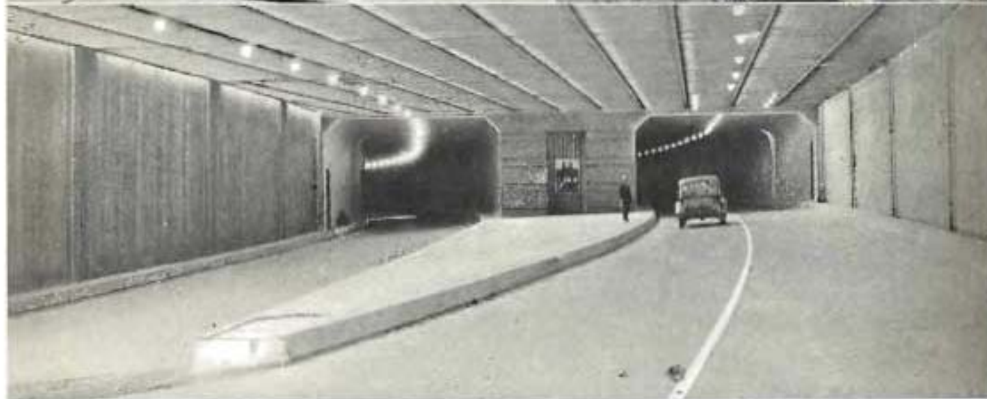
Broadway Low Level Tunnel Project. Upper—Landfills overhead across west approach to tunnel. Center left—West portal of bore. Center right—State highway leading from Moraga Junction to east portal. Lower—Twin tubes of tunnel and lighting system.
