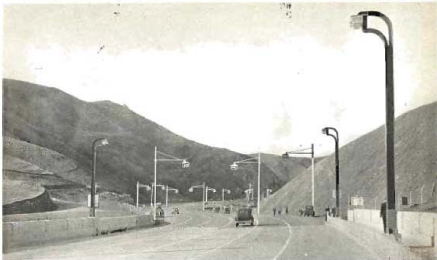
Sketch and photograph shows proposed Waldo Approach lighting system off northern end of Golden Gate Bridge.
