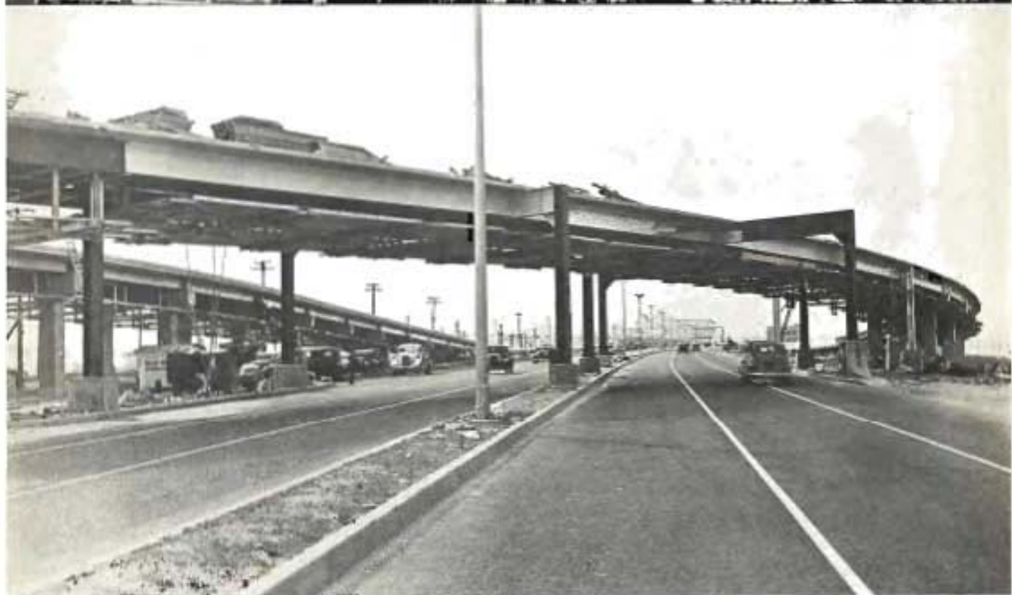
Upper drawing on aerial photo shows East Bay electric railway approaches to Bay Bridge. Key Route trains will proceed through subway. Southern Pacific trains will be routed overhead at end of 26th Street. Lower—Section of Part of Oakland overhead with Bay Bridge and its Toll Plaza in distance. Overhead will connect with bridge highway by ramps as shown in lower picture.
