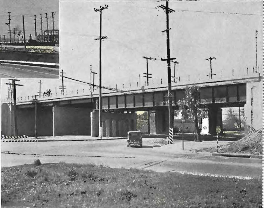
Four grade separations in the Los Angeles Metropolitan area are shown in this group. At top, left, 2600 foot structure across intersection of Mission Road, Huntington Drive and Soto Street where traffic count showed daily movement of 43,000 vehicles and 560 trains. Inset shows old grade crossing. At top, right, structure carrying 600 interurban trains over Firestone Boulevard that shows a daily movement of 20,000 autos. Inset is view of old grade crossing. At bottom, left, structure carrying Santa Fe railroad tracks over four-lane, divided roadway of Atlantic Boulevard. At right, a 2200 foot structure at intersection of Valley Boulevard where through vehicular traffic on Soto Street is carried over both the main line Southern Pacific tracks and Valley Boulevard traffic.
