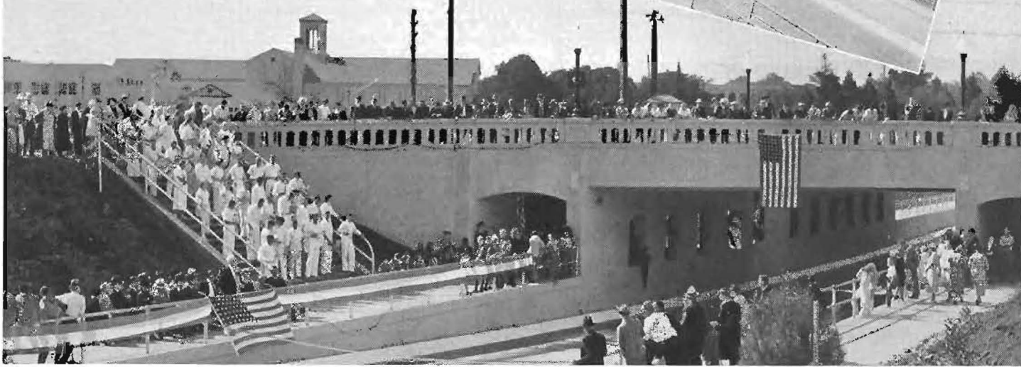
The Embarcadero Underpass at Palo Alto eliminates a dangerous traffic point formed by the intersection of the Southern Pacific main line tracks and the Embarcadero lateral connecting El Camino Real State Highway with the Bayshore Highway—a crossing daily used by a large number of high school pupils and Stanford students and by the large football crowds on game days to and from the adjoining Stadium Station. The underpass carries the Embarcadero roadway beneath the tracks of the railroad and the roadway of Alma Street both of which are accommodated on the structure above. The top picture shows the wide subway for the Embarcadero lateral swinging down to the underpass with pedestrian ramps on either side. Inset is a view of the structure that carries railroad and Alma Street over the subway. At bottom is the scene on dedication day showing the crowd at the speakers' stand and the high school band grouped on the steps.
