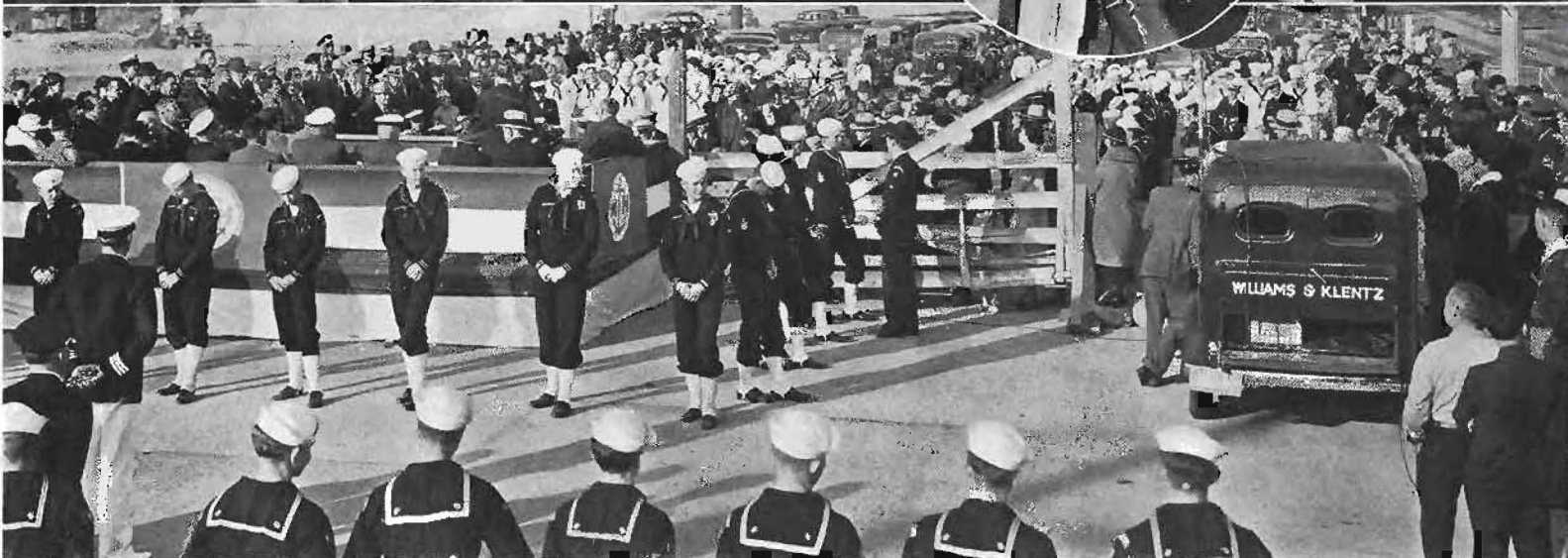
At top, view of Newport overhead, showing east and west ramps and Coast Highway passing under viaduct. Center—Official party at dedication; (left to right) City Engineer R. L. Patterson, Newport; S. V. Cortelyou, District Highway Engineer; Assistant Director of Public Works Justus F. Craemer; Mayor Harry Williamson, Newport; Mrs. Philip A. Stanton, Julien D. Rousael, secretary California Highway Commission; Highway Commissioner Philip A. Stanton; Governor Frank F. Merriam.
