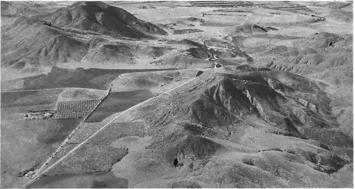
This aerial view taken on the south side of Conejo Summit and looking west toward Oxnard and Ventura shows existing State Highway and realigned route in left foreground, and the realignment down the grade. Photograph taken by Fairchild Aerial Surveys, Inc.
