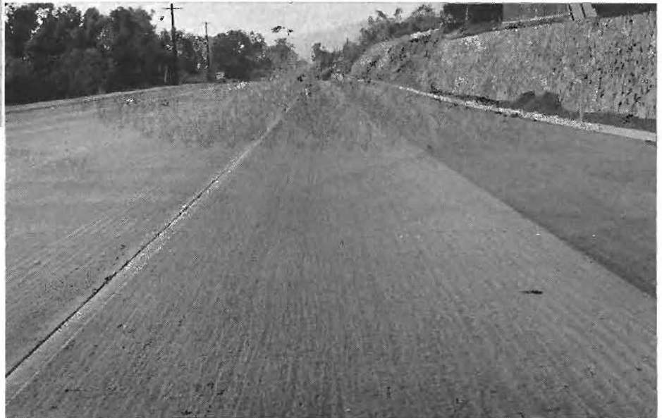
Upper—Close-up view of new type drag finisher being used in road construction by Division of Highways. Upper left—Showing operation of mule-drawn float which reduces cost of highway finishing. Lower—Appearance of highway after use of drag finisher.
