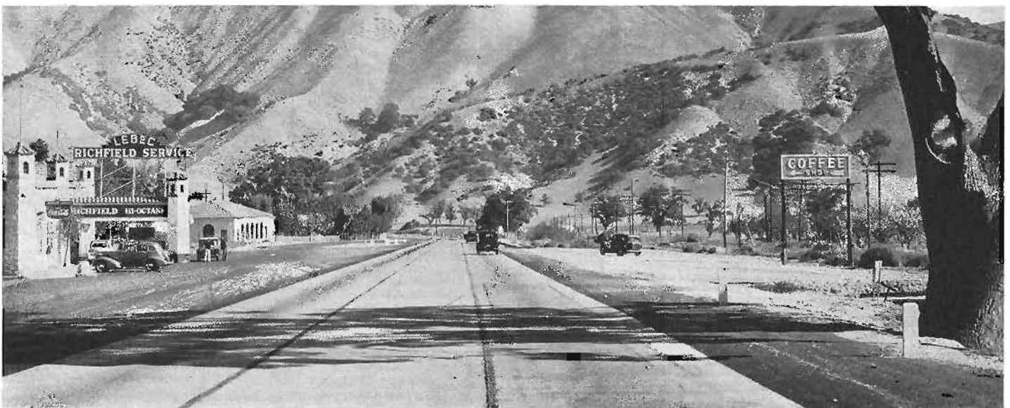
Photograph of portion of 5.5 mile section of 30-foot Portland cement concrete pavement near Fort Tejon in Kern County.
