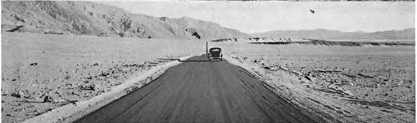
Construction scenes on new highway leading into Death Valley and eliminating Darwin Wash. Drillers at work on difficult stretch with Panamint Sink and Panamint Mountains in distance. Heavy equipment at work on grade which will do away with steep, narrow roadbed over Zinc Hill and Lane Hill. Section of completed desert highway.
