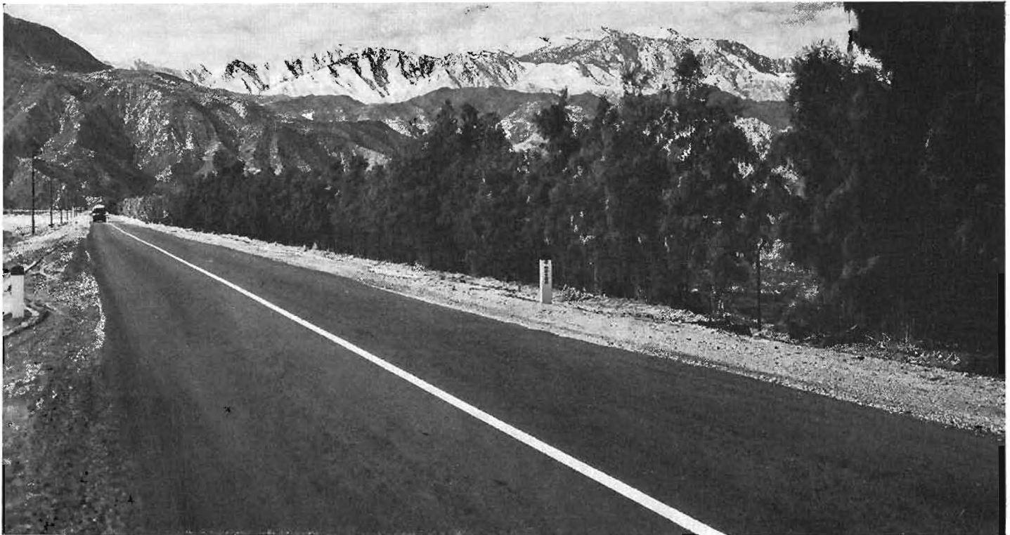
This is a sample of 20-foot road-mix oiled surface on a 10.9 mile section of highway in Riverside County, west of Indio.
