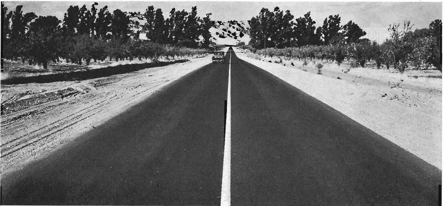
Fine example of 20-foot asphalt pavement laid on a 3.8 mile section of highway near Vacaville in Solano County.
