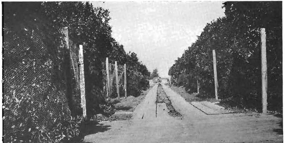
Picture shows how highway engineers built detour through orange grove and protected trees
