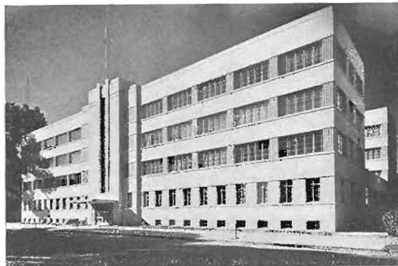
New Public Works Building at Twelfth and N Streets, Sacramento, California
