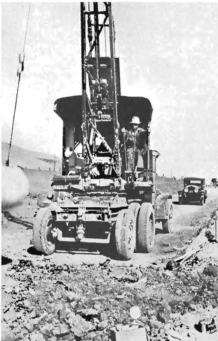
The picture on the left shows portable crane with 2500-pound iron ball attached which is used to break out old highway pavement. Upper right: Iron ball in place on crane truck for transportation. Lower right: Pressure cell on steel plate and concrete blocks placed eight feet below grade to test compaction strength of ball.
