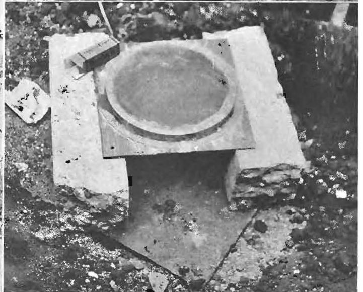
The picture on the left shows portable crane with 2500-pound iron ball attached which is used to break out old highway pavement. Upper right: Iron ball in place on crane truck for transportation. Lower right: Pressure cell on steel plate and concrete blocks placed eight feet below grade to test compaction strength of ball.
