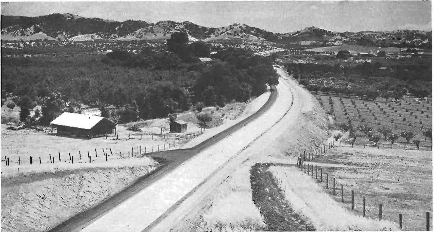
View of stretch of newly completed Vacaville By-Pass constructed to route highway away from schools and congested business district in city of Vacaville.
