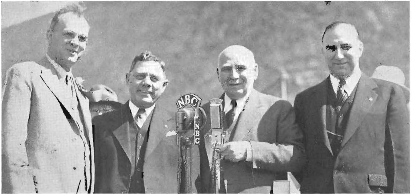
California's Chief Executive formally dedicates Waldo Approach to Golden Gate Bridge, broadcasting his words over a nationwide radio hookup. Left to right: Highway Commissioner Paul Jasper; Harry A. Hopkins, Chairman of Highway Commission; Governor Frank F. Merriam; Director of Public Works Earl Lee Kelly
