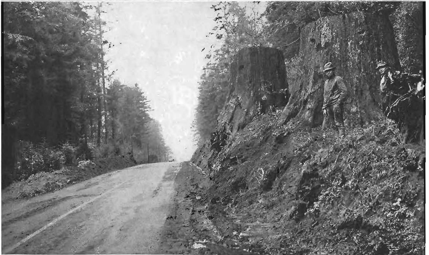
Upper picture is view of section of highway between Trinidad and McNeill's Ranch looking north across Mill Creek showing rolling grade of existing road, which is being realigned. Lower: Redwood stumps which were removed to widen highway.
