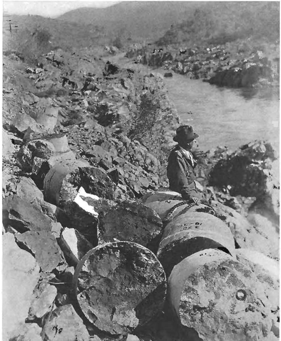
Three foot diameter cores taken out by Calyx drill at Kennett dam site typifying the hard solid rock foundation upon which Kennett dam will be placed.
