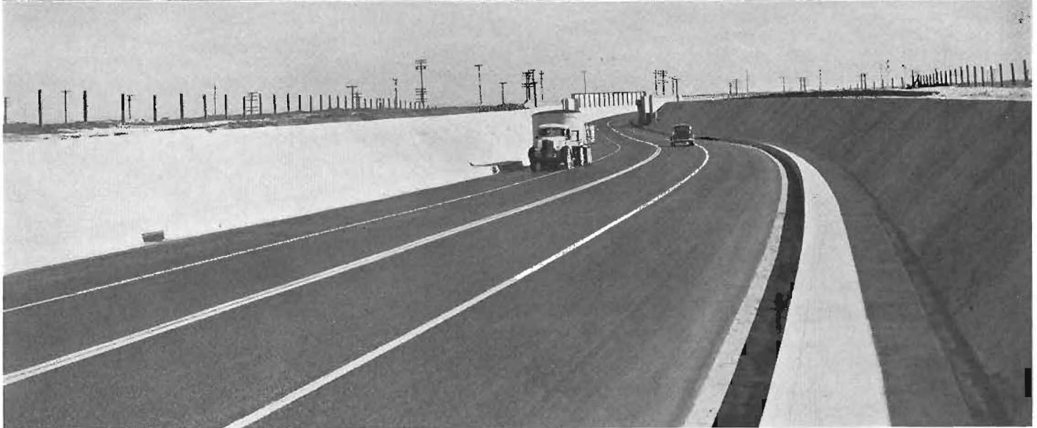
Two views showing close-up and approach to recently completed Famosa grade separation project in Kern County involving a bridge over Poso Creek, a cattle pass, a bridge over Lerdo Canal and subway beneath railroad. Pumps and storage space assure subway will be kept dry.
