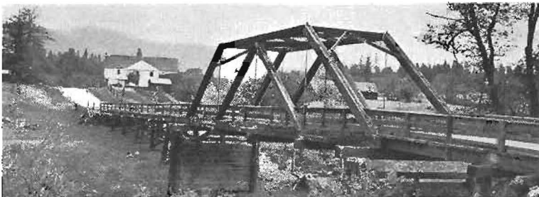
Hayfork Creek bridge, Trinity, is old, narrow and posted.
