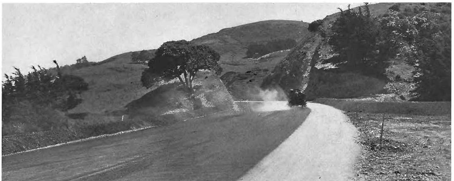
Finishing touches being put on section of new $2,000,000 State Highway leading to Golden Gate Bridge.
