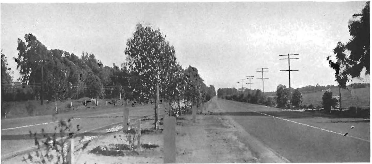
Type of four-lane divided highway used on route through Leucadia in San Diego County showing landscaping of center strip.
