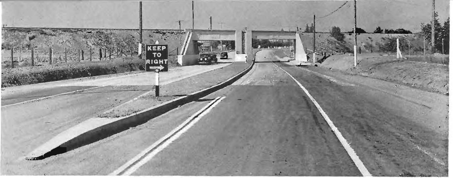
This unit of the Niles grade separation project is the Edenvale Underpass under tracks of Western Pacific Railroad.
