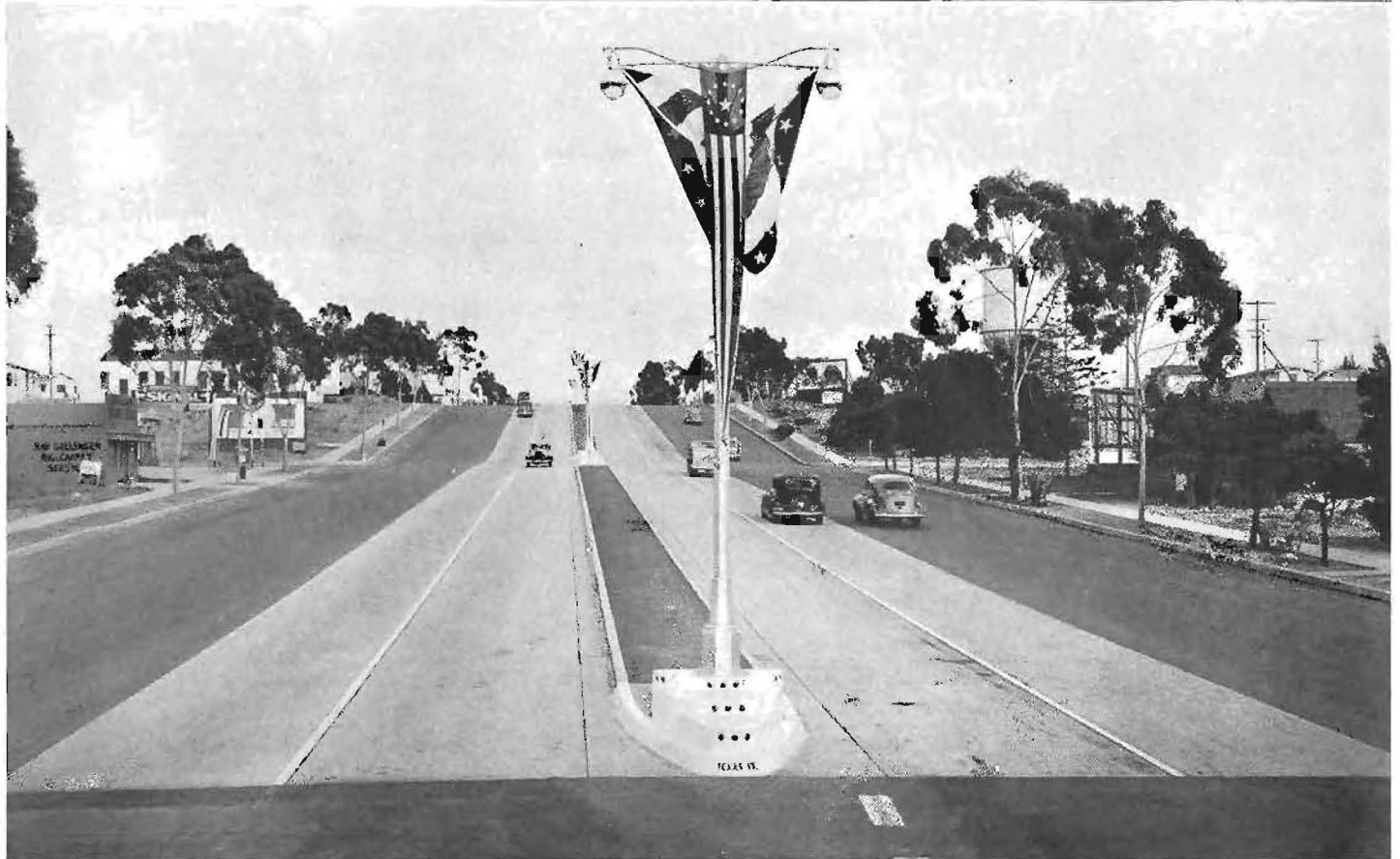
These views of El Cajon Boulevard in San Diego graphically show the width of this new highway and the ornamental divided strip which also affords a safety zone for pedestrians.
