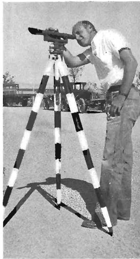
Instrumentman W. C. Names and painted level tripod in use in District IX.
