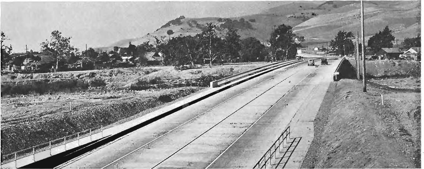
View of four-lane bridge across Alameda Creek, one of units of the Niles improvement undertaking recently completed.
