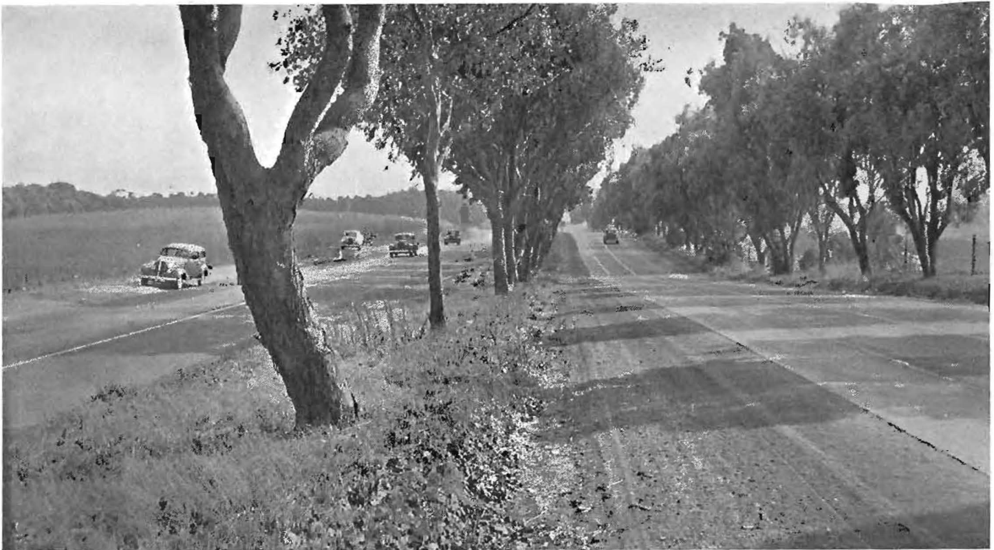
Four-lane divided highway on coast route preserves existing tree rows in the separation strip.
