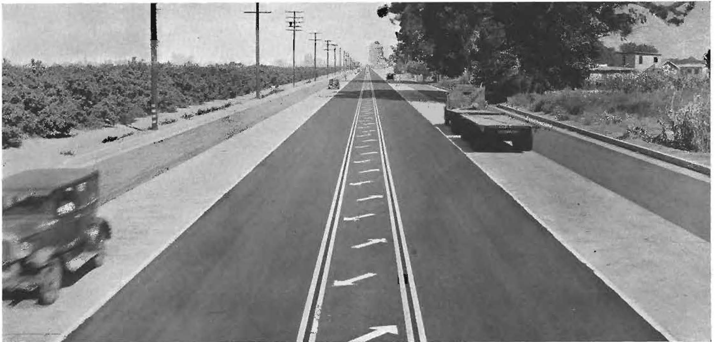
State highway approaching Long Beach; raised white arrows in center dividing strip.
