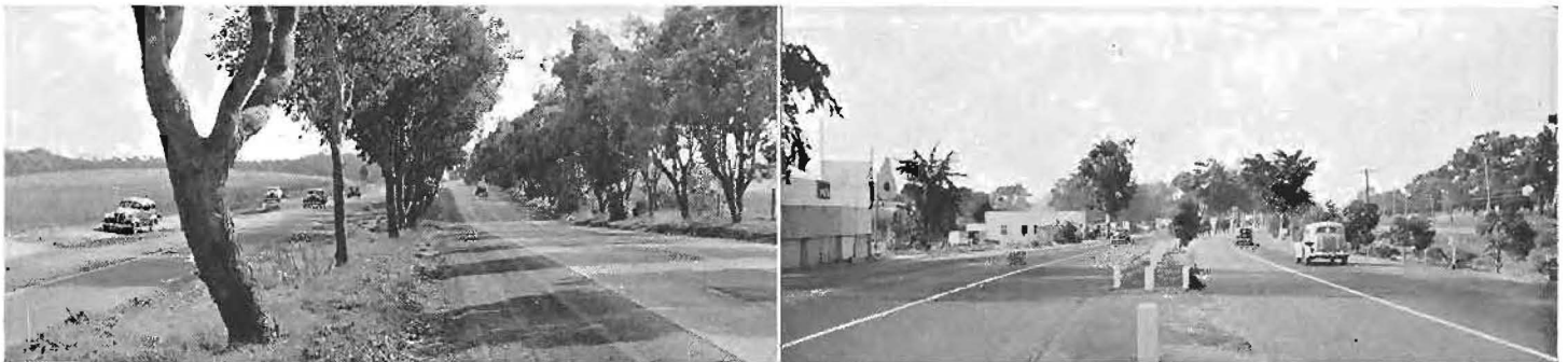
Two views of completed 4-lane divided highway. On left Torrey Pines Mesa section. Right—Stretch through Leucadia.
