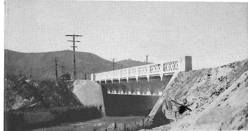
Before and after views of the bridge across Verdugo Creek on State Highway 61 in Los Angeles County. Fed by small tributary streams in the San Gabriel Mountains the creek became a raging torrent that cut a new channel, swept away the bridge approach and damaged the abutment.
