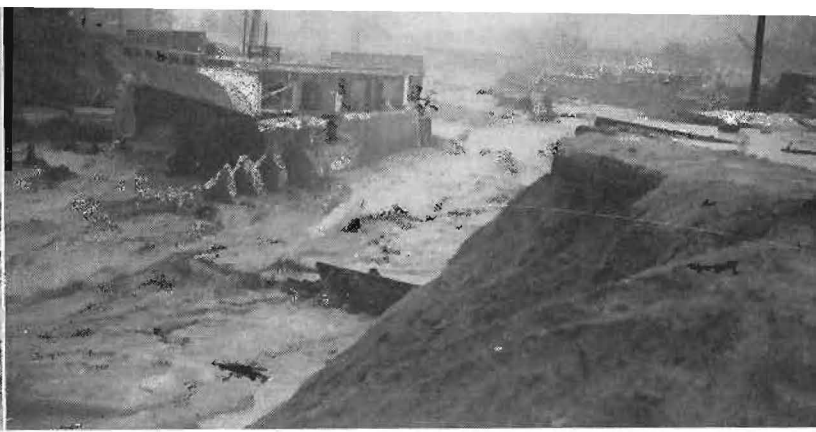
Before and after views of the bridge across Verdugo Creek on State Highway 61 in Los Angeles County. Fed by small tributary streams in the San Gabriel Mountains the creek became a raging torrent that cut a new channel, swept away the bridge approach and damaged the abutment.
