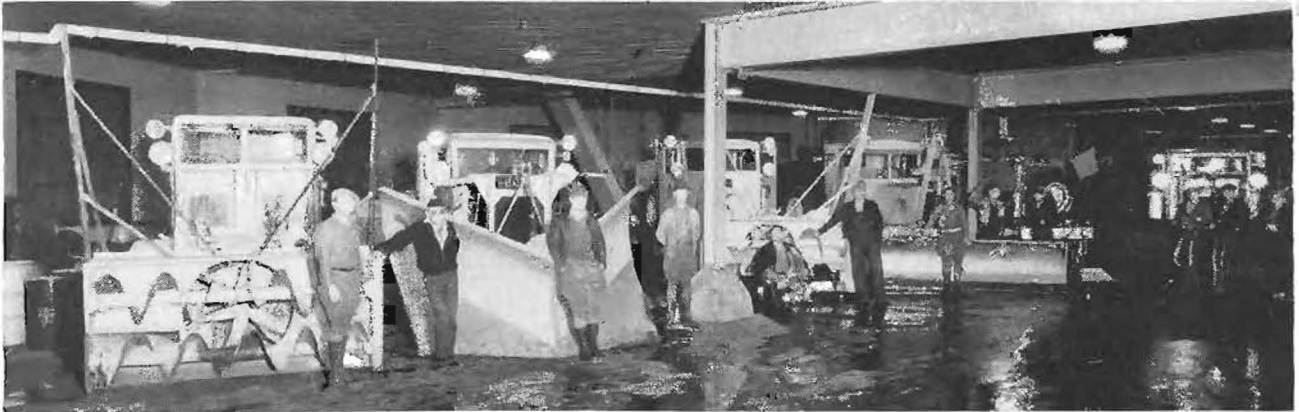
Snow removal crews and equipment. Upper—Maintenance Station Building and crew at Yuba Pass on Donner Summit Highway. Center left and right—Snow plows operating day and night on Donner Summit. Lower—Interior of Donner Summit Maintenance Station showing men and equipment.
