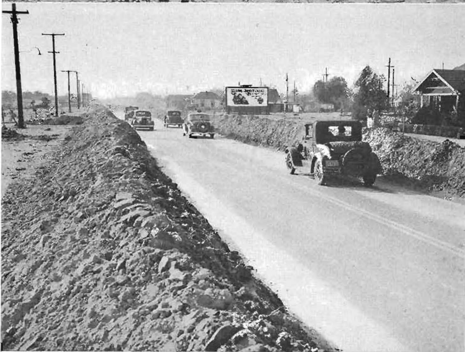
Upper—Huge boulder deposited by flood on Topanga Canyon Road below Wildwood, Los Angeles County. Lower—Mud cleared from highway near east city limits of Colton, San Bernardino County.
