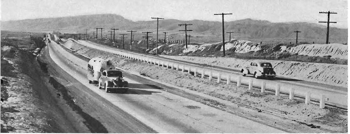
The ample separation strip on the four-lane section of new realignment between San Onofre and Oceanside renders head-on collisions practically impossible.
