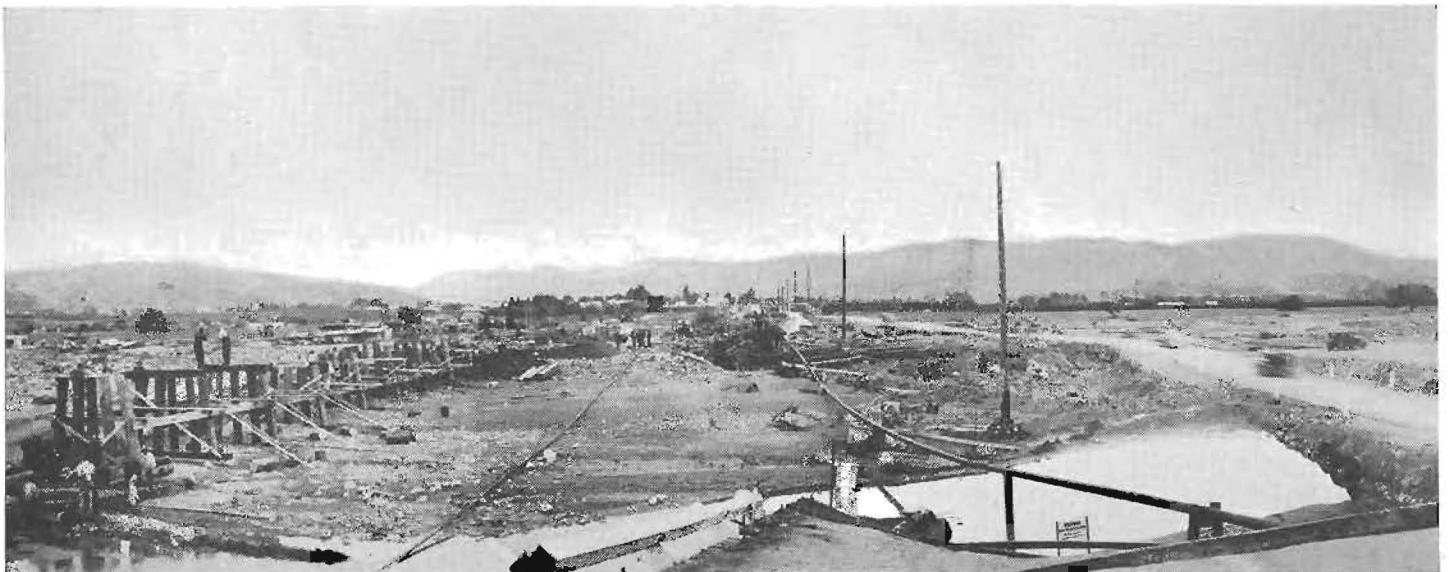
Sespe Creek swollen out of its banks by tributaries in a high mountain area of Ventura County cut a wide swath of damage as it swept across State Highway 79 near Fillmore. A county-built timber and concrete bridge and a paralleling railroad structure were washed away. A large section of highway was obliterated but a detour road shown at right was quickly built and opened.
