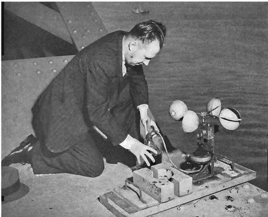
This instrument is an "air analyzer" used on the San Francisco-Oakland Bay Bridge. Carl Hamilton, Maintenance Engineer of the span, demonstrates its use.
