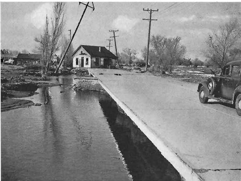
House washed onto highway on E Street near city limits of San Bernardino.
