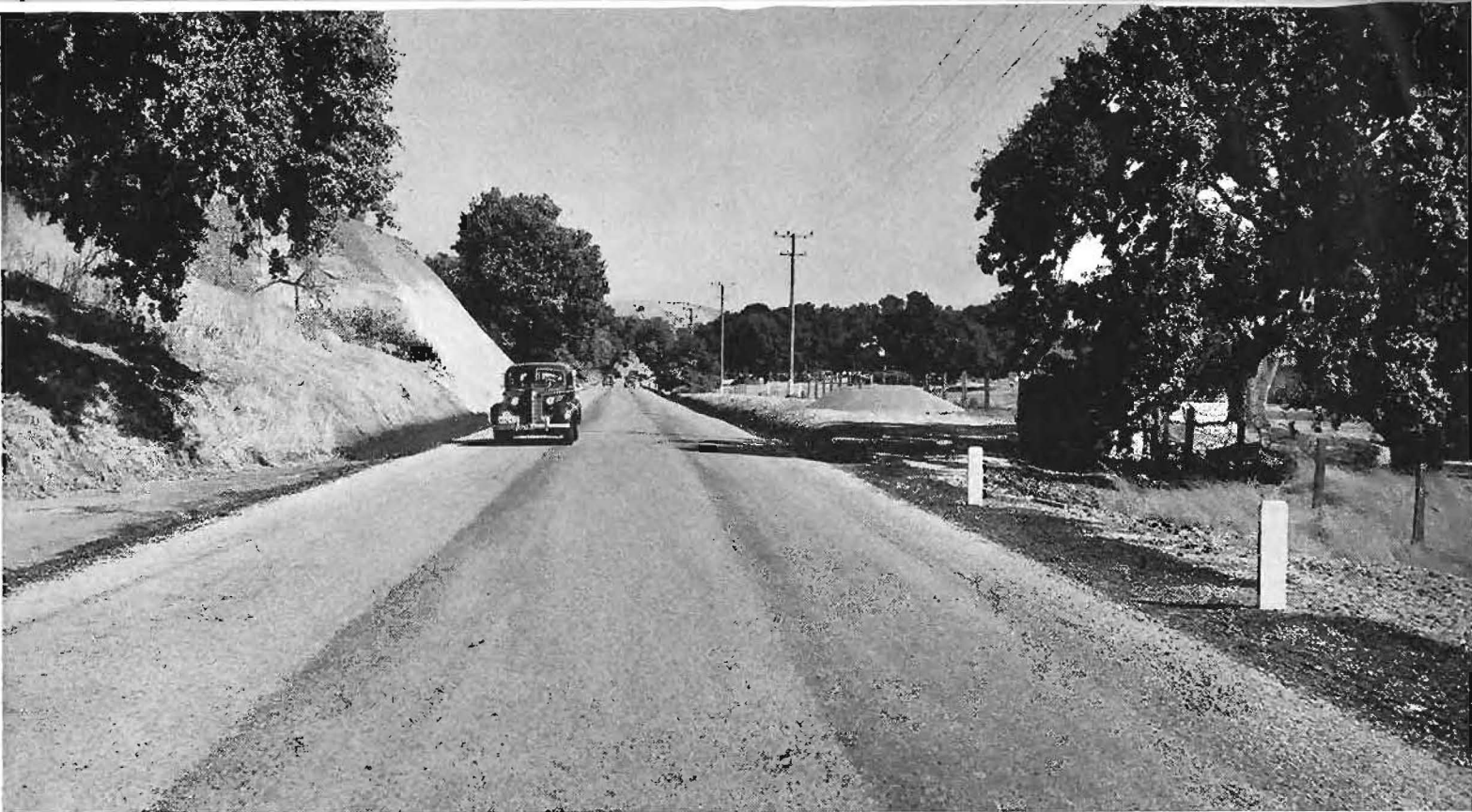
Recently completed section of route to Pinnacles National Monument in San Benito County. Bolado Park on right.
