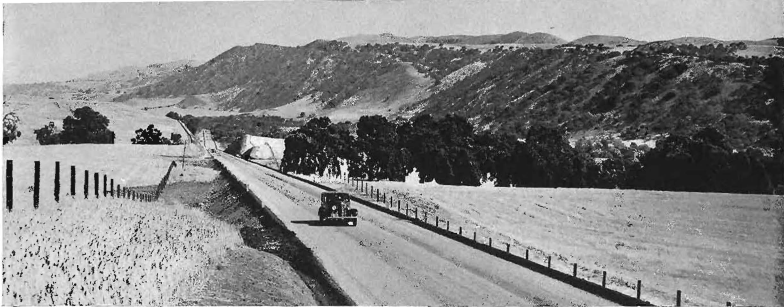
View of another section of new highway between Paicines and Tres Pinos on route to Pinnacles National Monument.
