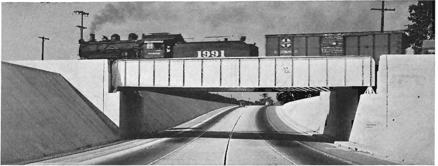
Grade separation on State Sign Route 19 carrying Atchison, Topeka and Santa Fe railroad tracks over highway near Rivera.
