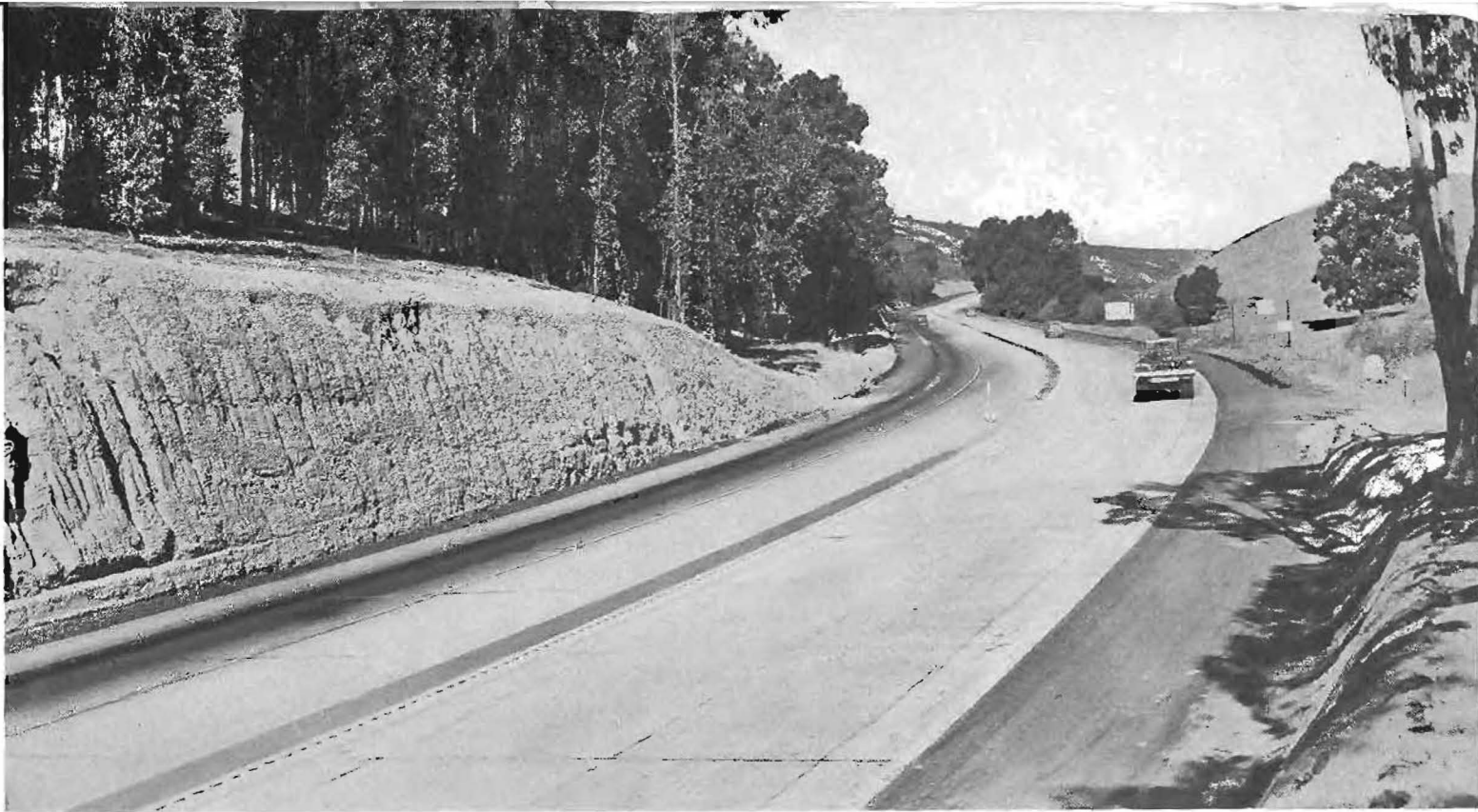
Rose Canyon improvement looking north from Elvira Station showing new divided highway, long easy curves and safety features.
