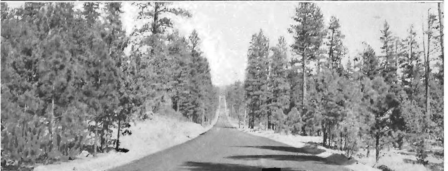
Views of recently completed portions of the Cougar-Macdoel sector of the Weed-Klamath Falls highway, U. S. 97, in Siskiyou County. The top and bottom pictures show long, straight stretches of the 22-foot bituminous mixed surface highway through rolling, partly timbered area. The center picture shows the route looking south across Wild Horse mesa with snow covered top of Mt. Shasta looming in the background.
