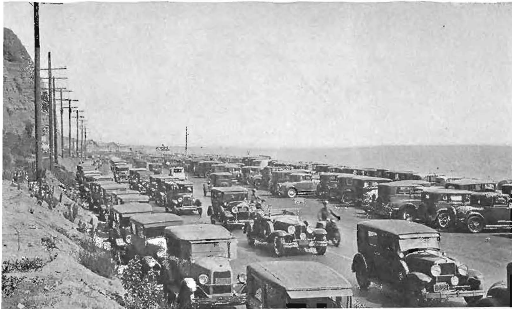
Top—Scene on Coast Route, State Highway 60, north of Santa Monica, which carries a daily average traffic of 10,000 to 15,000 vehicles and more on holidays. Center—Timber truss bridge across Rio Hondo River on State Highway 172, near Montebello oil fields, Los Angeles County. Bottom—Sharp turn at bridge on State Highway 138 between Maricopa and Ojai.
