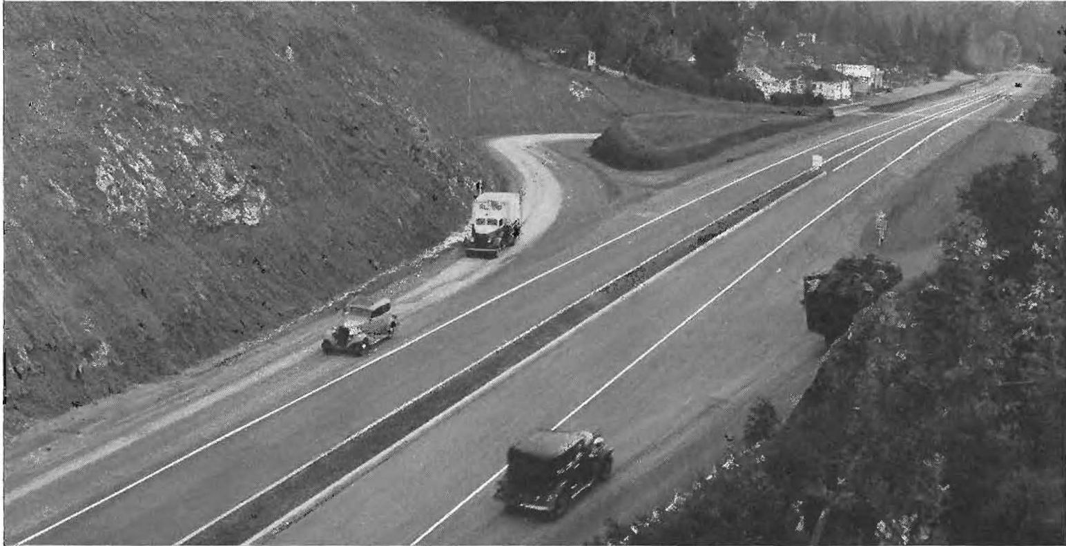
Two views of the realignment of U. S. 101 in Marin County looking from Puerto Suello cut south toward city of San Rafael. Through traffic bound north and south is separated from local traffic by the grade separation in the middle distance and the service roads at the left. Lincoln Avenue is shown on the right of the top picture with local traffic bound north coming through the underpass and up the service road on the left to merge with through traffic. At right of lower picture may be seen a loaded truck entering the truck route on former routing into the city via Lincoln Avenue.
