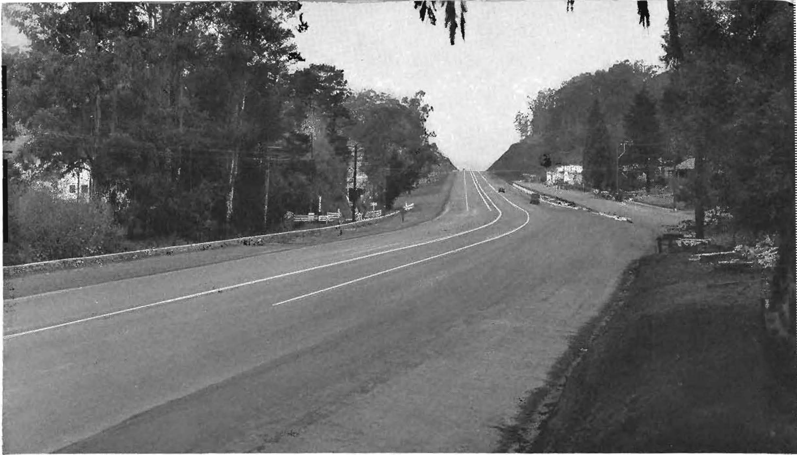
Realignment of U. S. 101 through San Rafael near Grand Avenue has four traffic lanes with painted dividing strip—Service road at right.
