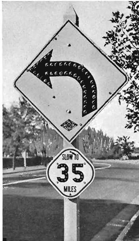
Safe speed signs being placed at curves in test program.
