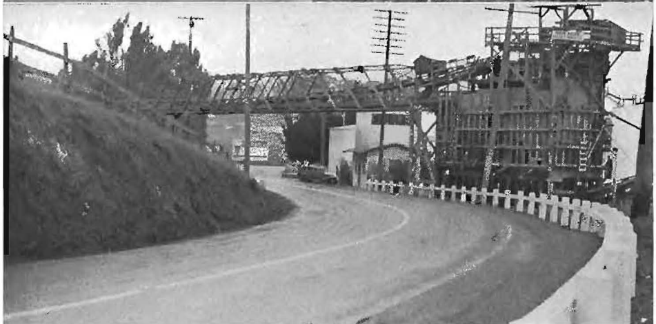
From top to bottom—A danger spot on heavily traveled U. S. 101 near Santa Barbara. Guard rail emphasizes the narrowness of this coast connection in San Mateo County. Another impediment to smooth flow of traffic near Sunol, Alameda County. Alignment such as this is both a bottle-neck and hazard on Redwood highway near Petaluma, Sonoma County.
