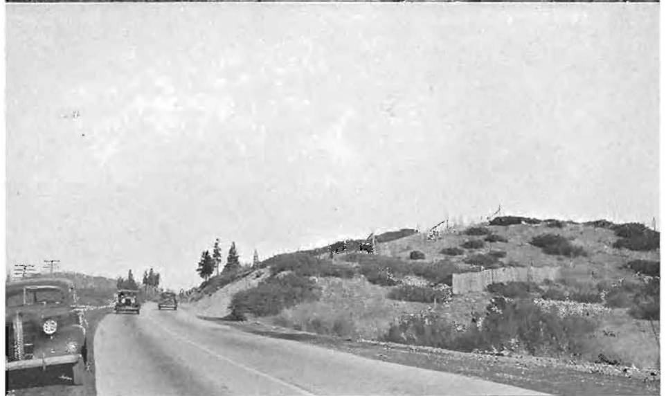
Upper—Trees planted parallel to snow fence will form drift shelter when winds whine down from Mt. Shasta. Center—Trees planted across the front of snow fences on this sidehill. Lower—Wind carried snow up and over this hillside, causing one of heaviest drifts on the road. Six rows of trees are planted up the side of this hill.
