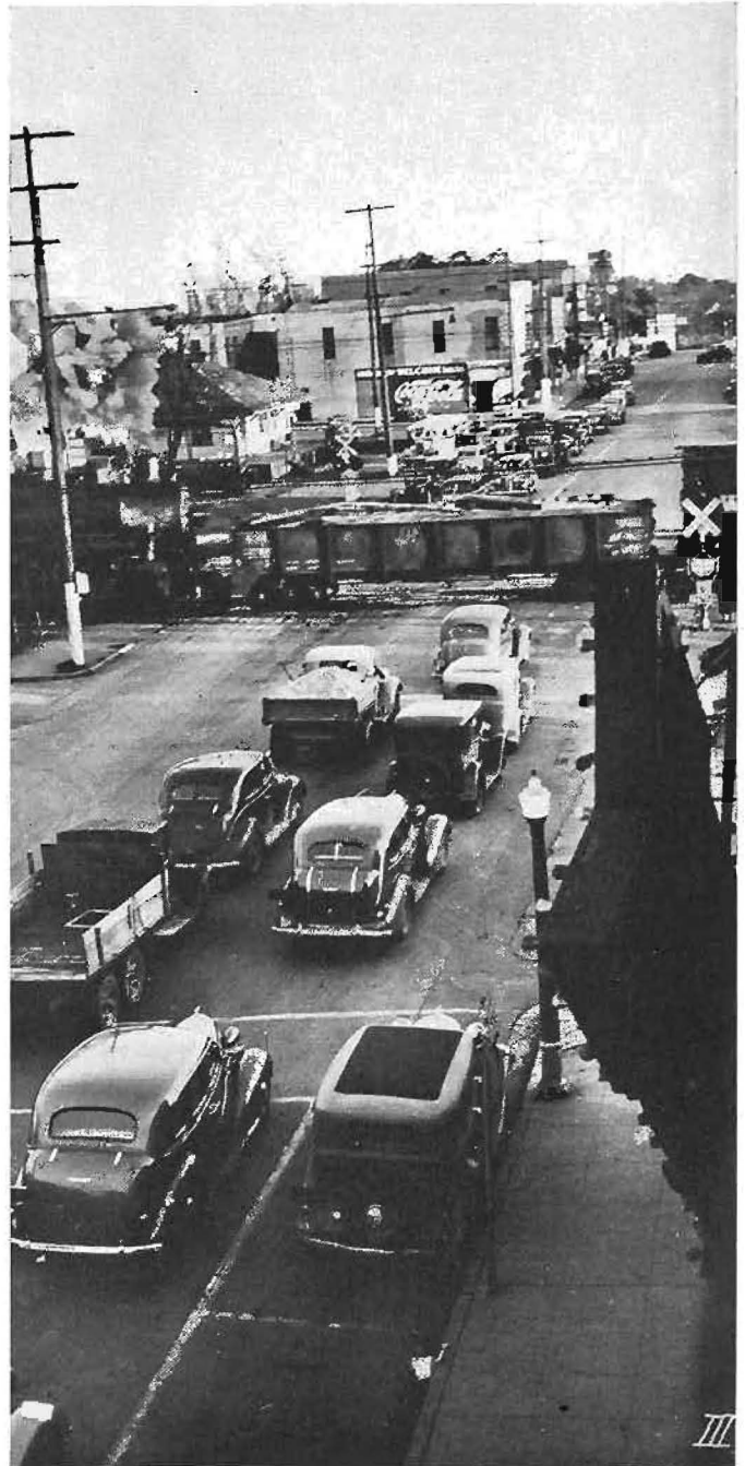
Intersection of U. S. 99E with Southern Pacific Railroad in Roseville. Such traffic blockades as this are frequent.
