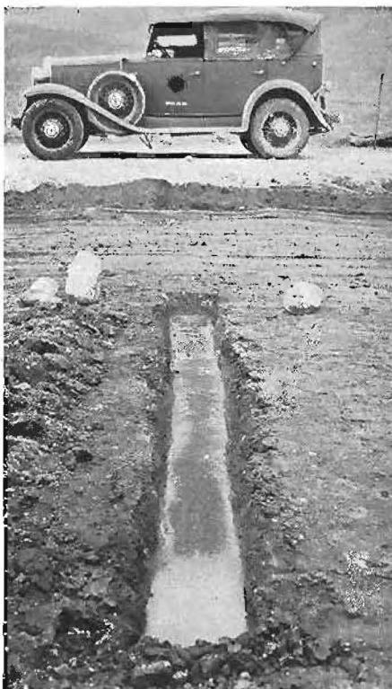
Compacted imported borrow removed to show membrane seal intact.
