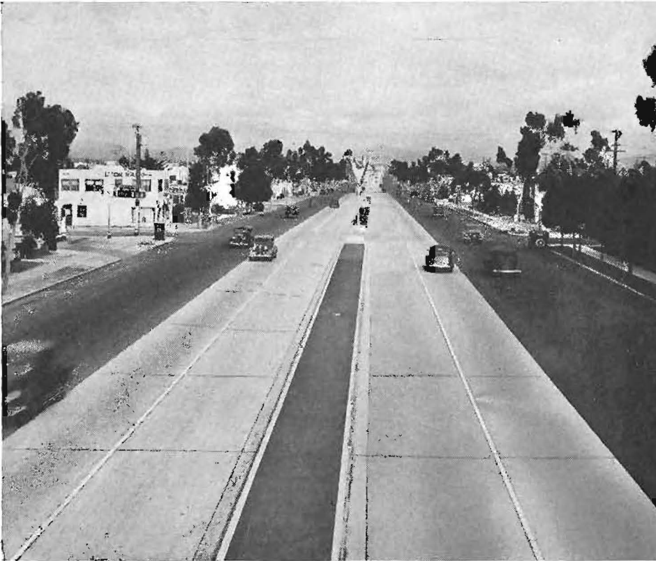
Another highway project completed last year. El Cajon Boulevard in San Diego.
