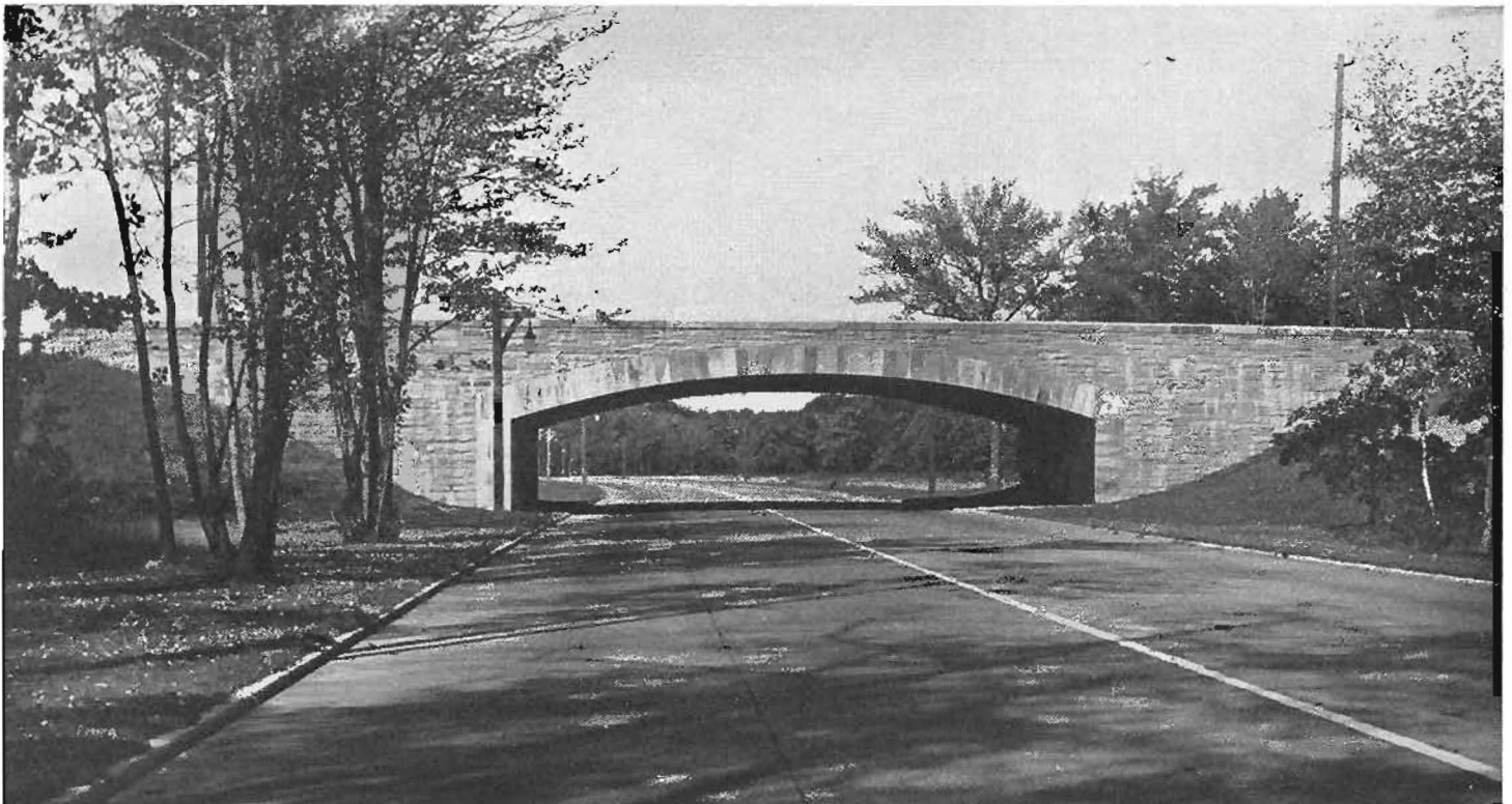
Numerous grade separation structures like the above provide safe traffic movement on the New York Parkway systems in city and suburban areas. The overpass bridges are built of steel and faced with imported cut stone blocks.
