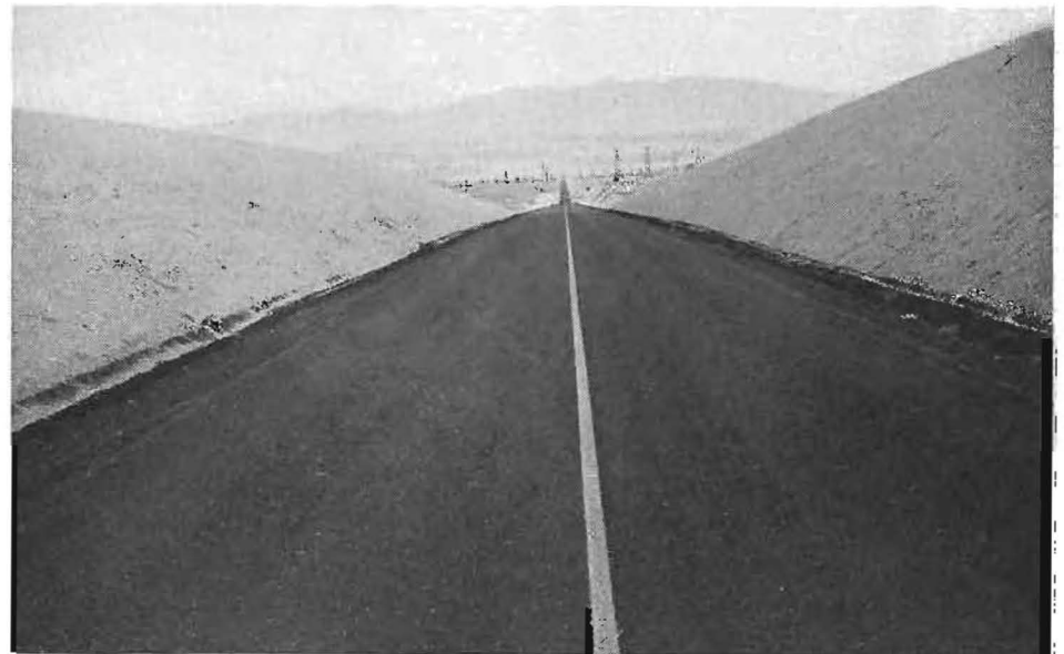
View of recently dedicated Taft-Maricopa Highway looking southerly in direction of Maricopa.
