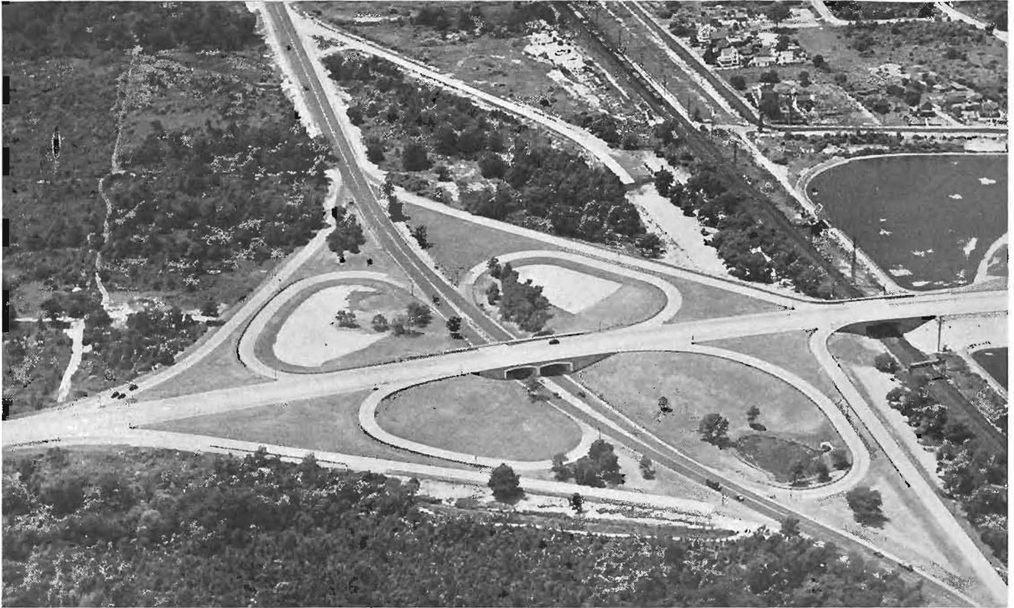
Clover leaf design grade separation typical of many in New Jersey by which vehicles are enabled to make turns at intersections without interfering with through traffic and congestion is eliminated.
