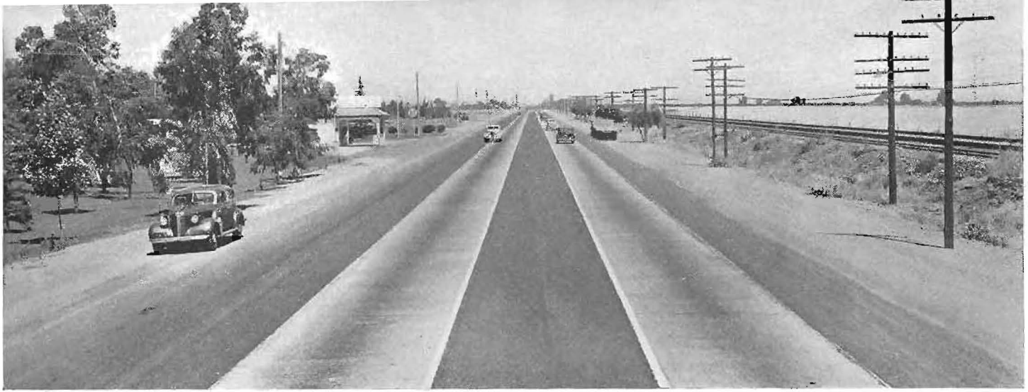
Typical section of new highway between Fresno and Herndon.
