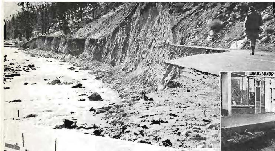
2. Washed-out abutment of Joseph Creek Bridge on Alturas-Lakeview Road, U. S. 395.
