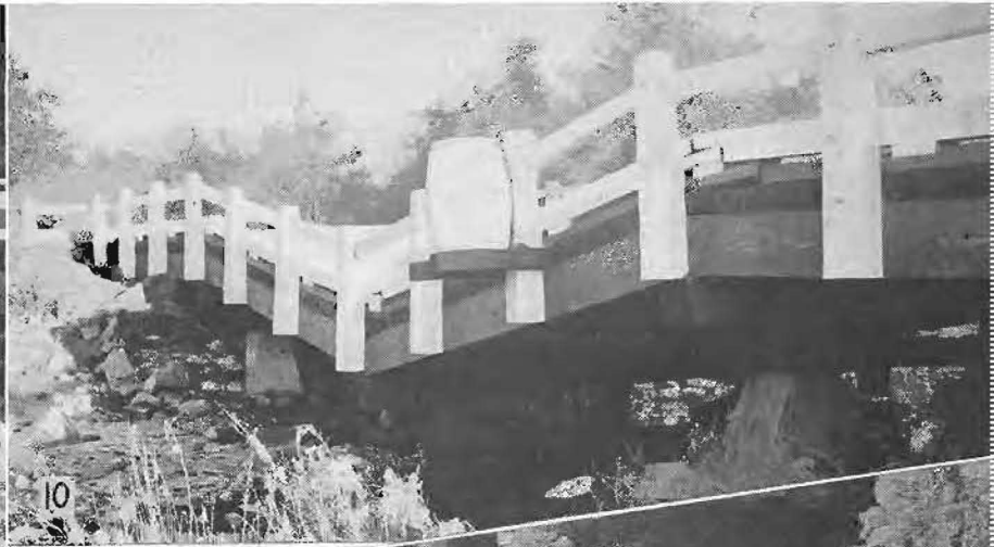
7. Yellow Creek Bridge on Feather River Highway at Belden, State Sign Route 24. 8. Approach fill wash-out at Bear Creek south of Los Molinos, U. S. 99-E. 9. Fill partially washed out along Trinity River west of Junction City, U. S. 299. 10. Undermined bridge near Dales on Red Bluff-Susanville Highway, State Sign Route 36.
