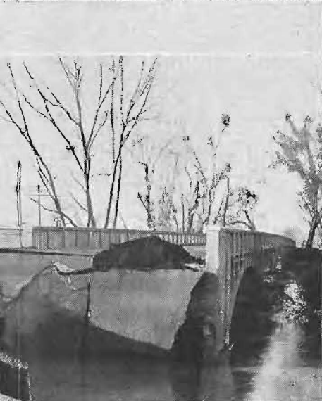
7. Yellow Creek Bridge on Feather River Highway at Belden, State Sign Route 24. 8. Approach fill wash-out at Bear Creek south of Los Molinos, U. S. 99-E. 9. Fill partially washed out along Trinity River west of Junction City, U. S. 299. 10. Undermined bridge near Dales on Red Bluff-Susanville Highway, State Sign Route 36.
