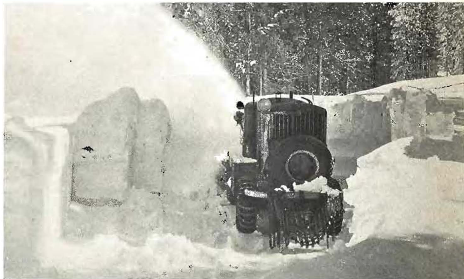
Widening operations to clear highway of deep snow banks.
