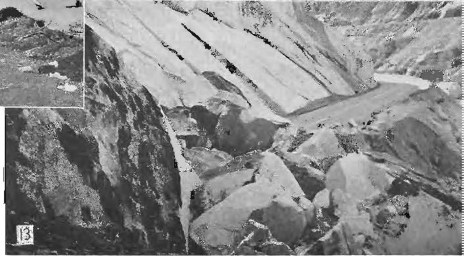
11. Wash-out east of Ingot, U. S. 299. 12. Pavement damaged by flood water east of Hamilton City, State Sign Route 32. 13. Feather River Highway covered by boulders at Butte-Plumas Line.
