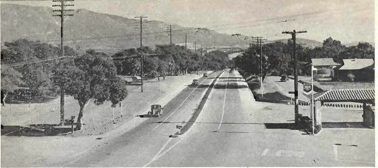
This picture shows westerly end of Montecito project at Olive Mill Road. Local service roads shown on left and right.
