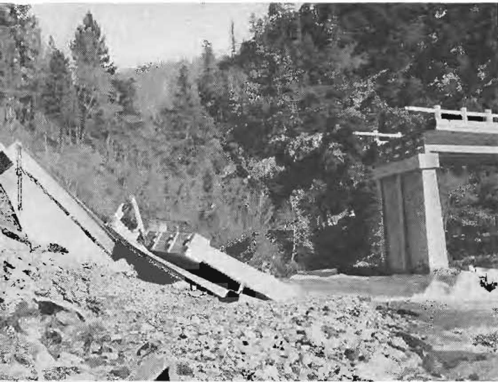
7. Yellow Creek Bridge on Feather River Highway at Belden, State Sign Route 24. 8. Approach fill wash-out at Bear Creek south of Los Molinos, U. S. 99-E. 9. Fill partially washed out along Trinity River west of Junction City, U. S. 299. 10. Undermined bridge near Dales on Red Bluff-Susanville Highway, State Sign Route 36.
