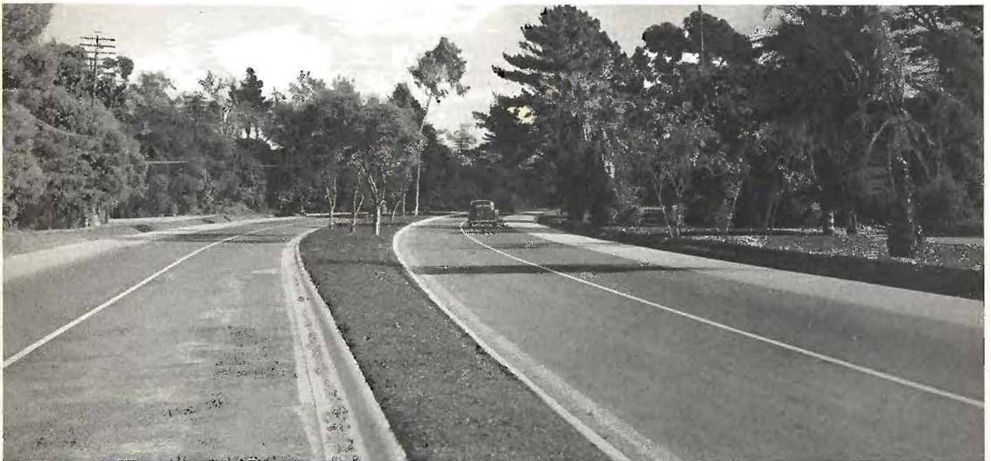
Rolled curb on parting strip is revealed by this photograph. Public utility poles are concealed by trees.
