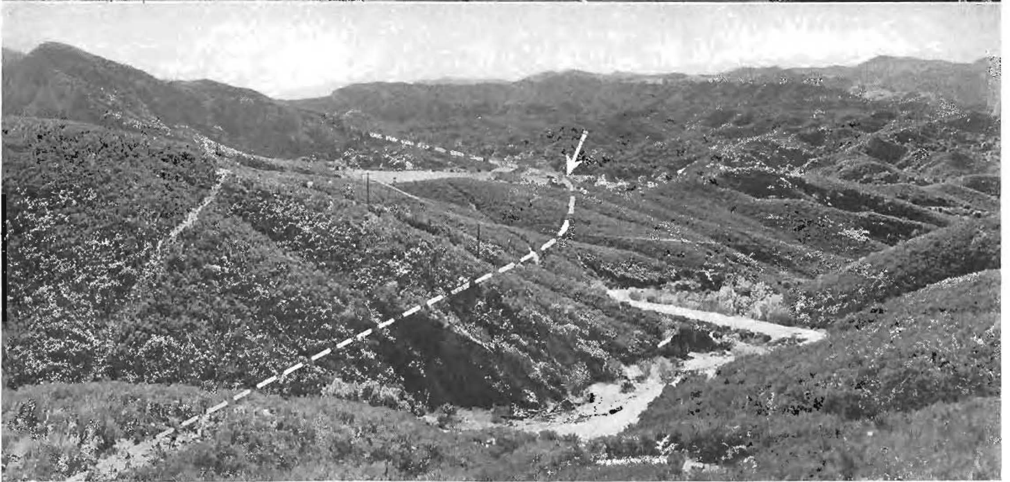
Upper—Newhall Tunnel, narrow bore on Route 23, long has been a serious bottleneck for traffic between the Los Angeles metropolitan area and interior valleys. In construction of the Mint Canyon Cut-off it will be eliminated. Dotted lines on photograph indicate proposed cut slopes to abolish tunnel and provide wide roadway. Lower—Looking south on Mint Canyon short cut route, broken line indicating location of proposed new highway. Arrow shows junction of projected road with present traveled portion of Route 23.
