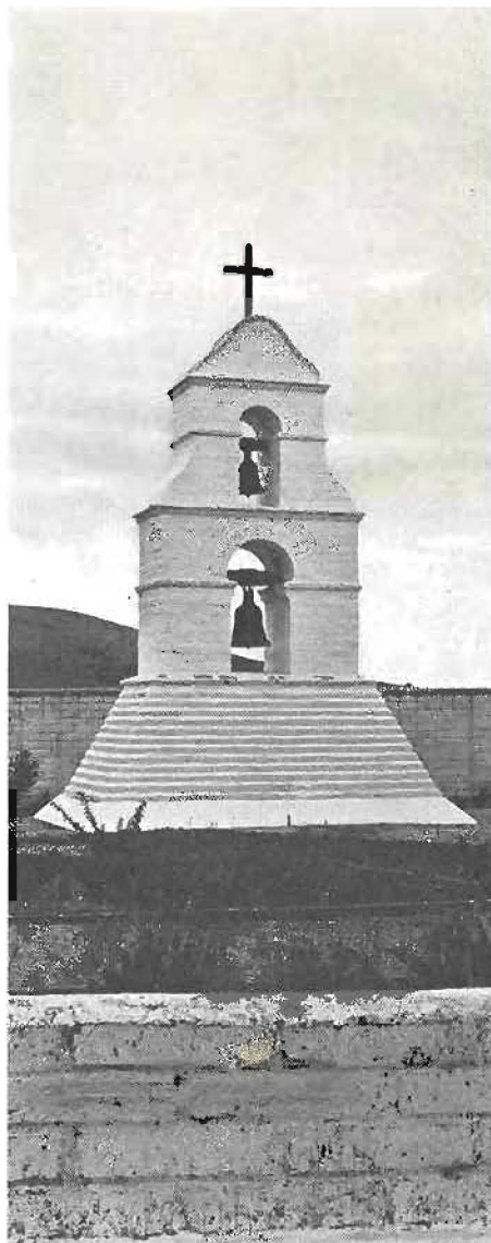
Cross and campanile with its mission bells form motif for Prunedale Cut-off intersection improvement.
