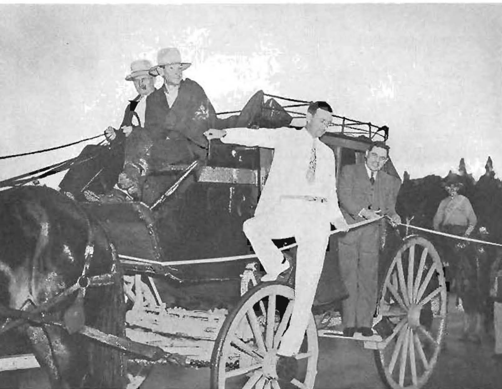
Harry A. Hopkins, Assistant Public Works Director, assisted by Ed Willis, Highway Maintenance Superintendent, snips ribbon barrier on new Placerville Highway as Henry Barton, pioneer stage driver, drives ancient stage coach through it.
