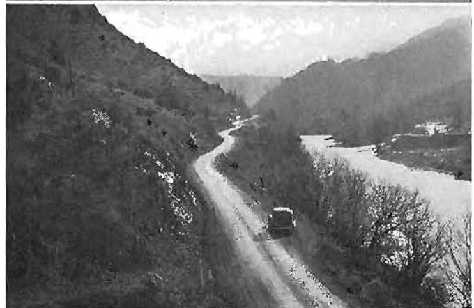
Types of unimproved road in Shasta (top), Plumas (center) and Siskiyou counties in District II.
