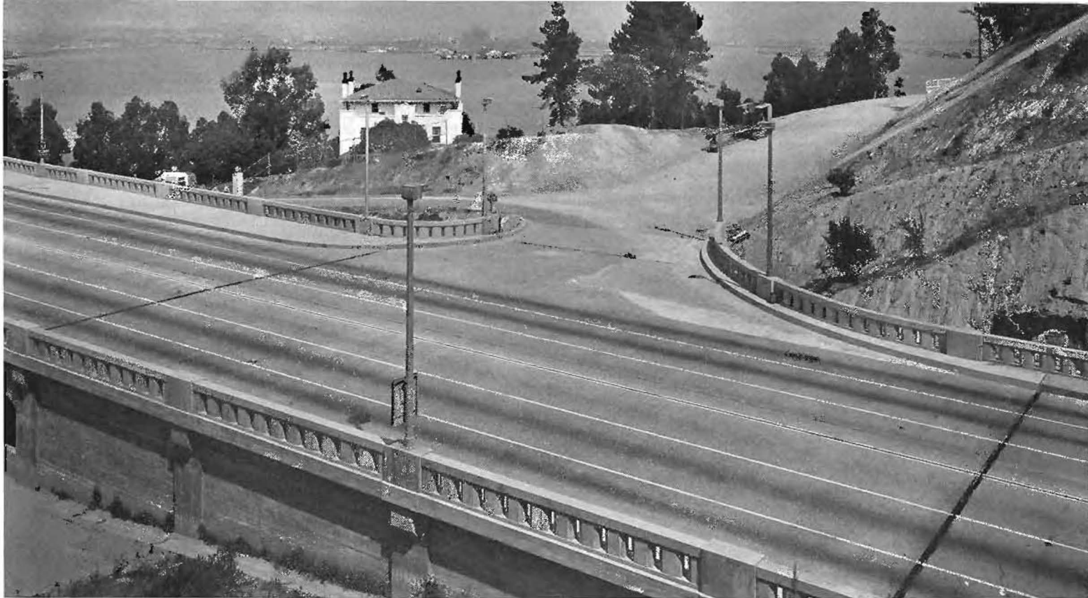
Connection east of Yerba Buena tunnel with World's Fair-Bay Bridge highway. San Francisco motorists having passed through tunnel, will turn right here and circle Island; those leaving Island, bound for East Bay points, will also turn right.
