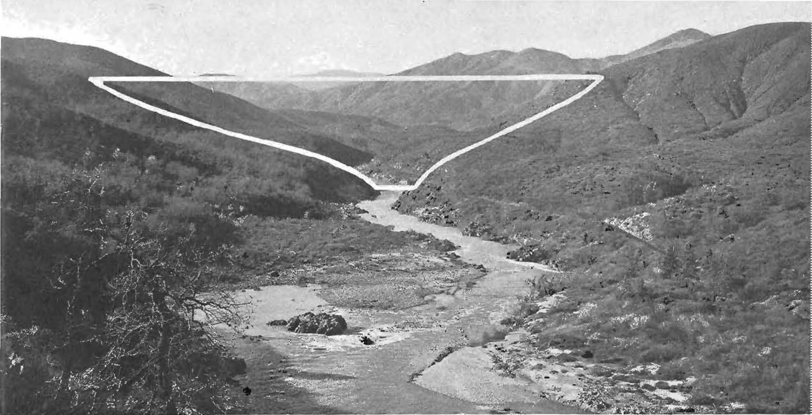
Site of Shasta Dam looking downstream. White line shows approximate outline of dam which will be second largest in world, towering 560 feet, storing 4,500,000 acre feet of water and creating a lake 35 miles long.
