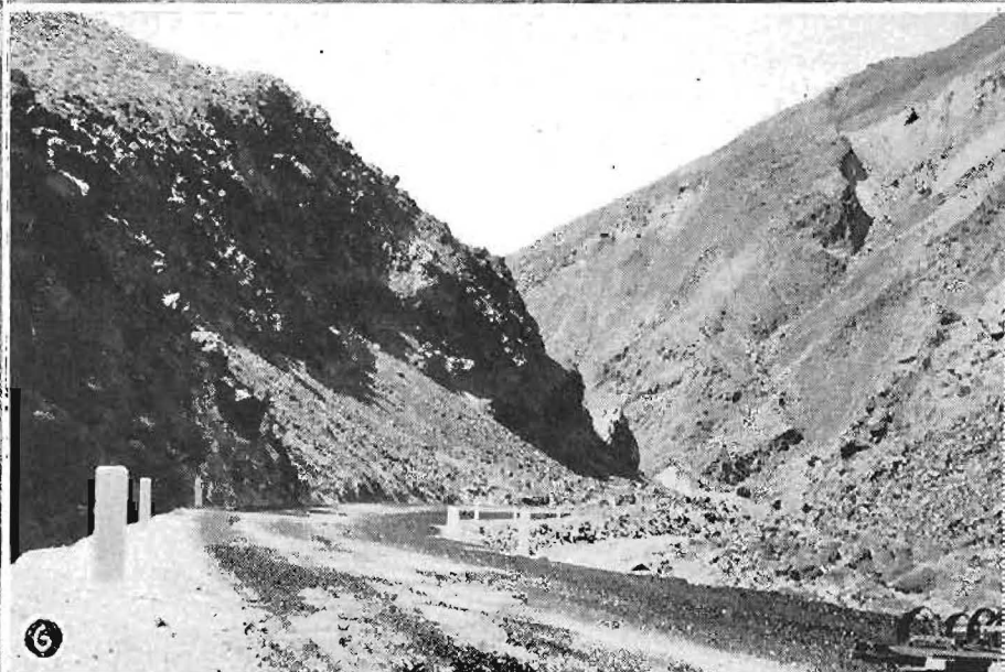
Views of the newly realigned section of Towne's Pass highway entrance to Death Valley National Monument. On the left, views 1, 3 and 5 show conditions before construction that compare with finished highway views 2, 4 and 6 on the right. Drilling and blasting was required through a good portion of the job.
