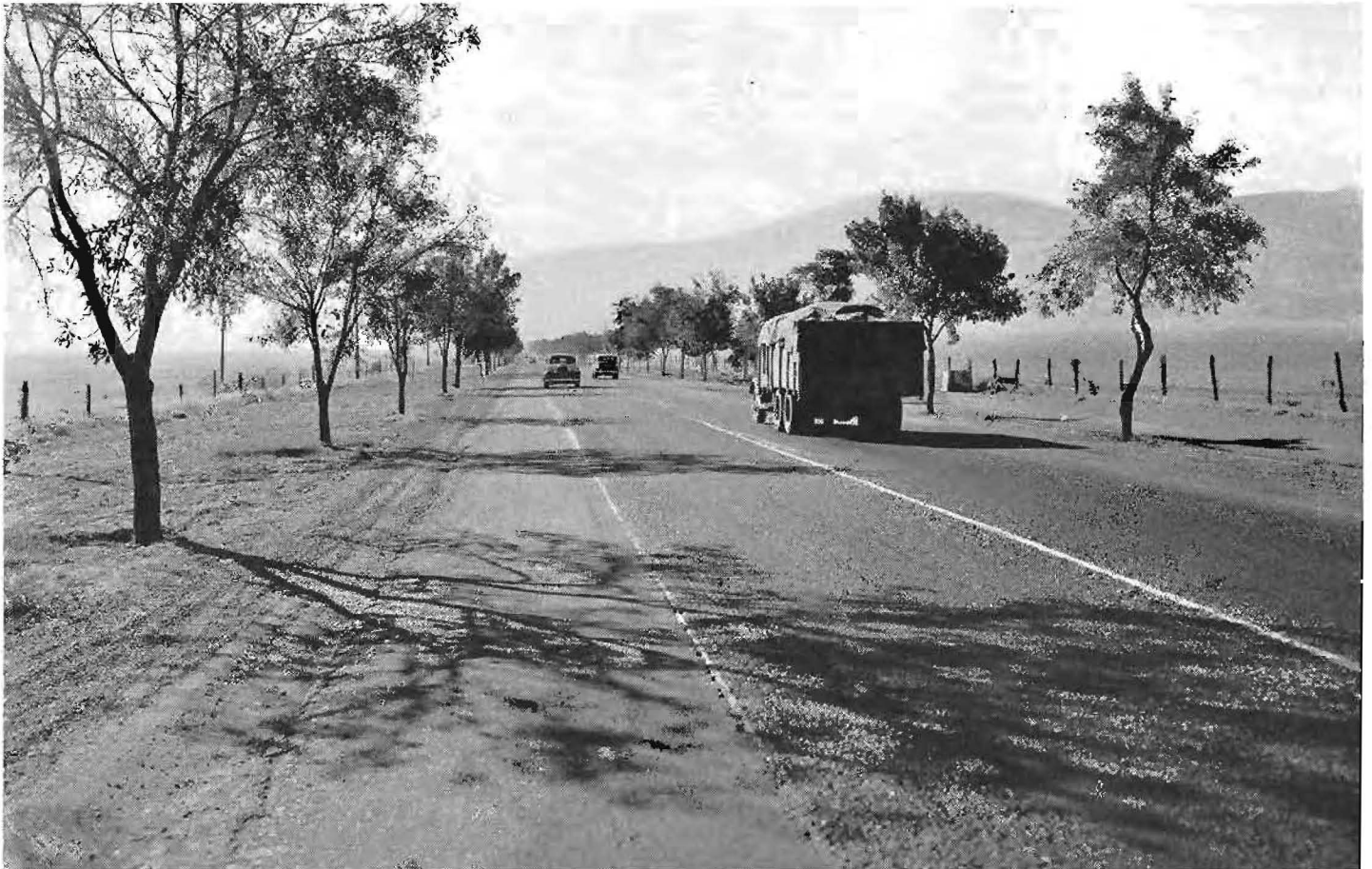
Looking south on Bakersfield-Grapevine Highway showing present road which is being converted into a four-lane divided highway.
