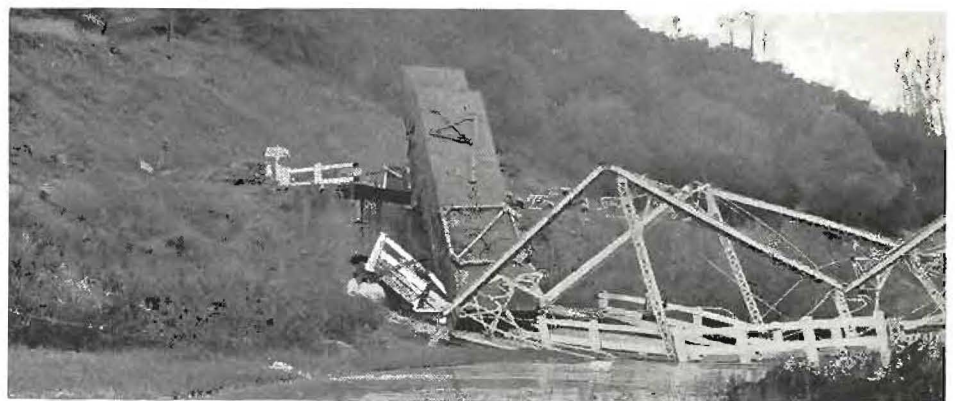
Lower, truss span over Woods Creek on the Oak Flat Road demolished by truck.
