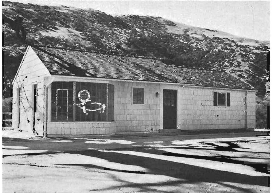
General view of weighing and brake testing station near Fort Tejon in Kern County. Roadway on left protected by guard rail is provided for brake testing runway. Lower—Closeup view of scale house, showing dial clearly visible from outside the house.
