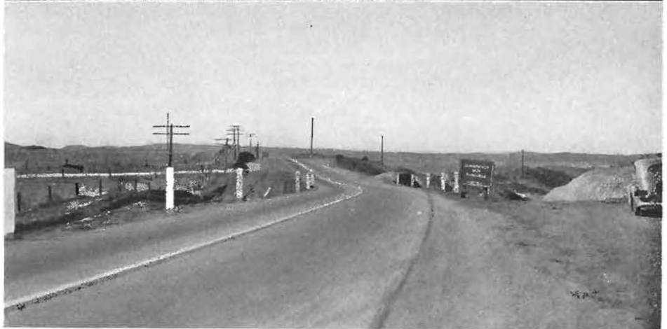
Upper—Construction on stretch of highway between Redlands and Beaumont. Lower—Highway north of Beaumont looking toward Redlands.
