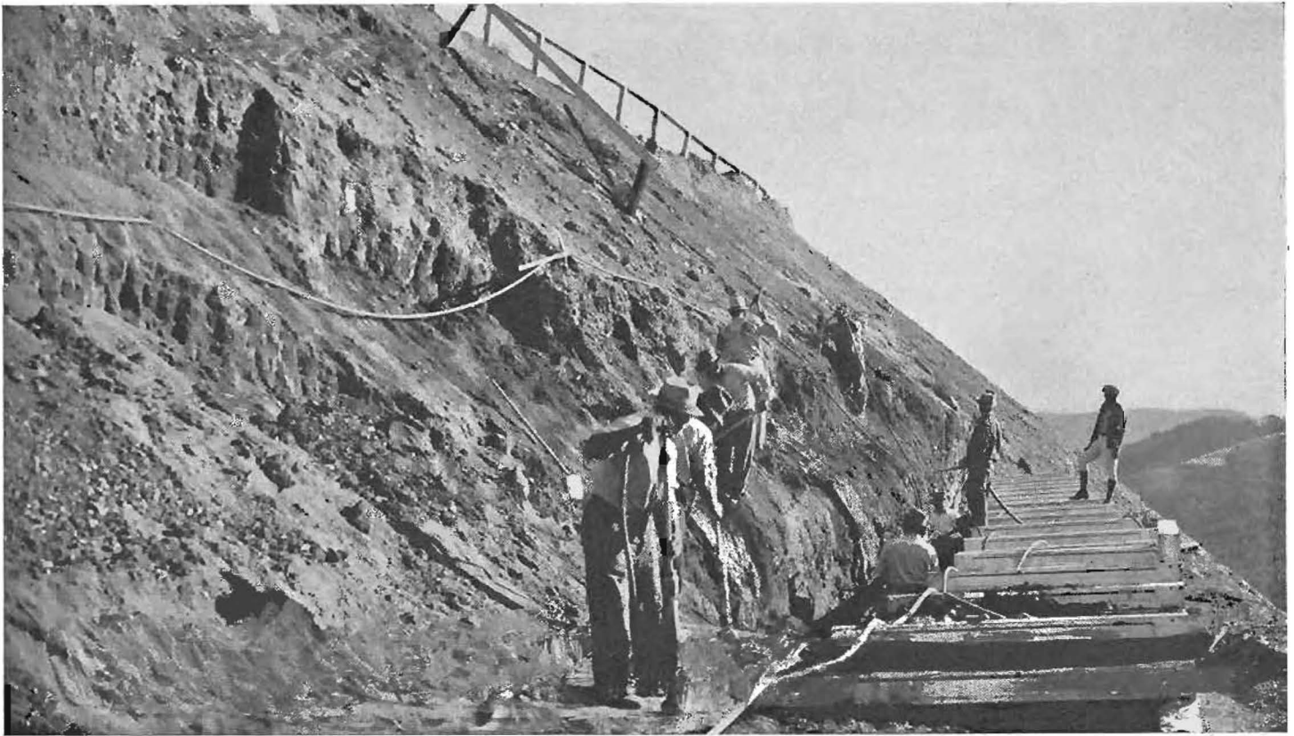
Air spade breaking bank and air tampers backfilling on Cuesta grade.
