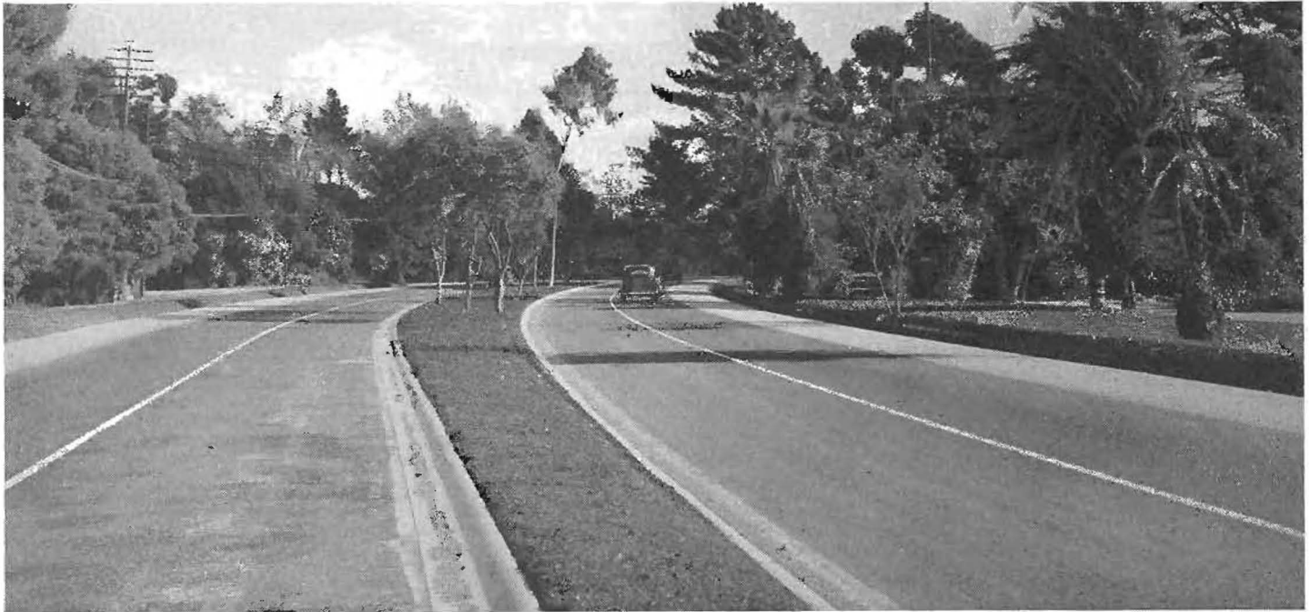
Example of 20-foot asphalt concrete lane with concrete curbs and earth dividing strip in Montecito, Santa Barbara County.
