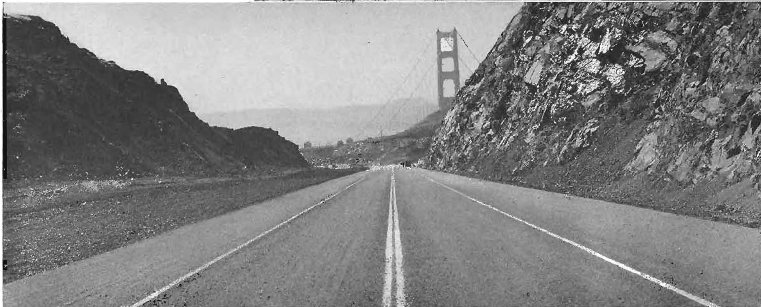
This is 42-foot plant mix surface on Marin County approach to the Golden Gate Bridge.
