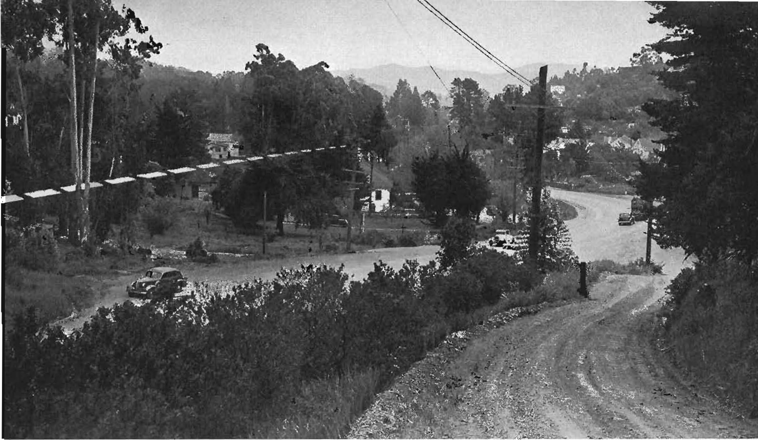
View taken from top of cut through the saddle at Puerto Suello on westerly side of highway looking southward. Section shown in dotted line represents approximately that portion of reconstruction through San Rafael.
