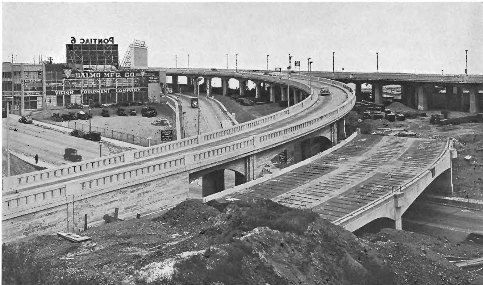
Trains will leave the westerly end of the bridge over a viaduct paralleling the truck and "off" vehicular ramps.
