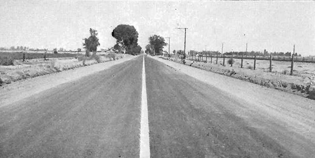
Before and after pictures of secondary highways in Imperial County. These views show sections of the same roads prior to improvement and following regrading and surfacing.
