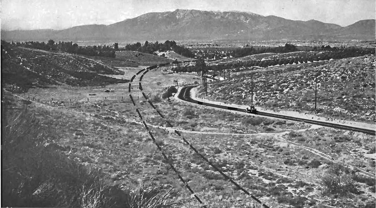
Proposed improvement of East approach to Redlands. Dotted lines show new alignment through valley below Crystal Springs.
