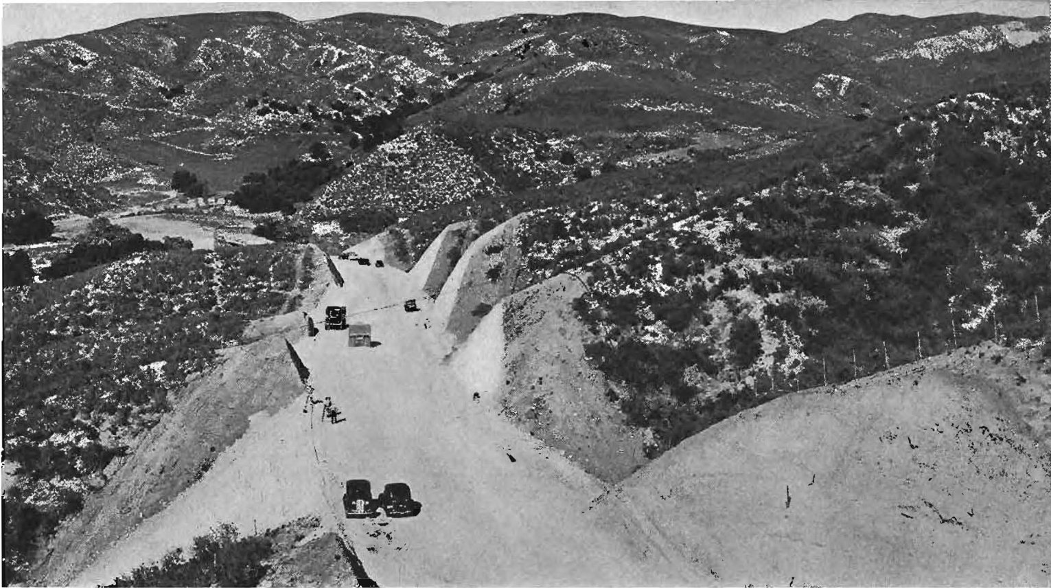
Construction scene on new highway known as Mint Canyon cut-off east of the old Newhall tunnel site. Lower photo shows widening operations eliminating a sharp curve on present approach road to old tunnel site.
