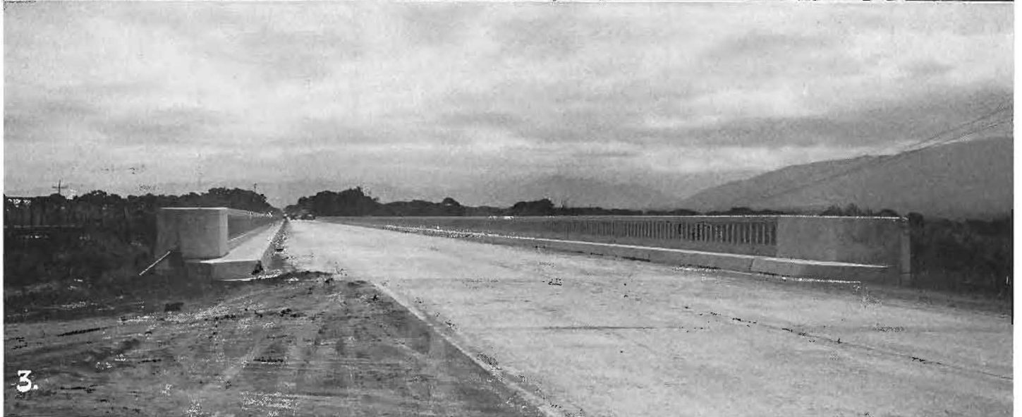
The recently completed bridge across the Salinas River on U. S. 101, near Soledad, is the longest continuous bulb-shaped girder type in the State. It is built on improved alignment near the narrow old structure as shown in the center picture. The overall length is 1530 feet with a roadway width of 34 feet between 2½ foot sidewalks.
