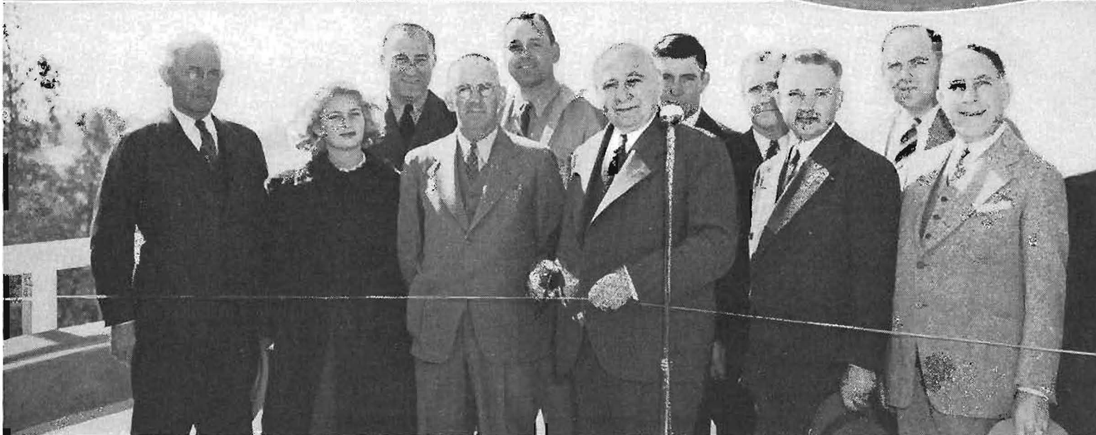
At top, section of new Tahoe-Ukiah lateral realignment. Center—New reinforced concrete bridge across Sutter By-Pass. Upper inset shows flood water conditions. Lower inset shows jumbo moving falsework unit of deck span. At bottom, left to right, State Senator W. P. Rich; Miss Stuart Franklin; Public Works Director Earl Lee Kelly; District Engineer C. H. Whitmore; N. L. Nagler; Governor Merriam; Frank Ettl; Parker Reische; Judge Coates; Maitland Pennington; Dr. W. S. Franklin.
