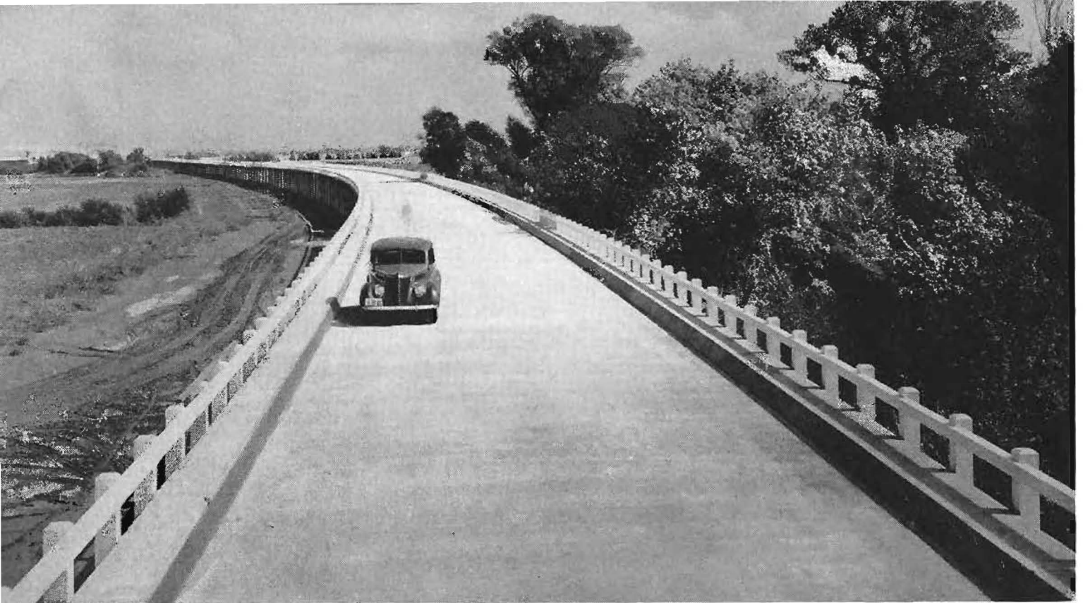
New concrete bridge across Sutter By-Pass on Tahoe-Ukiah Lateral is 4149 feet long and 24 feet wide between curbs.
