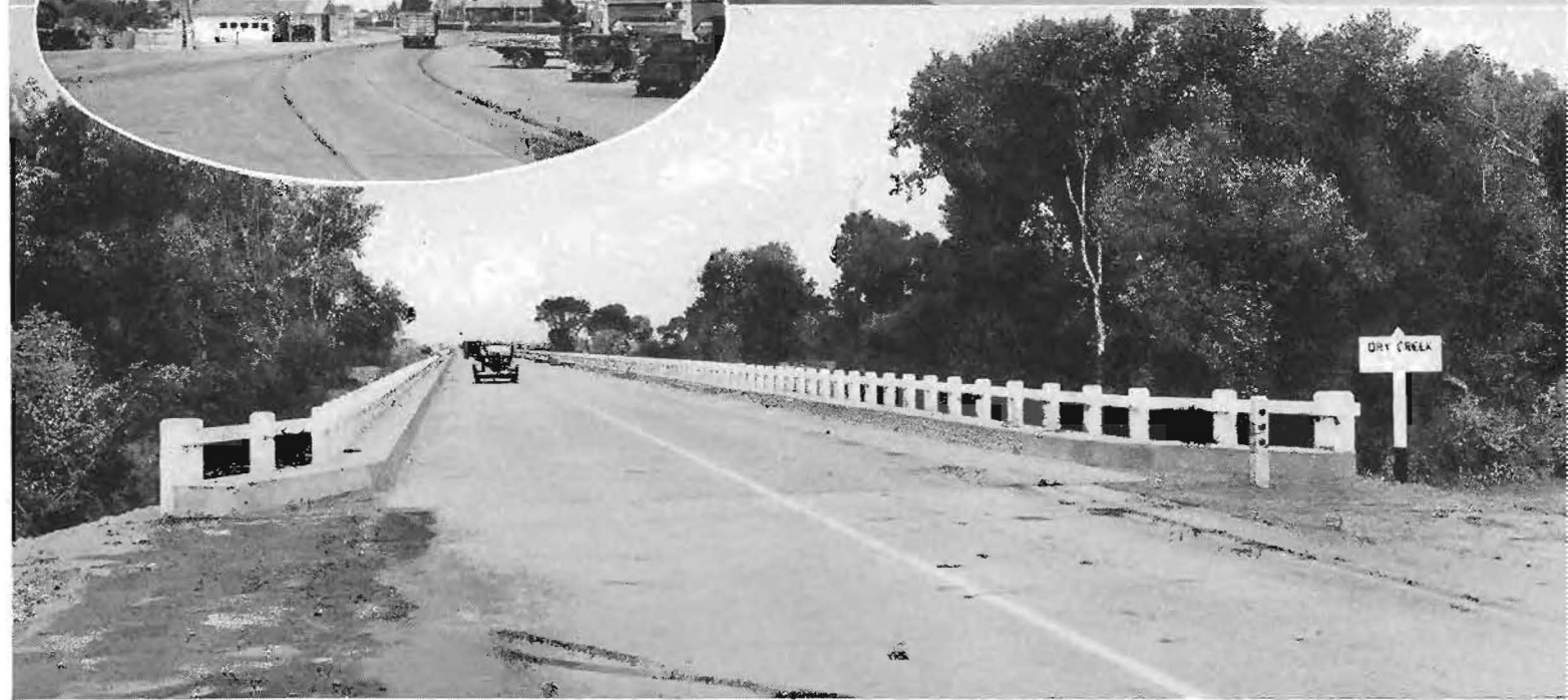
Features of the Galt realignment shown above are: Top and inset—Old, narrow Dry Creek bridge with curved approaches that constituted a traffic bottleneck. Center—Straight new 22-foot pavement with provision for four-lane divided highway. Inset shows old "S" curve through business section past high school. Bottom—New Dry Creek bridge.
