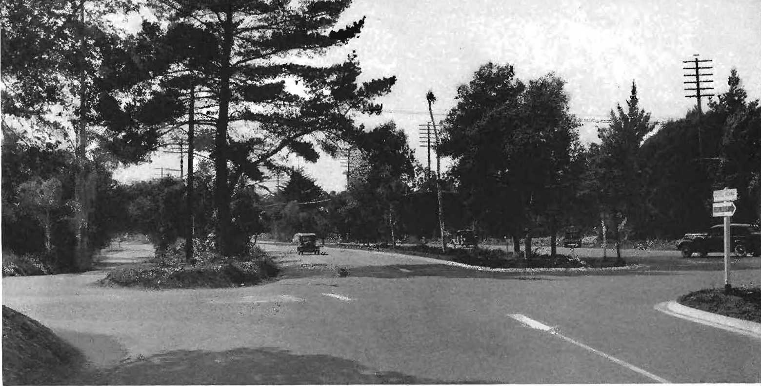
Divided 4-lane highway at Montecito with planted dividing strip and two parallel service roads separated from central roadway.
