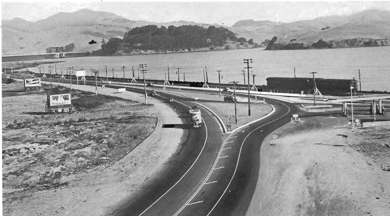
Another view, looking north, of channelized "Y" intersection of Coast Route to Sausalito and Waldo approach to Golden Gate Bridge.
