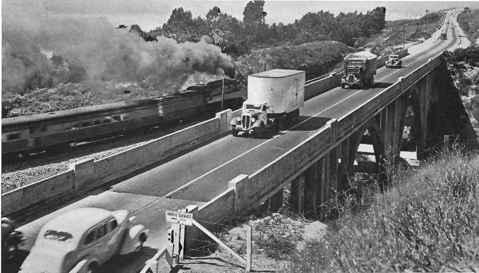
Narrow Bridge on Coast Route in Santa Barbara County that carries heavy truck traffic. Lack of funds prevents reconstruction.
