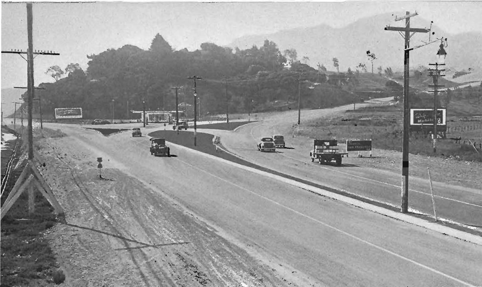
Channelized "Y" type intersection of Waldo approach highway to Golden Gate Bridge and Coast Route to Sausalito in Marin County.
