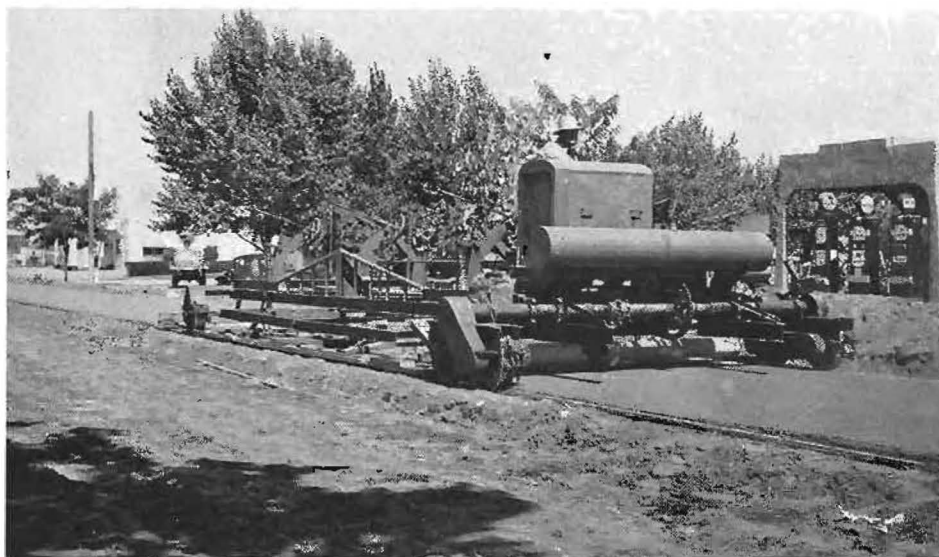
New motorized mechanical float finisher. Front tank holds additional water supply.
