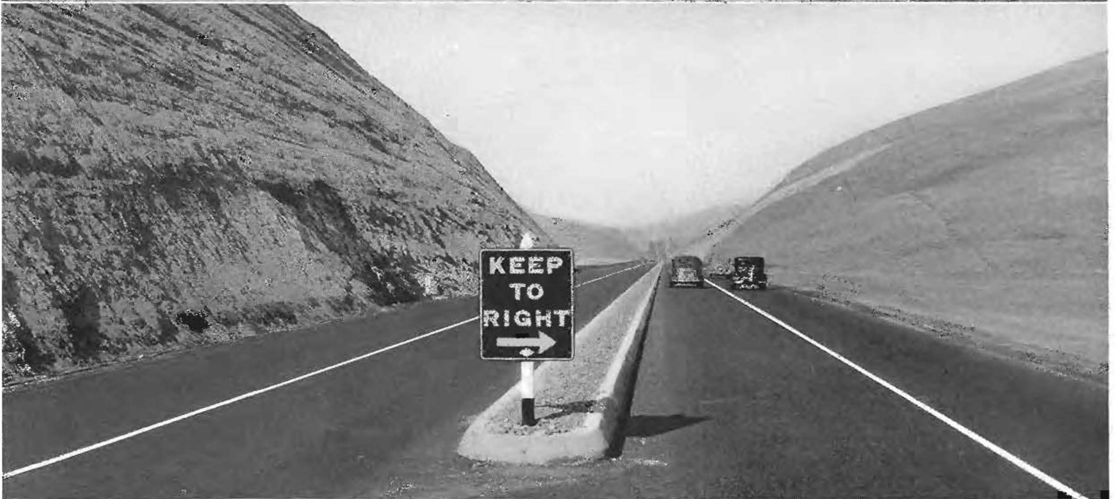
Altamont Realignment features: Top—In foreground overhead structure over Southern Pacific Railroad. Large arched underpass in background carries Western Pacific tracks. Center—Greenville overhead crossing both railroads. Bottom—Close-up of new highway showing raised 4-foot division strip with 6-inch curb and signed opening.
