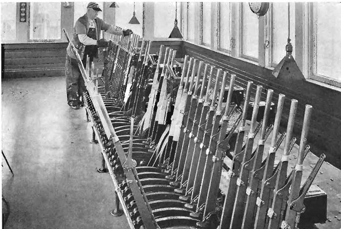
A mechanical lever system would have required 92 levers and 60-foot switch tower.
