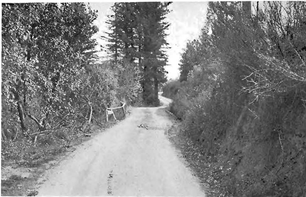
Top—Skyline Boulevard route near Woodwardia in Santa Cruz County. Original narrow county road maintained by State. Center—Blind intersection with Southern Pacific grade crossing with blind approach to Western Pacific underpass in background, near Sunol, Alameda County. Bottom—Blind curves on Russian River highway, between Gurneville and Monte Rio, Sonoma County.
