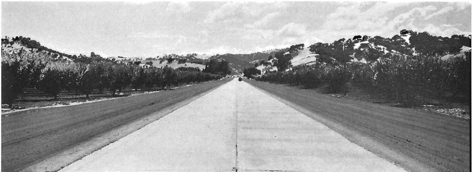
Right of way agreements secured by Division of Highways protect the Vacaville cut-off through beautiful Vaca Valley from business encroachments.
