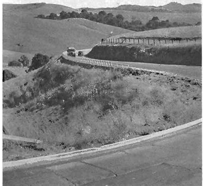
Narrow roadway with blind curves over railroad tunnel in Niles Canyon between Niles and Sunol. (Below) Circuitous routing with blind curves on Franklin Canyon Road.
