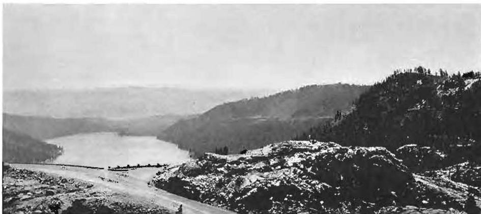
Rocks were blasted and safe entrance way and parking area constructed.
