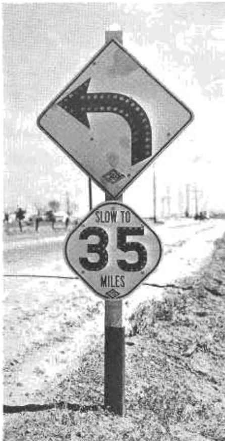
Warning signs tell safe driving speed for curve zones on California Highways
