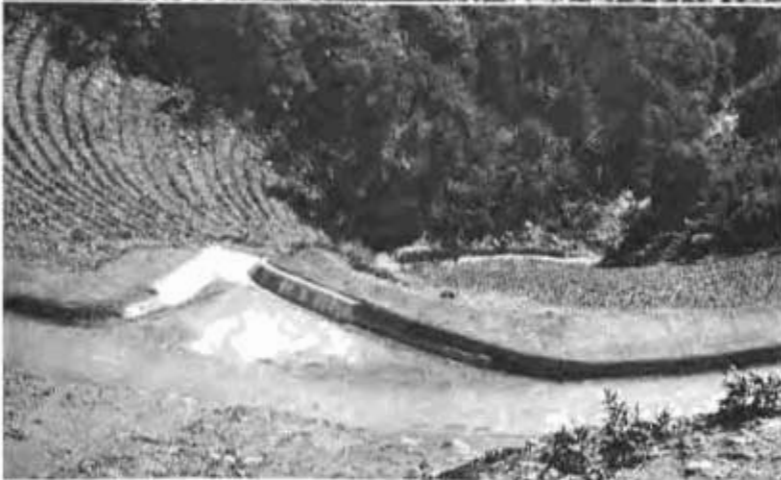
Drainage features of Angeles Crest Highway in Los Angeles County. Upper left—general view of terrain with spillway entrance in foreground. Below—grouted rock channel entrance to paved spillway. Upper right—paved spillway and planted slopes. Below—spillway paved with 18 by 36 inch concrete blocks.
