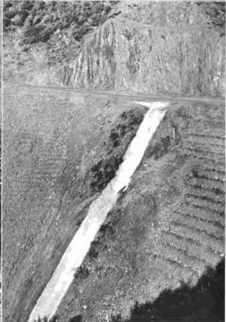
Drainage features of Angeles Crest Highway in Los Angeles County. Upper left—general view of terrain with spillway entrance in foreground. Below—grouted rock channel entrance to paved spillway. Upper right—paved spillway and planted slopes. Below—spillway paved with 18 by 36 inch concrete blocks.
