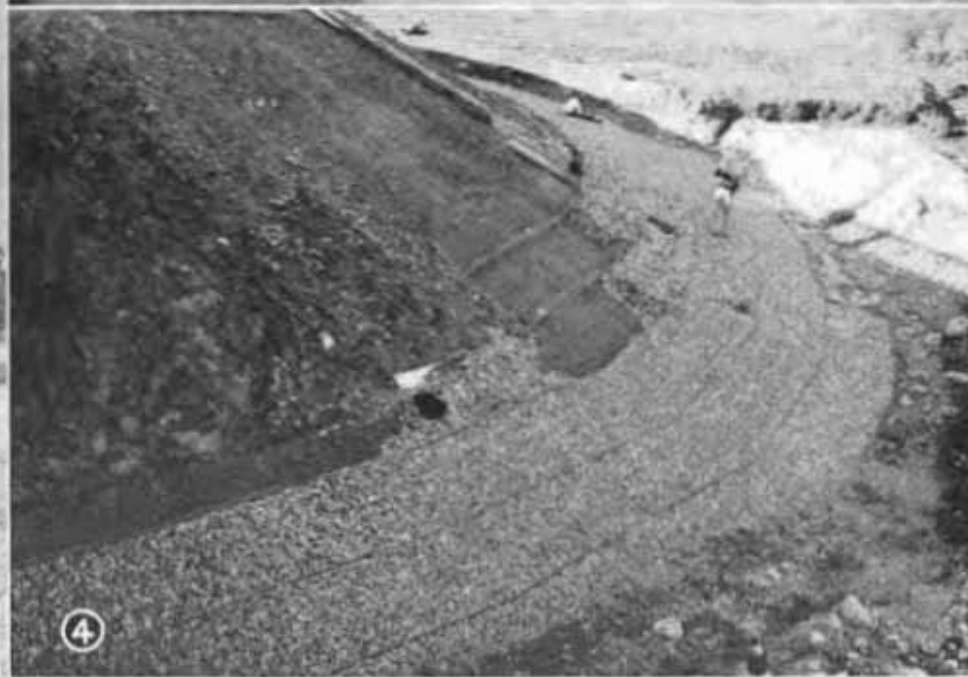
Picture No. 1 shows bar formed below steel tetrahedron jetty indicated by X line. 2—Cable connected jackstraws used to stop bank erosion. 3—Steel rail and wire fence backfilled with rock and brush. 4—Wire mesh and rock mattress.
