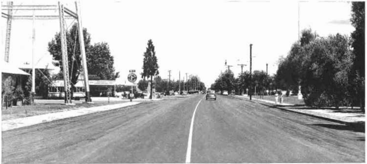
Newly paved portion of Orange Belt highway in Tulare County has 22-foot roadway with 17-foot shoulders on each side.
