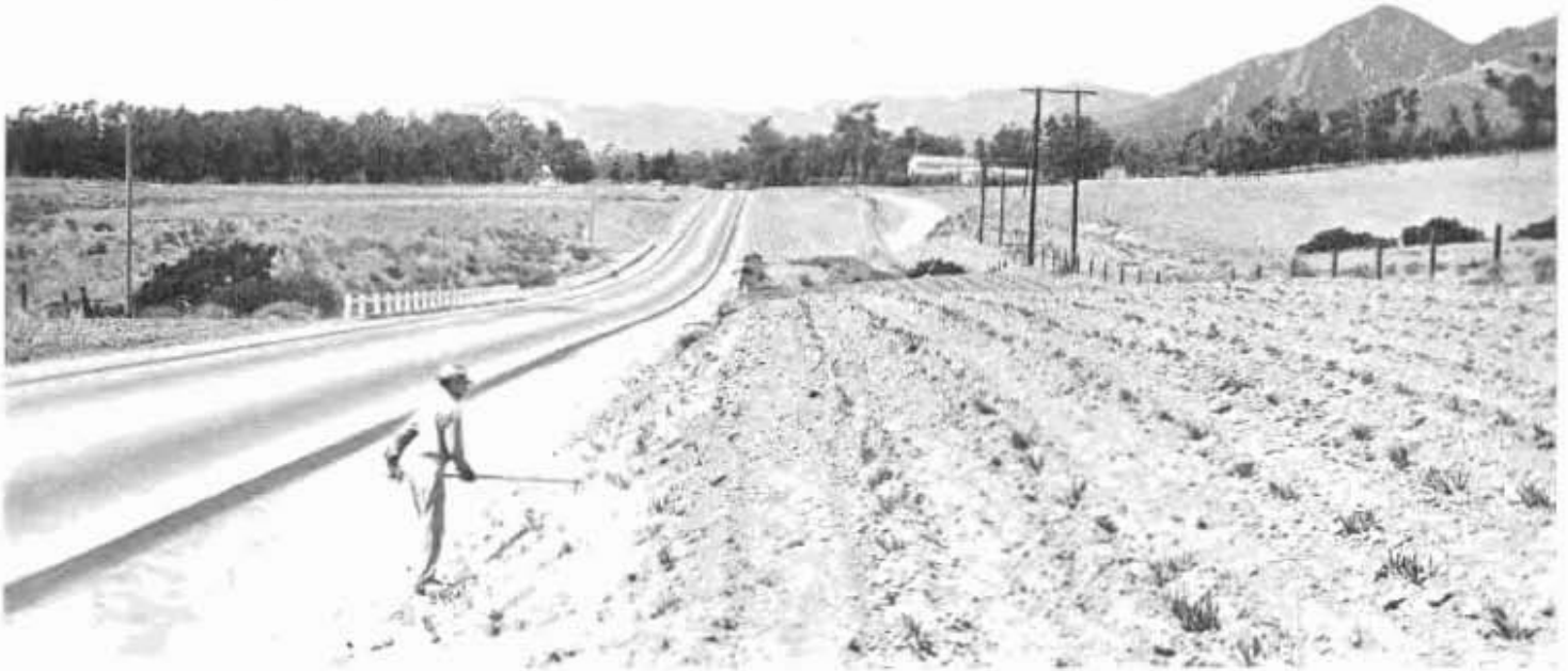
Planting and cultivating extensive right of way on Coast Route State Highway 56 with ice plant to prevent erosion.
