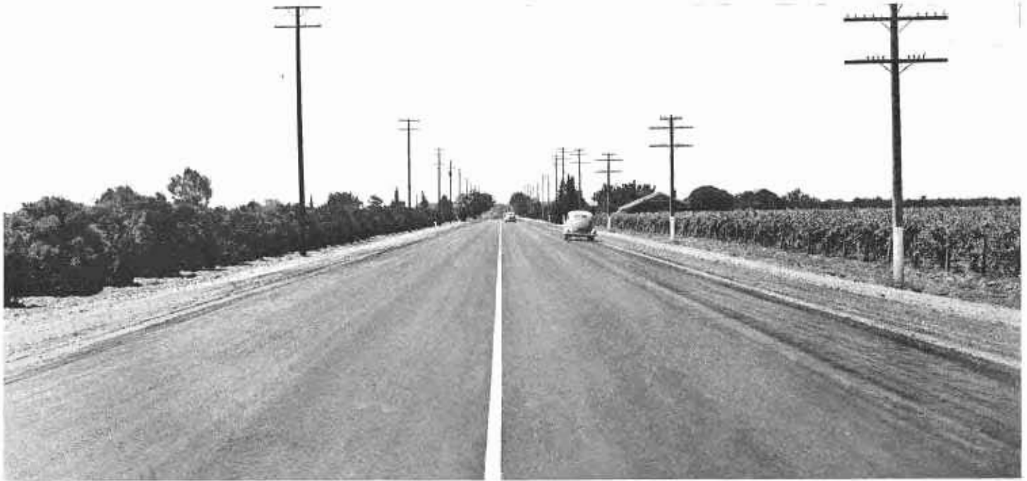
Portion of recently completed link of Sierra-to-Sea highway through Hanford which avoids business section congestion in city.
