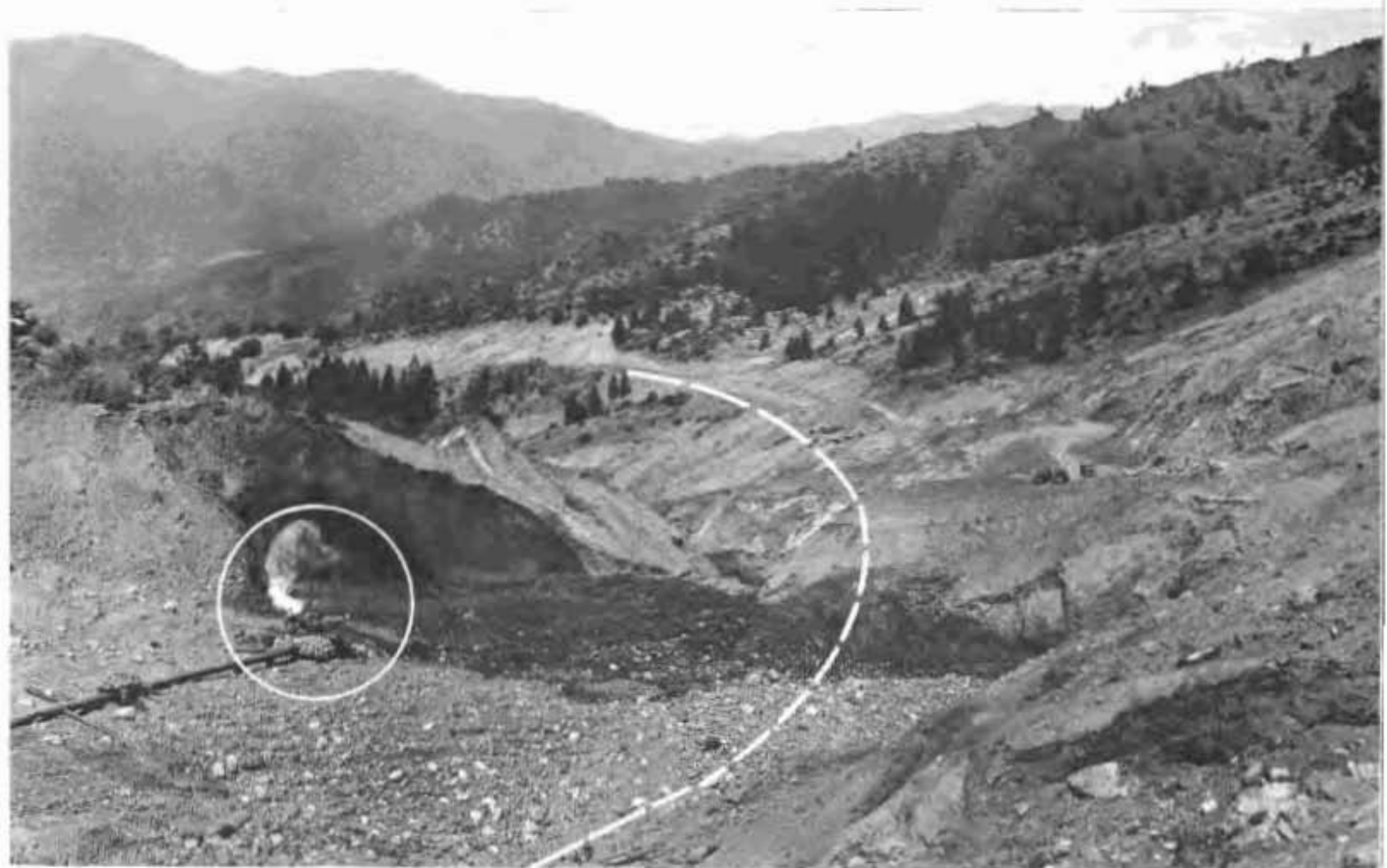
View from summit of Oregon Mountain looking down over proposed highway grade indicated by white line. Hydraulic giant at work in circle.
