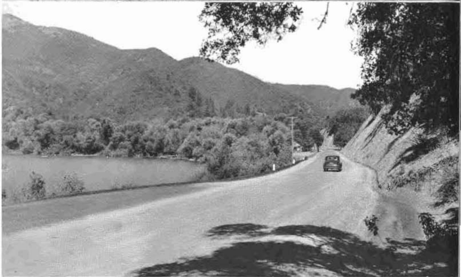
Two views of the recently reconstructed section of State Route 15 along the north shores of Laurel Del Lake and Blue Lake generally known as the "blue lakes" in Lake County. Fourteen curves were eliminated in a distance of two miles and parking areas constructed at vista points.
