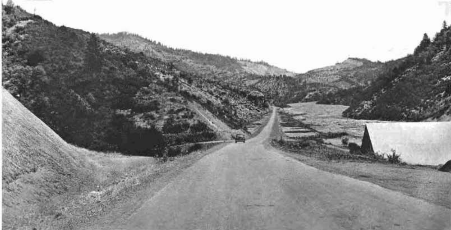
Roadway in Oregon Gulch built with hydraulic tailings. Log cribs, fence and brush were used to control deposit of tailings.
