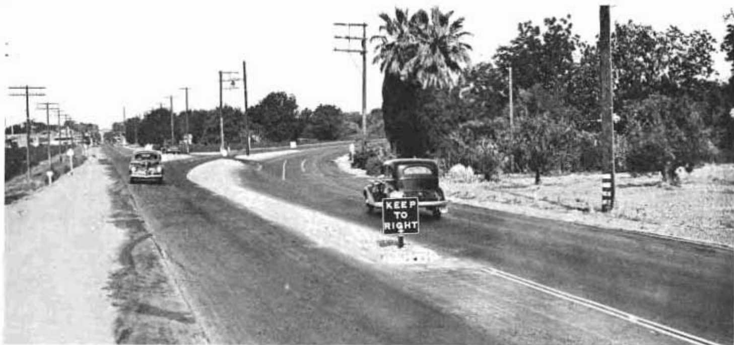
Improved section of highway near Hanford showing channelization of intersection at Lacey Boulevard which is provided with sodium vapor lamp amber flashers and red reflectors.
