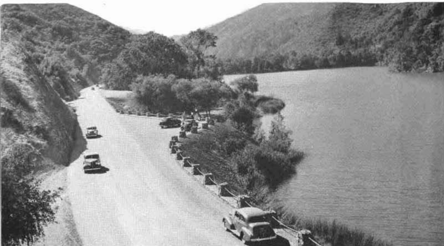
With roadway widened and curves eliminated convenient parking areas are provided on State Route 15 along the north shores of the Blue Lakes.
