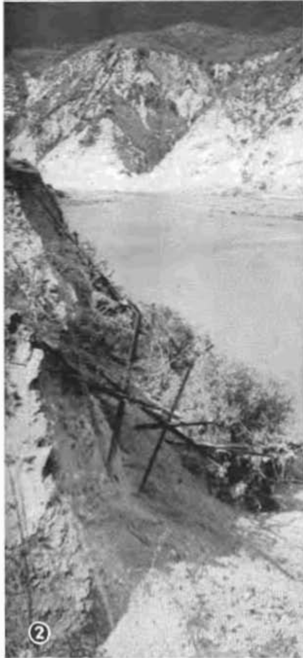
Picture No. 1 shows bar formed below steel tetrahedron jetty indicated by X line. 2—Cable connected jackstraws used to stop bank erosion. 3—Steel rail and wire fence backfilled with rock and brush. 4—Wire mesh and rock mattress.
