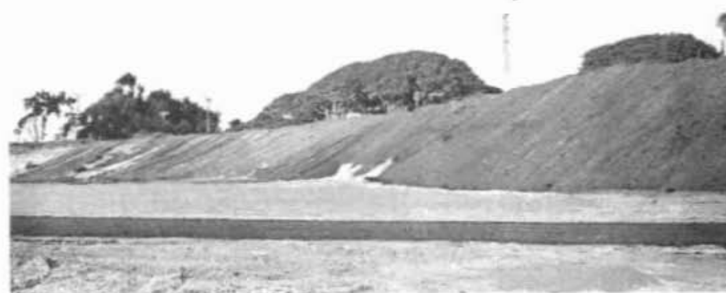
Protective cover produced on sandy slope by seeded thin topsoil blanket.
