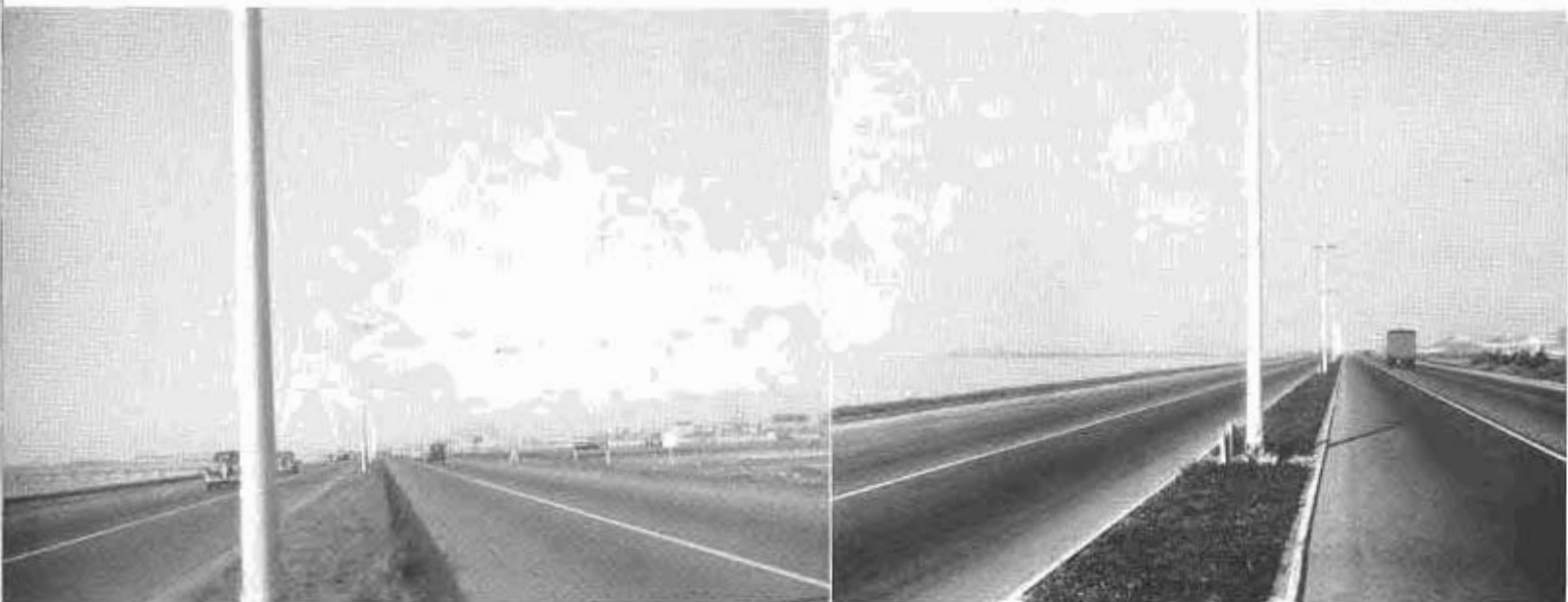
Typical planting of entire east shore approach. Group plantings along Berkeley Aquatic Park, with ice plant ground cover on bayside and center strip.
