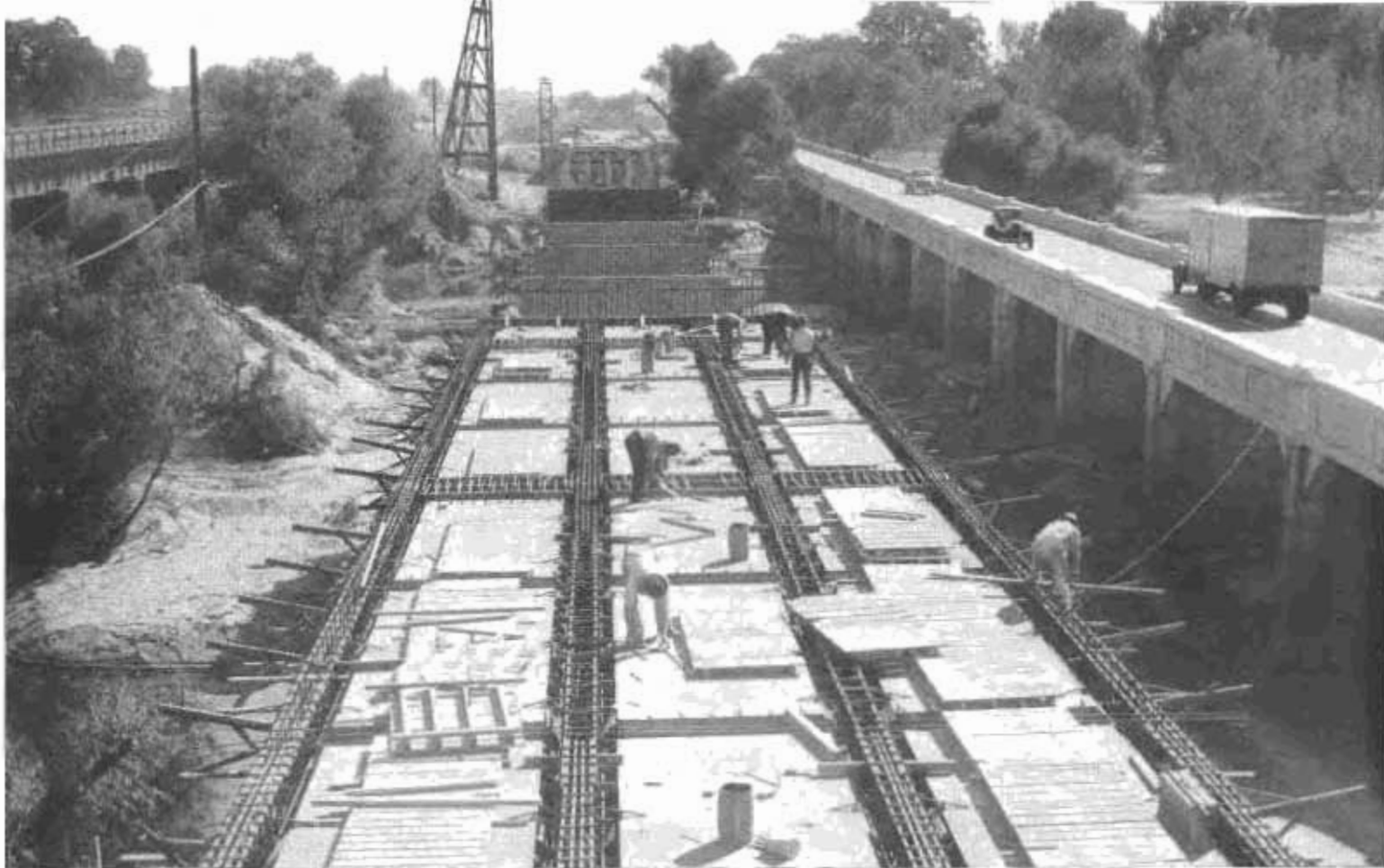
The new bridge will be 1024 feet long with a 27-foot roadway. The existing bridge will carry southbound traffic.
