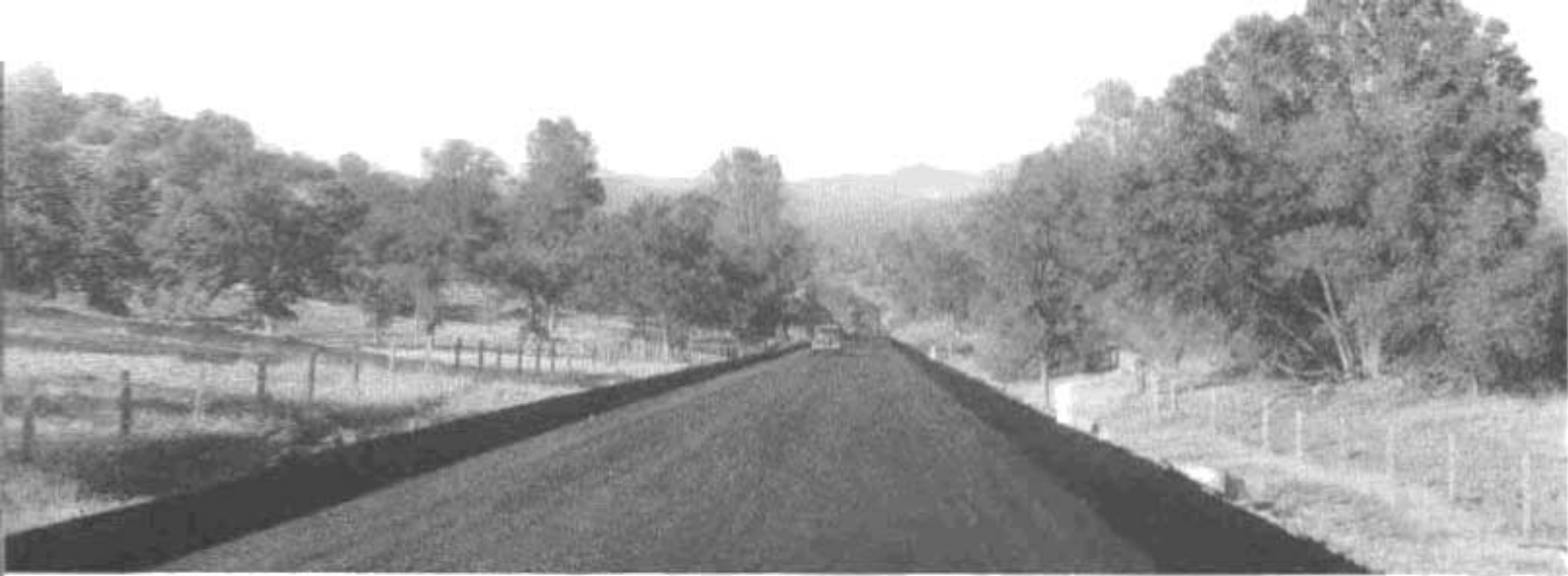
Section of new direct 10 mile highway link into Yosemite replacing 13 miles of narrow, tortuous old road.
