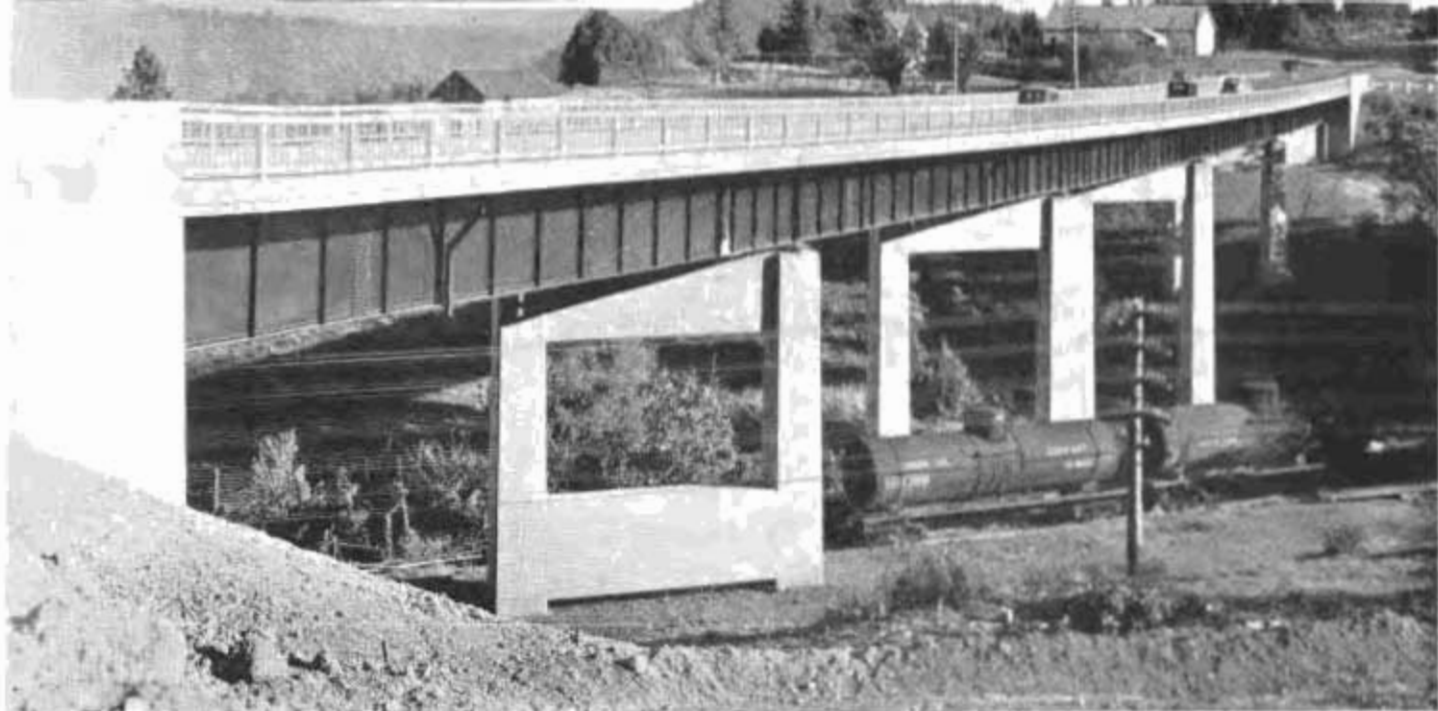
Recently completed grade separation structure at Colfax, Placer County, carrying U. S. 40 over main line railroad tracks.
