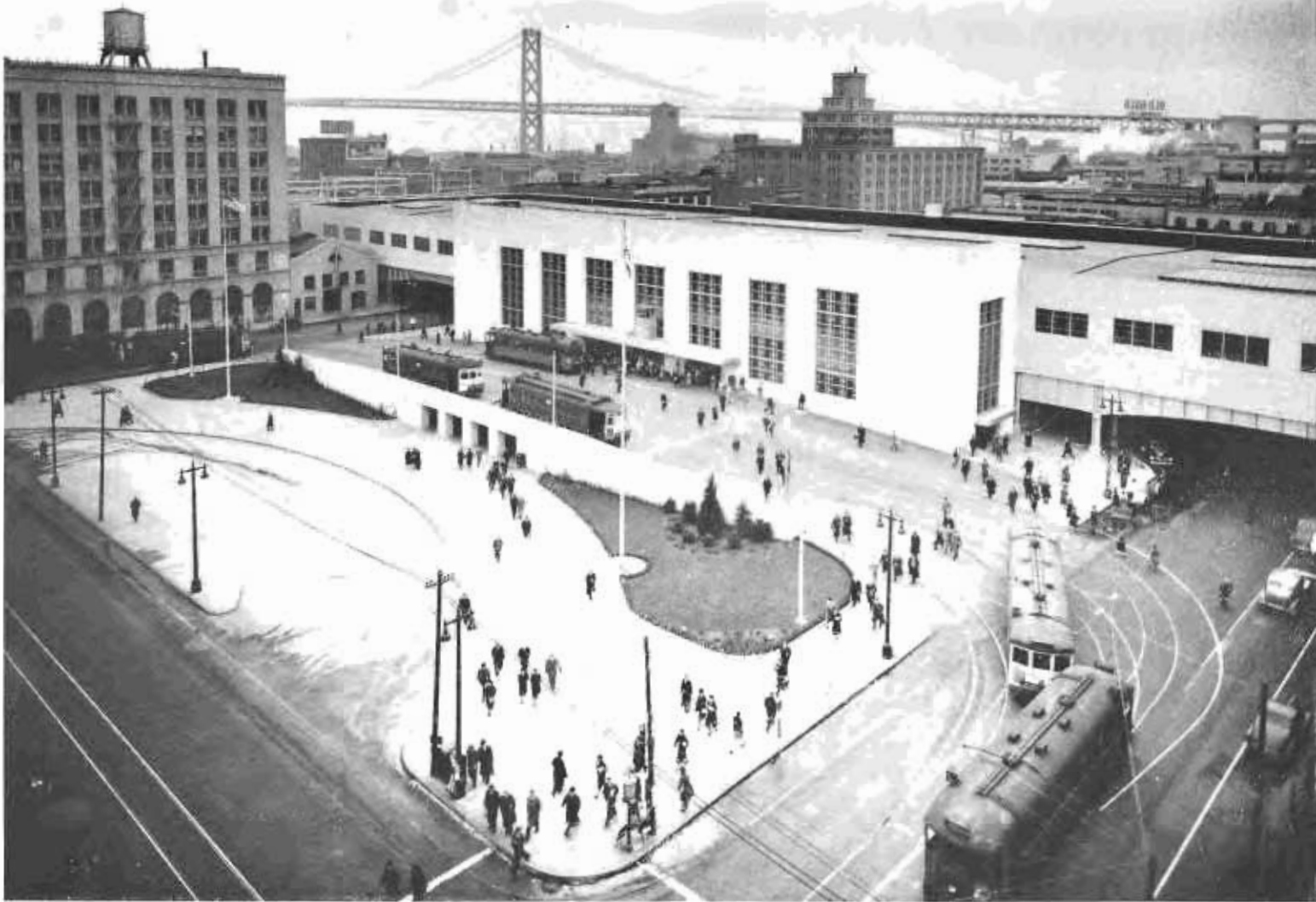
Terminal Plaza showing trolley car loop ramp to mezzanine level and street entrances for pedestrians and automobile passengers.
