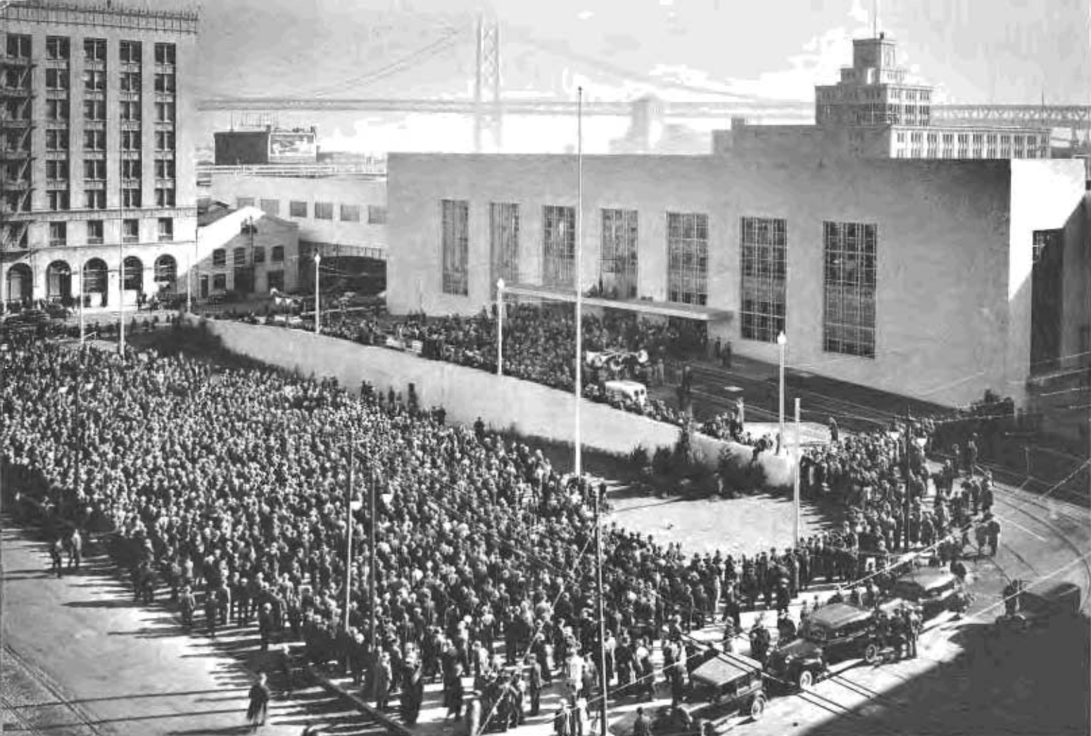
Scene at official opening and dedication of San Francisco-Oakland Bay Bridge Electric Railway Terminal Building in San Francisco.
