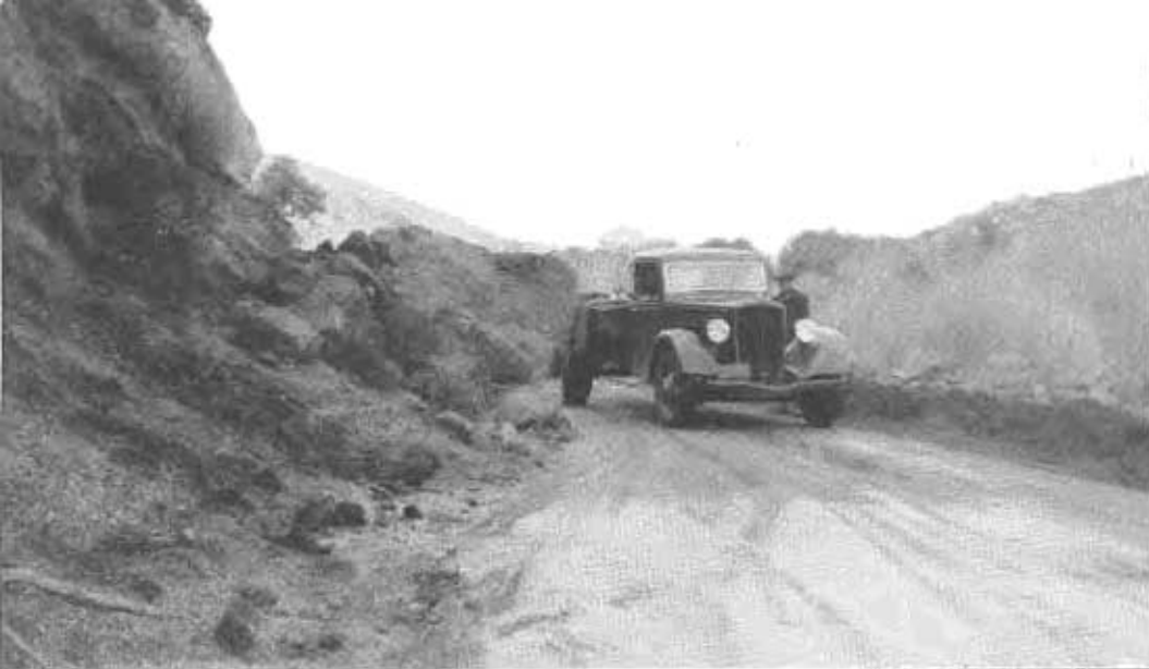
Top—This picture of a section of State Sign Route 94 in San Diego County shows a narrow road with poor alignment and hazards caused by inadequate slopes. Center—Poor alignment and many blind curves on this stretch of State Route 195 near Oceanside, San Diego County. Bottom—One of many “dips,” frequently flooded, on State Sign Route 94. It exists because there are no funds for a bridge.
