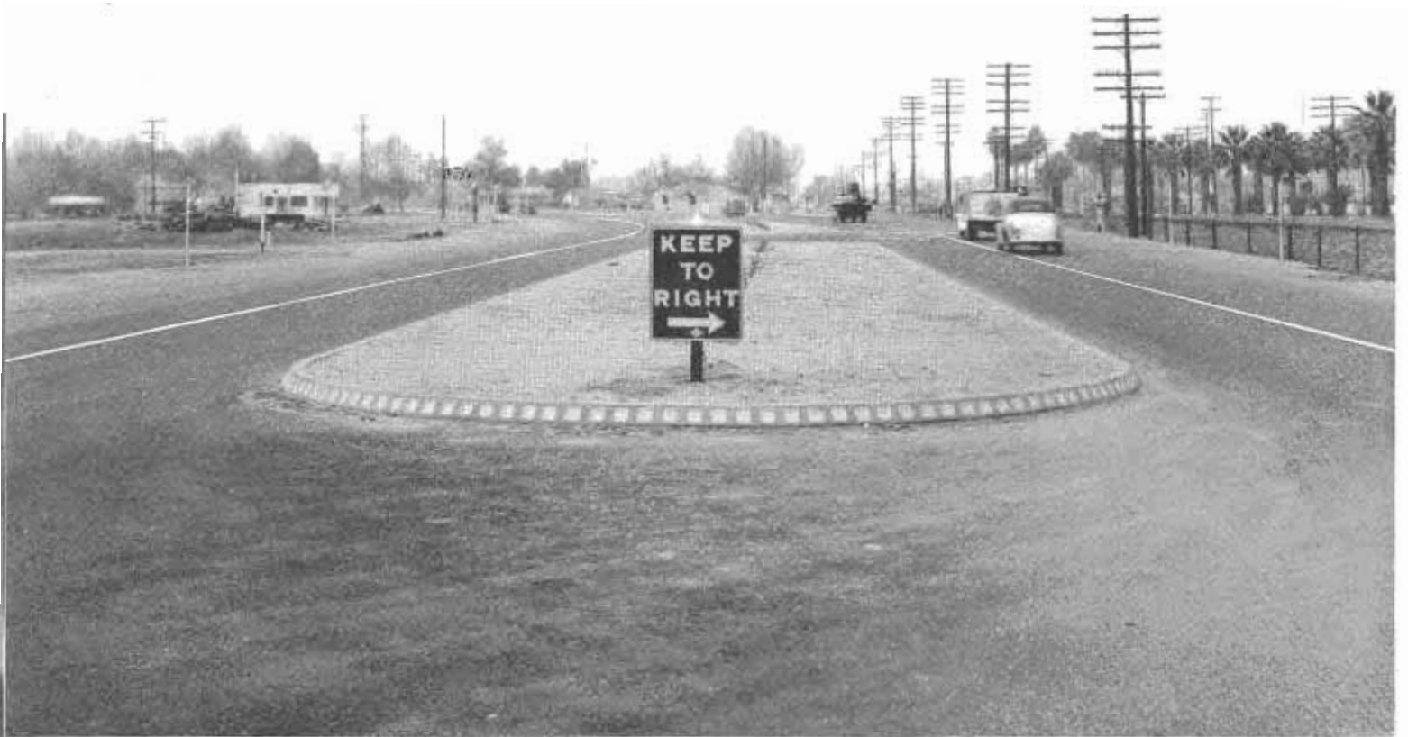
Channelization Islands on Divided Highway link of U. S. 99 relocation in Selma have 6 inch recessed curbs.
