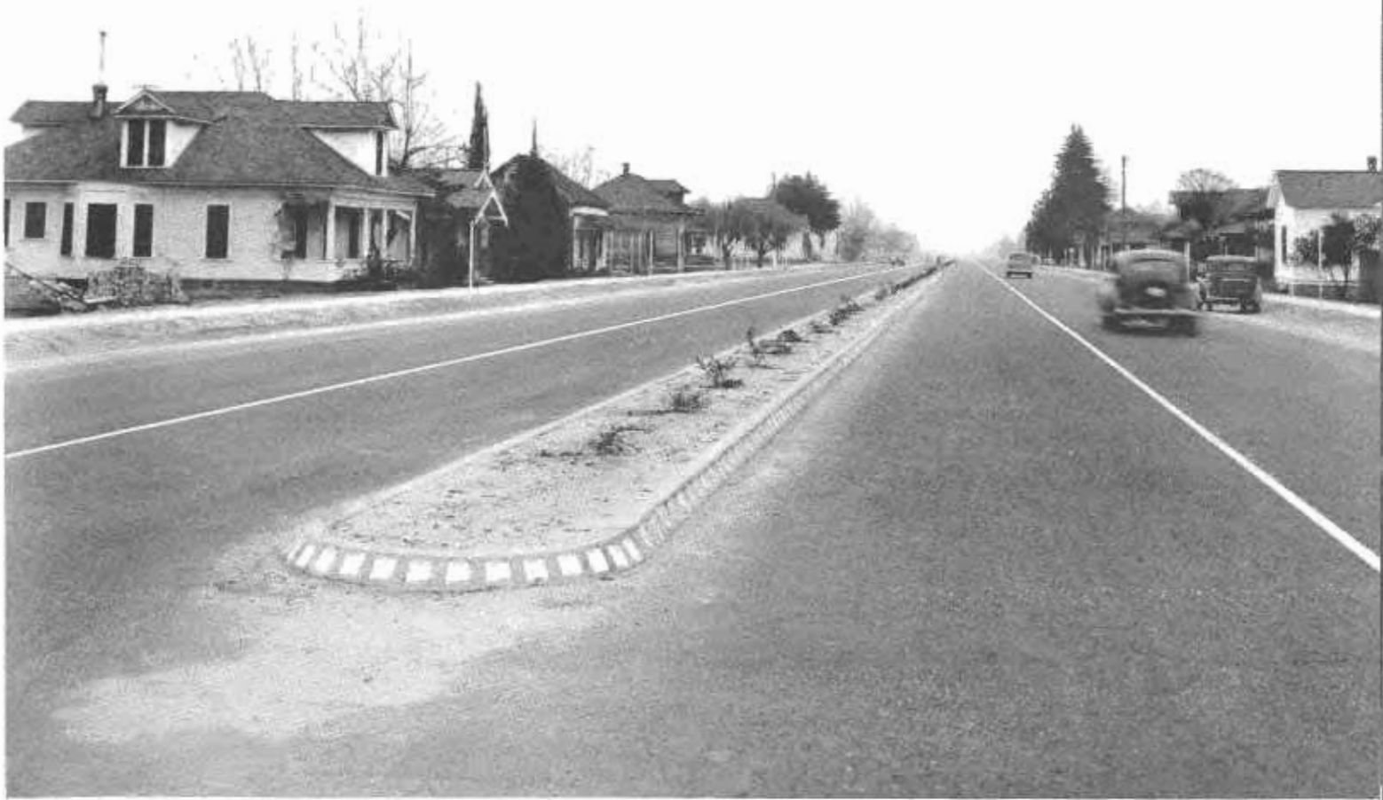
Two views of Divided Highway on relocation of a short link of U. S. 99 in city of Selma. Separation strips are bordered by six inch curbs recessed and painted white to reflect headlight beams.
