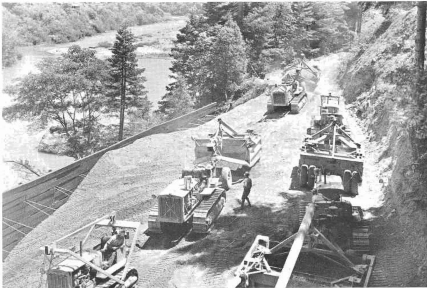
This picture shows construction crew back-filling bulkheads with porous river gravel.
