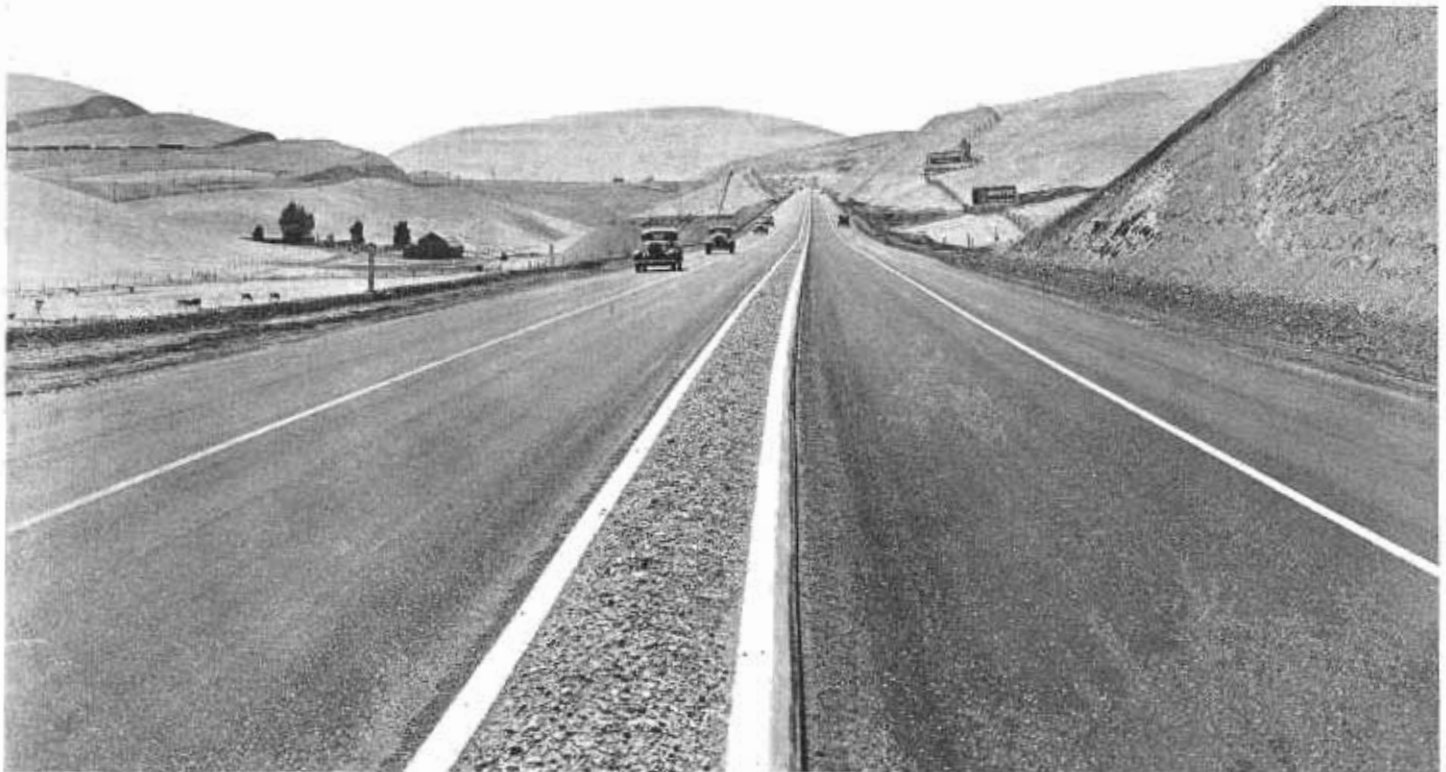
State Route 45 through Altamont Pass in Alameda County. Two 22-foot road-mix surface lanes with 4-foot dividing strip.
