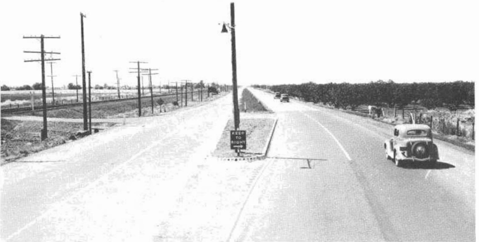
View of new Merced highway, on right, showing its elevation to escape flood waters. Old highway on left.
