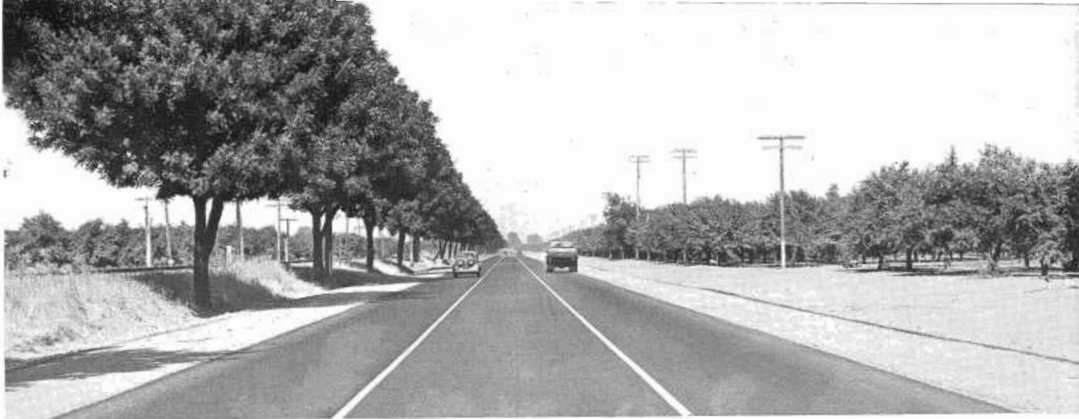
State Route 2 near Morgan Hill in Santa Clara County, showing 33-foot asphalt concrete pavement.
