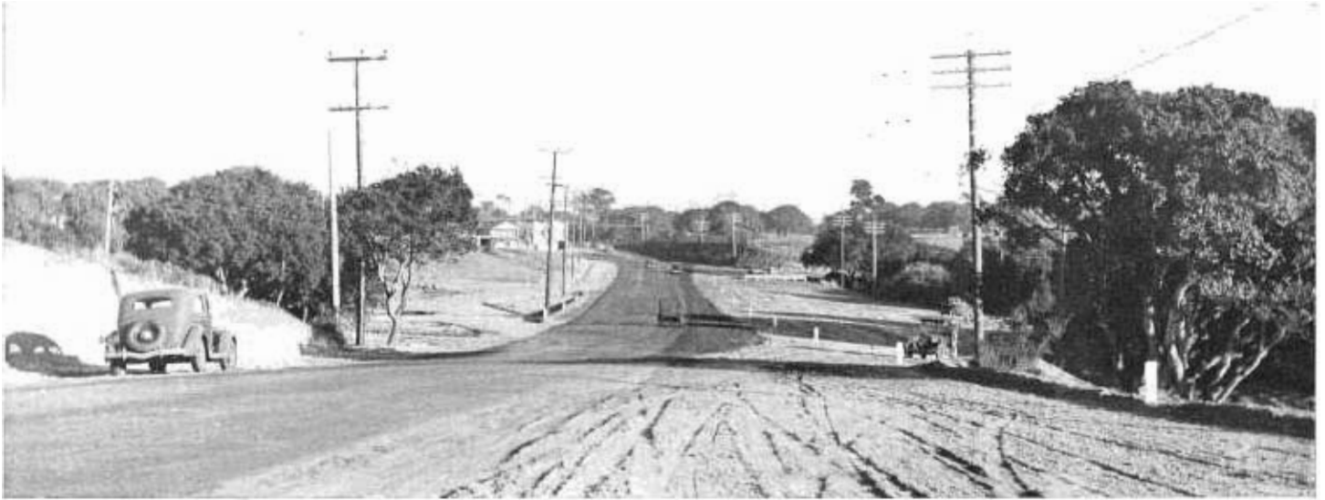
This picture shows a fine example of what cities can do with their 1 cent gas tax funds. It was taken in Monterey. The old dirt road on the right followed a route to the right of the line of white posts. It was replaced by the modern paved alignment shown on the left.
