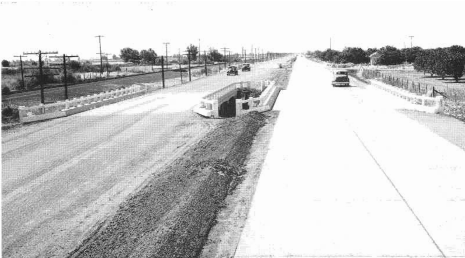
Another view of Merced highway, showing difference in grade between new road, right, and old road, left.
