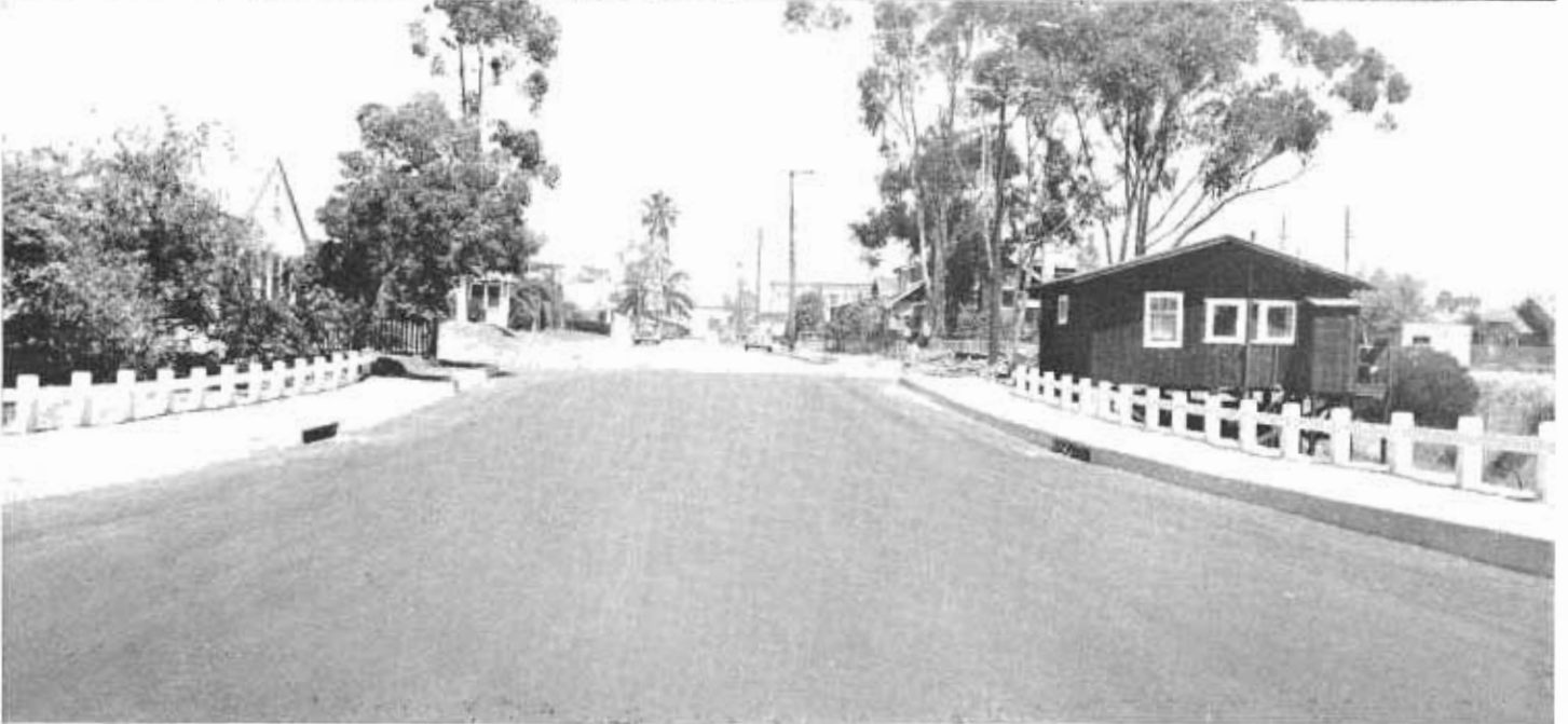
These two views vividly show what the City of San Diego was able to do with \frac{1}{4} cent city street gasoline tax funds. The picture at the top shows the site of the Douglass Street extension before construction. The one at the bottom shows the extension after completion. Both photographs were taken from the same spot. The slope at the left of the house in the upper picture was filled in to make the grade shown in the picture below.
