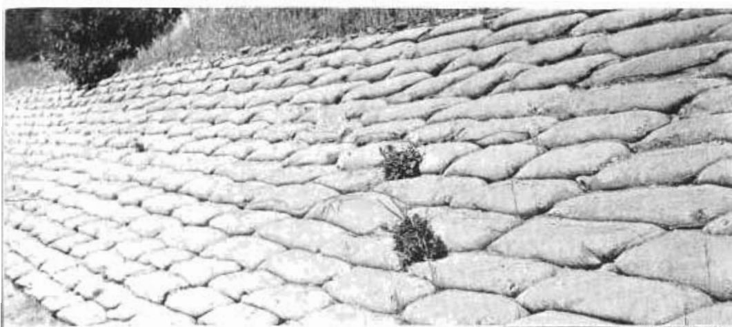
From top to bottom—Sacked concrete revetment on Grizzly Creek, Lake County. Heavy wire mesh revetment on Cow Creek in Shasta County. Reinforced asphalt concrete channel lining near Fillmore in Ventura County. Sacked concrete in use ten years on the Van Duzen River in Humboldt County.
