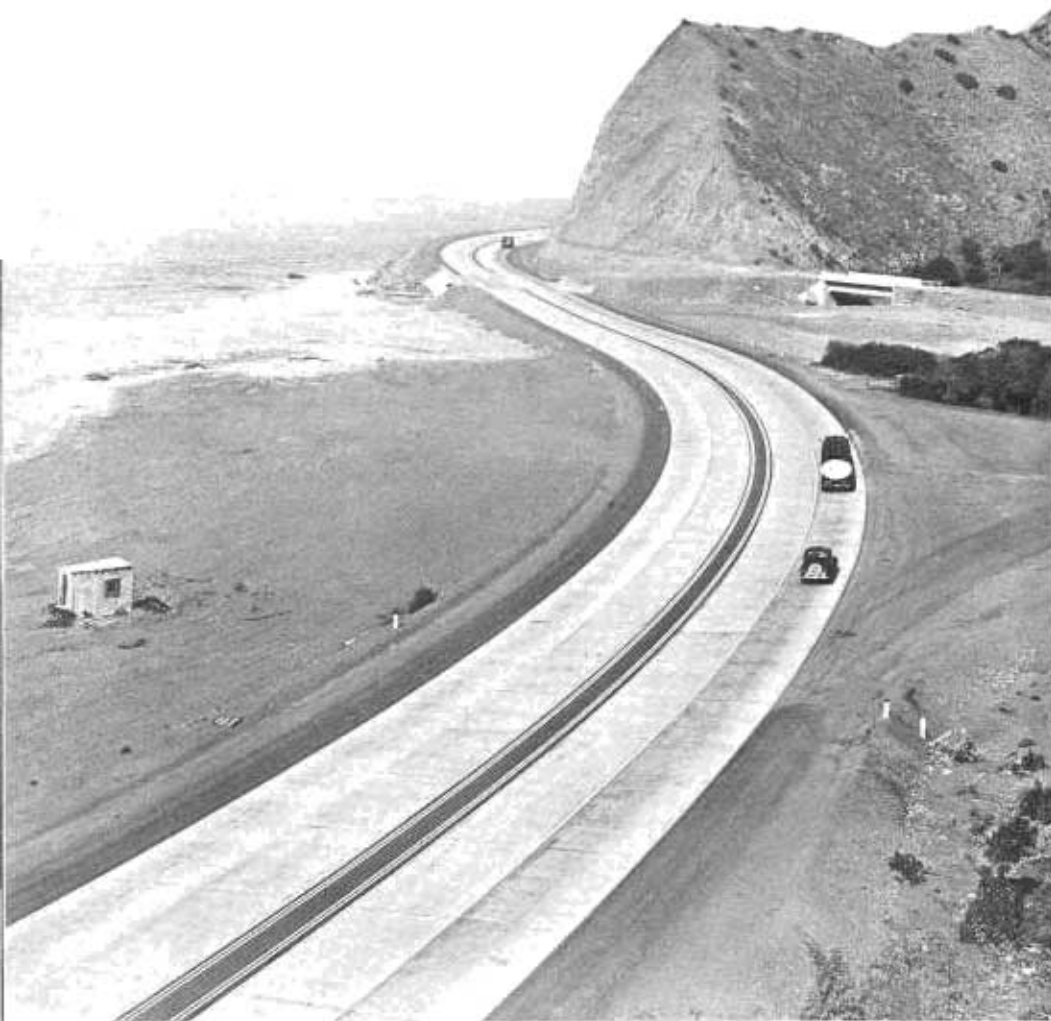
Coast Highway near Big Sycamore Canyon, Ventura County. Two 22-foot portland cement concrete pavement lanes separated by a 6-foot plant-mix center strip.
