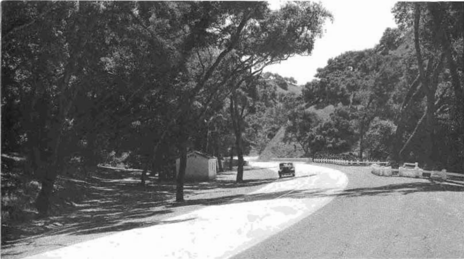
One of the scenes of sylvan beauty on the realigned Route 2 between Gaviota Pass and Santa Ynez River.
