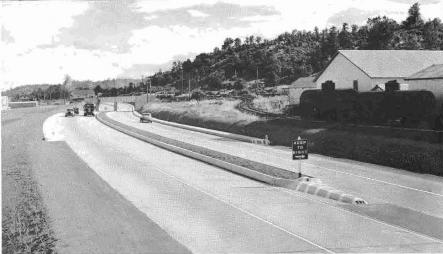
Two views of recently completed modern, 4-lane subway with 8-foot division strip on U. S. 99 near Redding.
