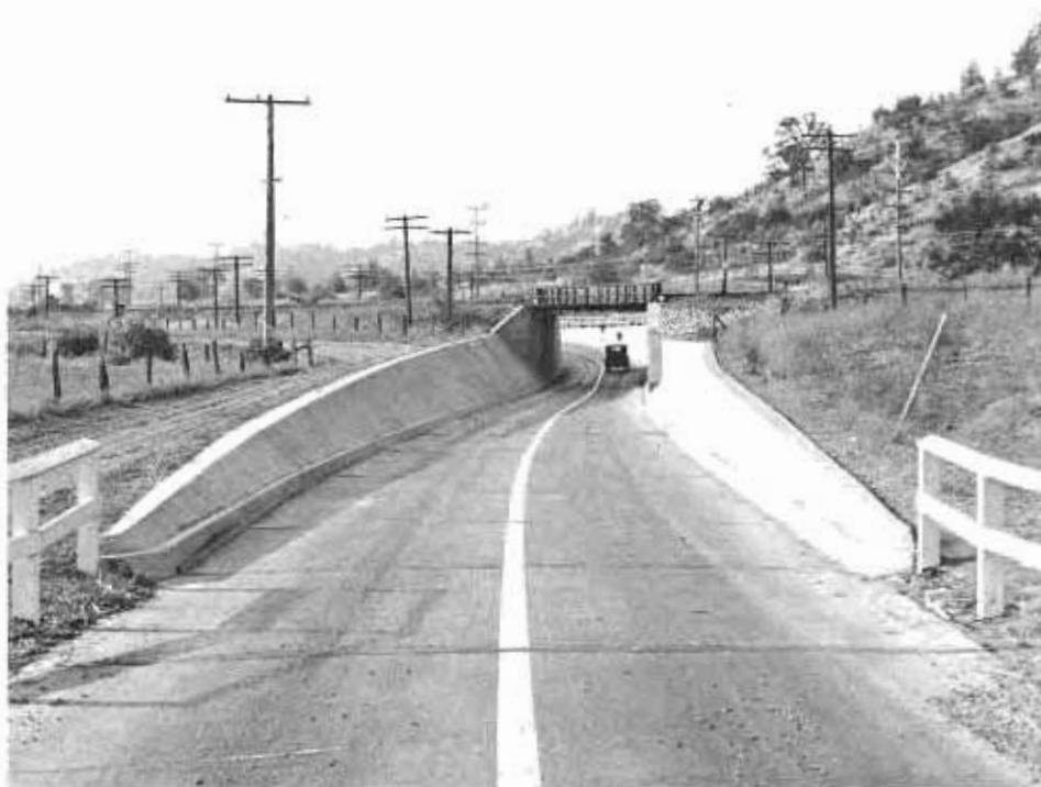
Old subway on U. S. 99 near Redding built in 1923 had 15-foot curved roadway.
