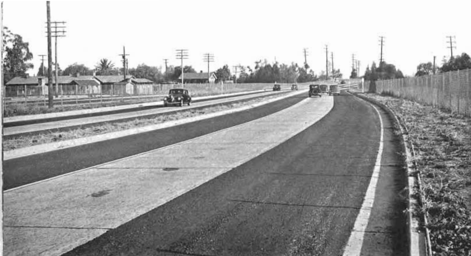
Completed section of Arroyo Seco Parkway beginning at Glenarm Street in Pasadena. Designed as a "freeway" it has six lanes divided by a raised separation strip and no stop lights or intersections in its nine-mile length between Pasadena and Los Angeles.
