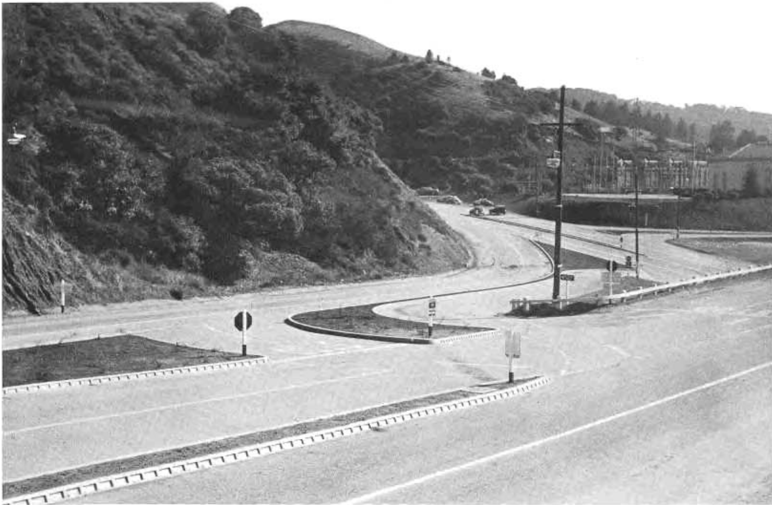
Another view of the channelization islands and continuous dividing strip at the intersection entrance to Landvale Road.
