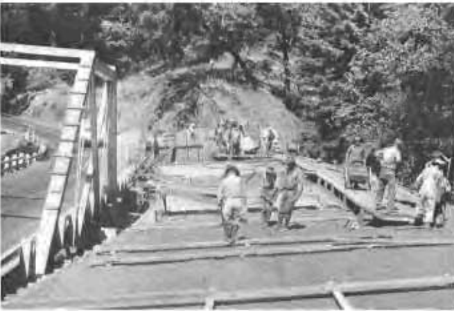
3—Partially completed new deck structure with traffic still using old bridge.
