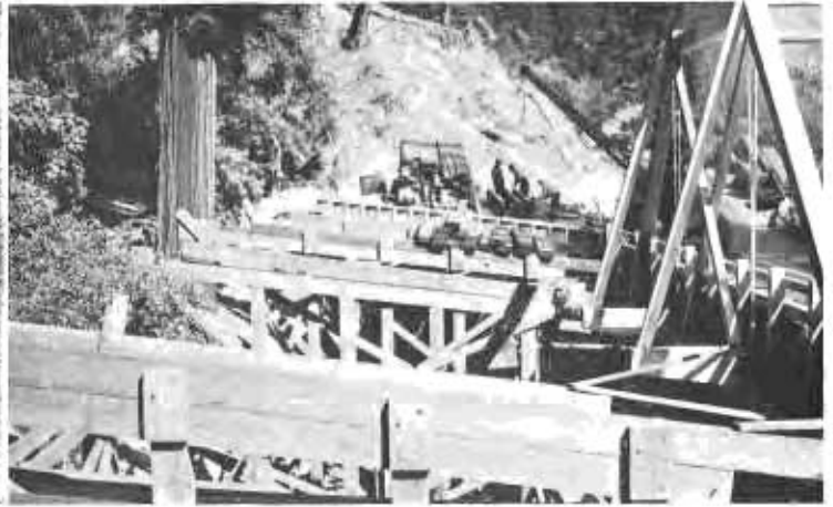
2—Constructing temporary supports on which new deck structure was built.
