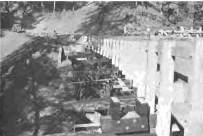
5—Picture of sliding deck structure approaching final position on permanent supports.
