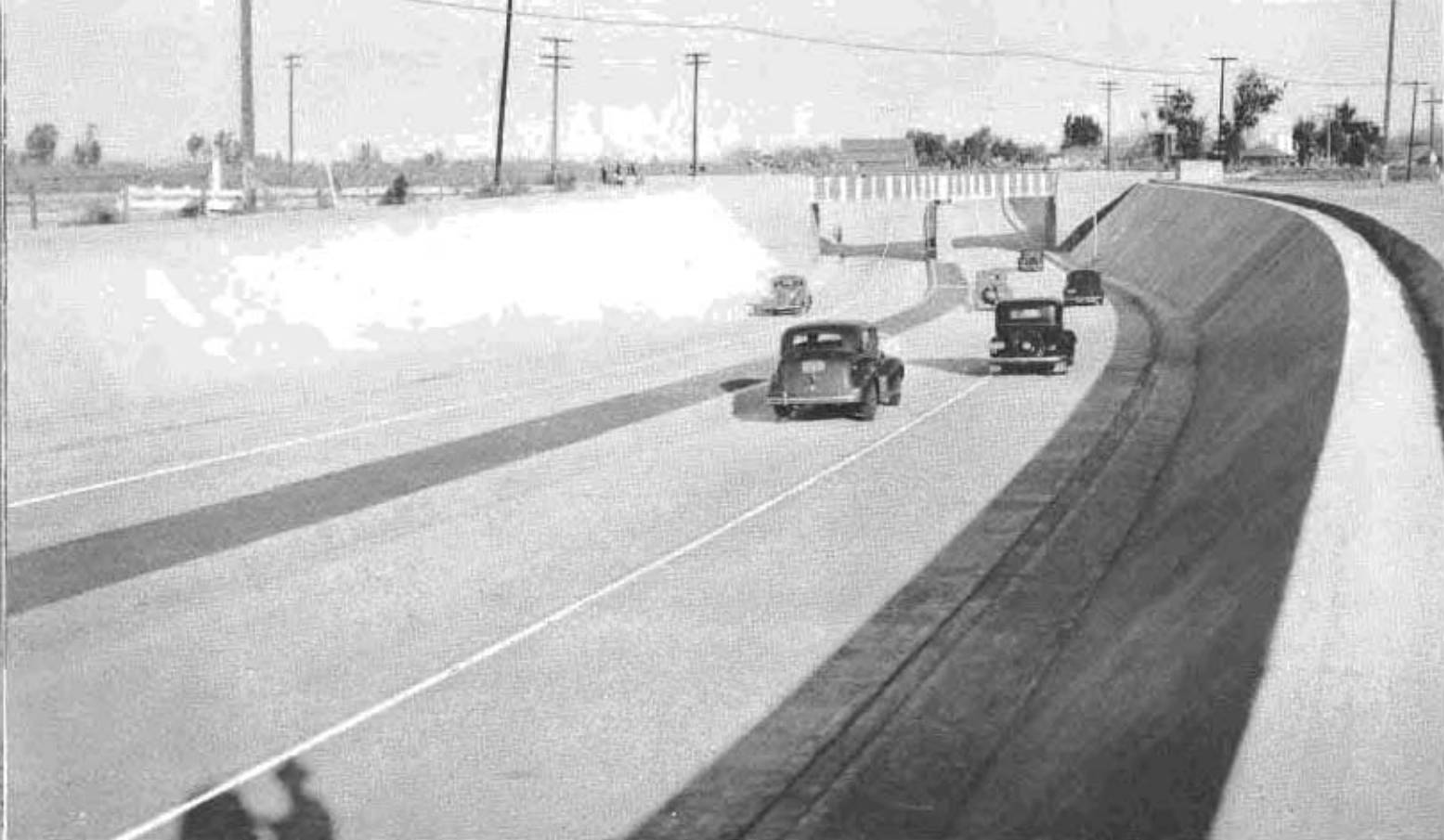
Recently completed underpass at Livingston, providing a four-lane divided highway beneath Southern Pacific tracks and eliminating a traffic hazard on U. S. 99.
