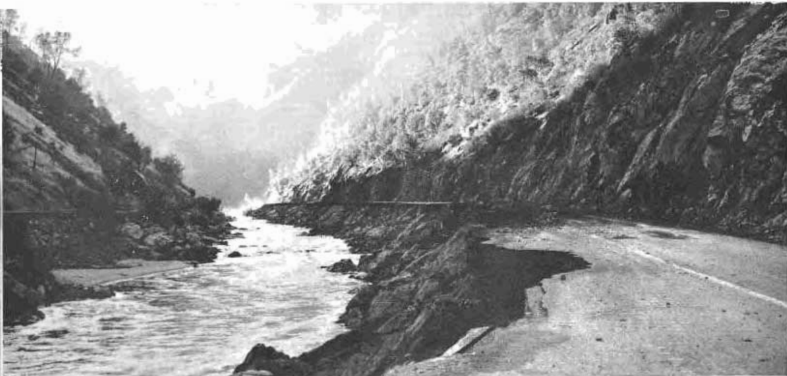
One section of Yosemite All-year Highway showing typical damage done by Merced River flood in 1937.
