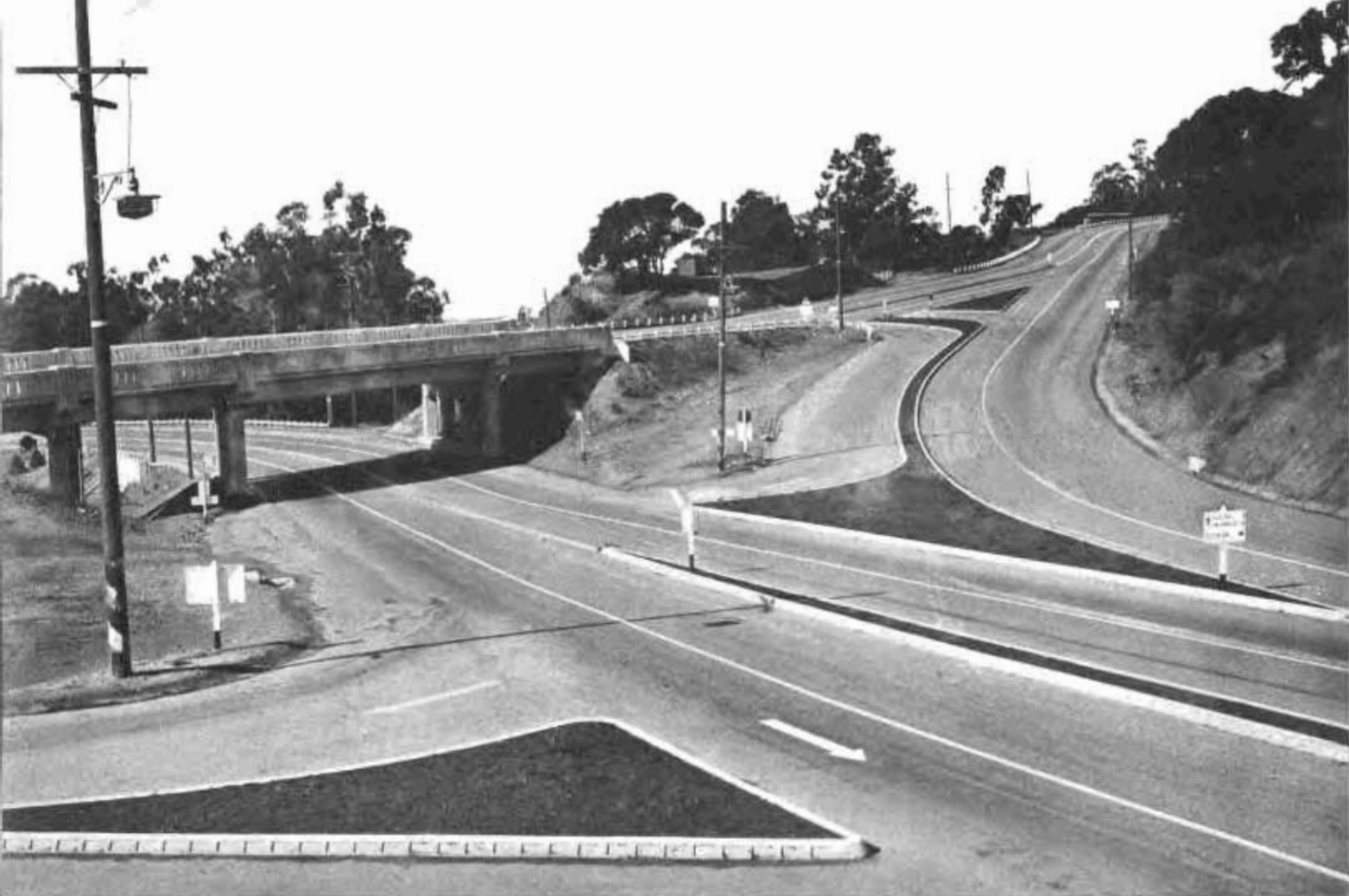
View of highway grade separation and divisional islands at intersection of Routes 75 and 206 near Broadway Tunnel in Oakland.
