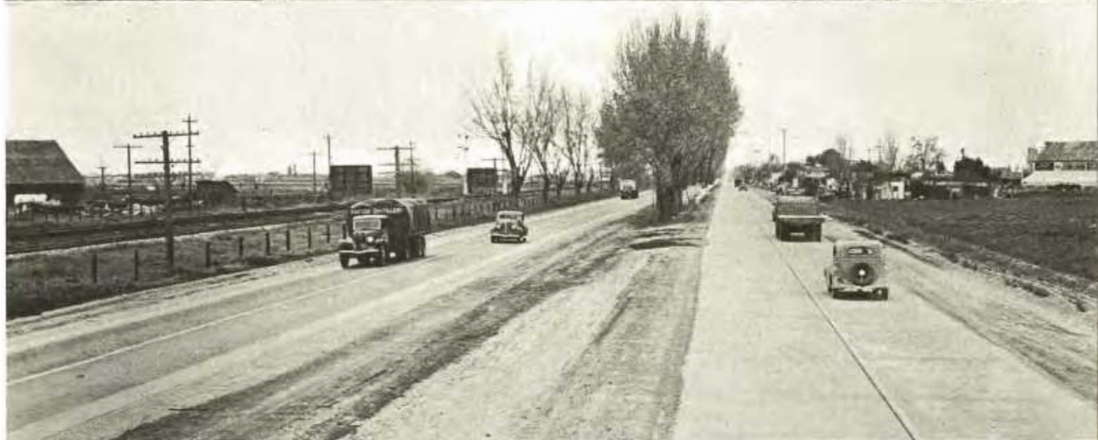
At top—Looking north from Modesto on U. S. 99 showing divisional island at transition from 4-lane undivided to four-lane divided highway. Center—Guard rail construction in separation prevents cross-over traffic except at designated points. Bottom—End of transition segment showing separation strip and trees that bordered roadside of old pavement on right with newly added pavement lanes on left.
