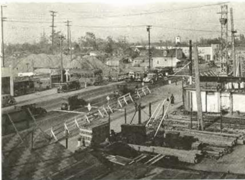
Before and after views of dangerous grade crossing on Firestone Boulevard in Los Angeles. Overhead structure carries railroad tracks.
