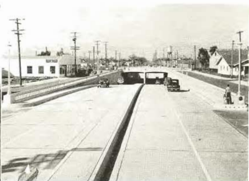
Where U. S. 99 formerly crossed the railroad tracks at Wilson Way in Stockton, motorists now pass safely through a divided 4-lane underpass.
