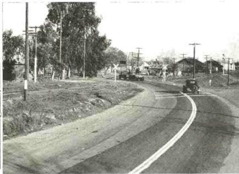
Railroad grade crossing on "S" curve at Livingston on U. S. 99 and underpass with 4-lane divided highway that eliminated it.
