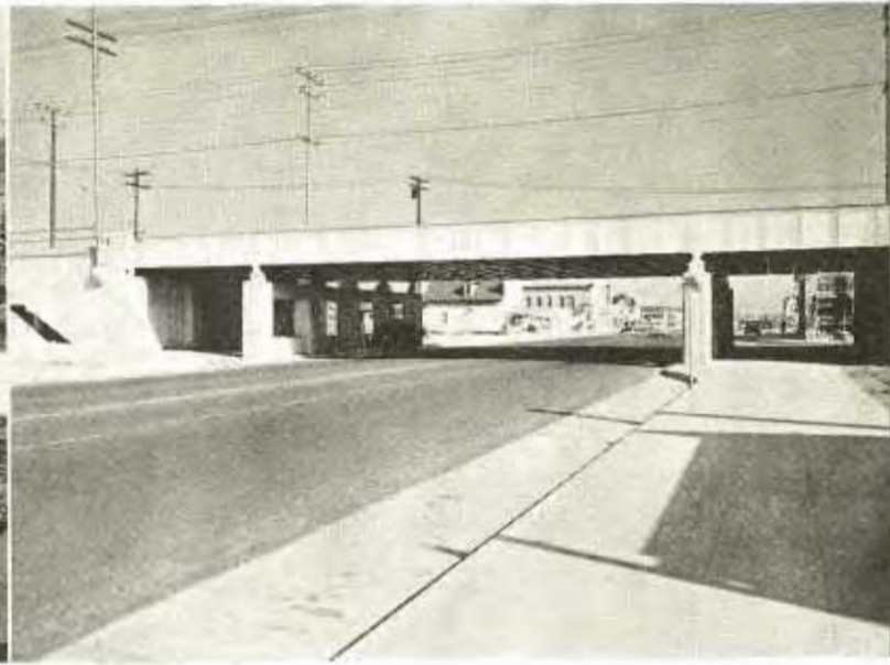
Before and after views of dangerous grade crossing on Firestone Boulevard in Los Angeles. Overhead structure carries railroad tracks.
