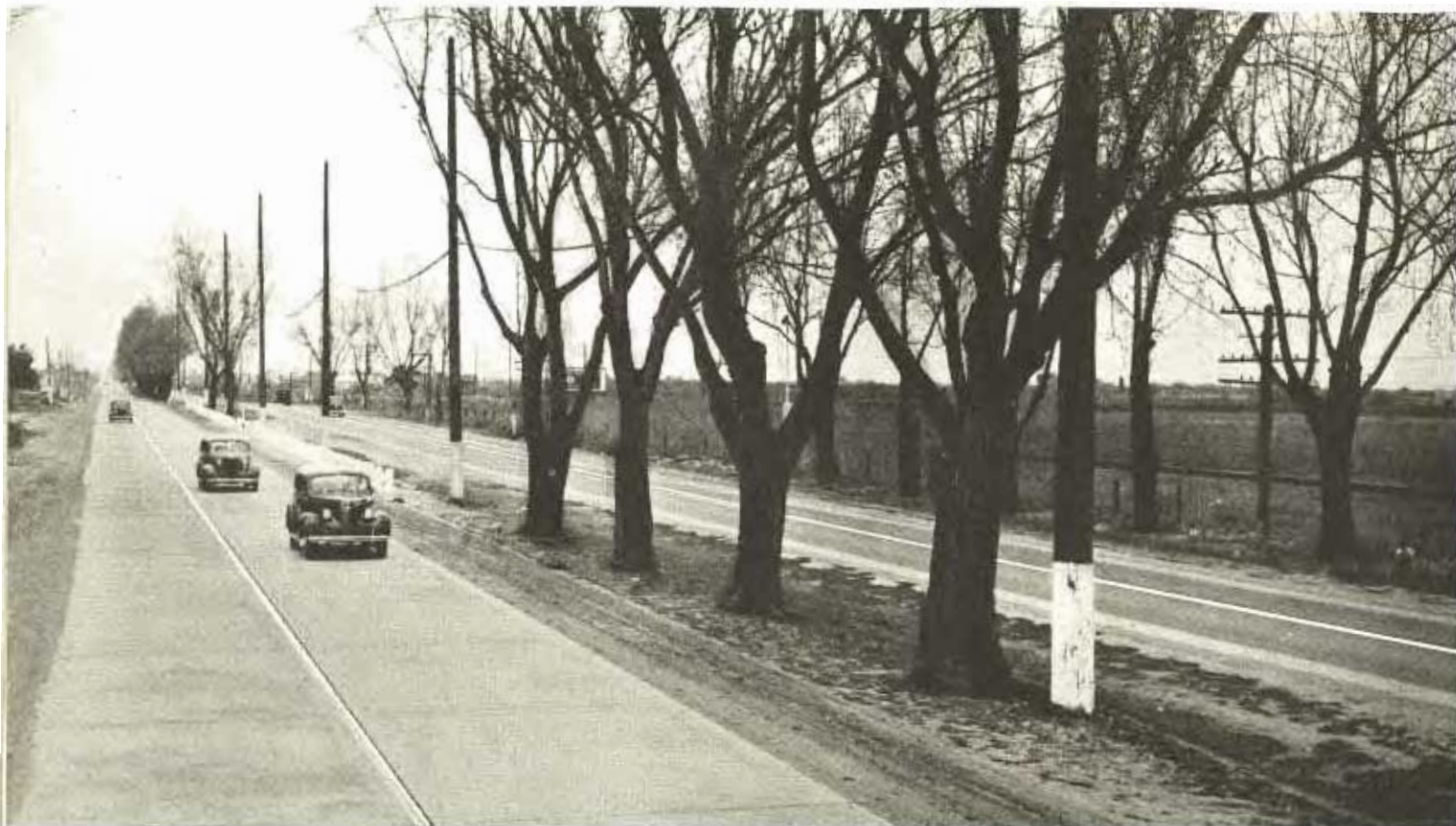
Preservation of roadside trees in 29-foot separation strip marks transformation of this section of U. S. 99 north of Modesto from a 2-lane into a 4-lane divided highway.
