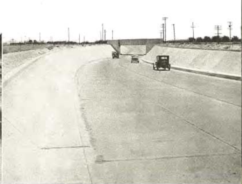
Another grade crossing on an "S" curve at Delano on U. S. 99 in Kern County and 4-lane subway that replaced it.
