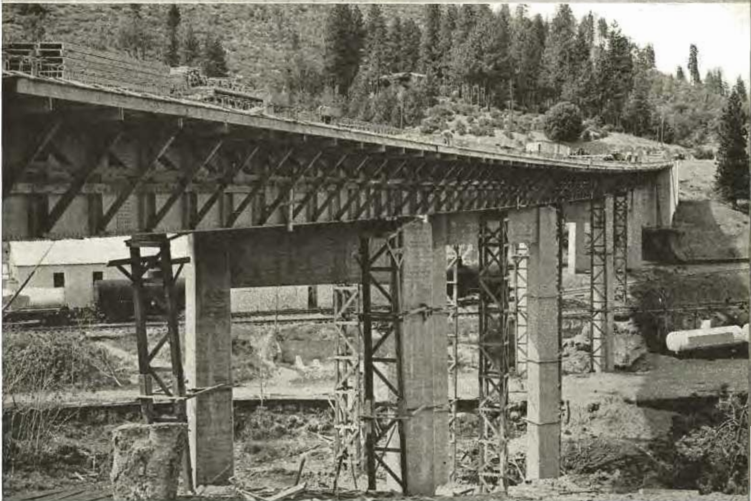
At top—grade crossing of tracks of Southern Pacific main line in city of Colfax, Placer County, where U. S. 40 makes numerous abrupt turns for through traffic. A relocation follows the east side of the city eliminating turns and carrying the highway over the railroad tracks on a steel and reinforced concrete bridge structure 504.30 feet long, shown in bottom picture under construction.
