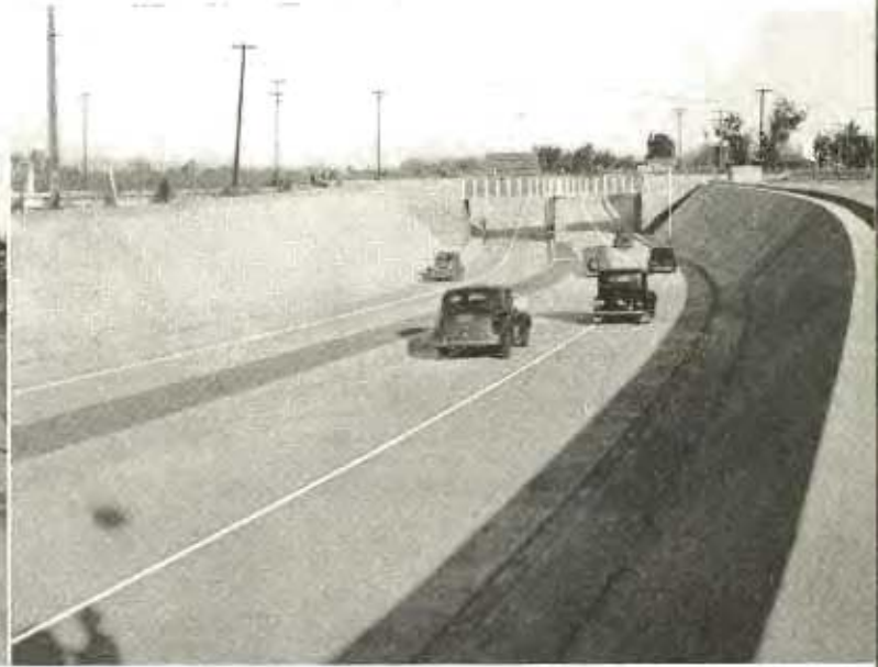
Railroad grade crossing on "S" curve at Livingston on U. S. 99 and underpass with 4-lane divided highway that eliminated it.
