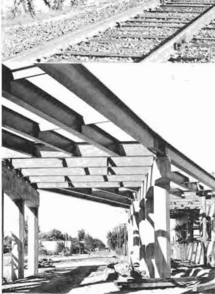
At top—General view of highway overhead structure under construction at Turlock separating grades of Golden State Highway and main line railroad tracks. Lower left shows unique design of placing some girders normal to the piers on skew curve. Bottom—Laying reinforcing steel on bridge deck.
