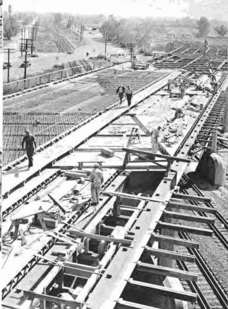
At top—General view of highway overhead structure under construction at Turlock separating grades of Golden State Highway and main line railroad tracks. Lower left shows unique design of placing some girders normal to the piers on skew curve. Bottom—Laying reinforcing steel on bridge deck.
