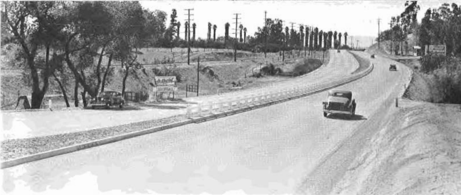
Top—Recently completed divided highway between Colton and Riverside on State Route 43 showing central dividing strip separating old pavement on the left from new lanes on right and guard rail in place where there is considerable difference in elevation. Center—Treatment of dividing strip transition is shown between locations where highways are on different levels. Bottom—Close up of two different level sections.
