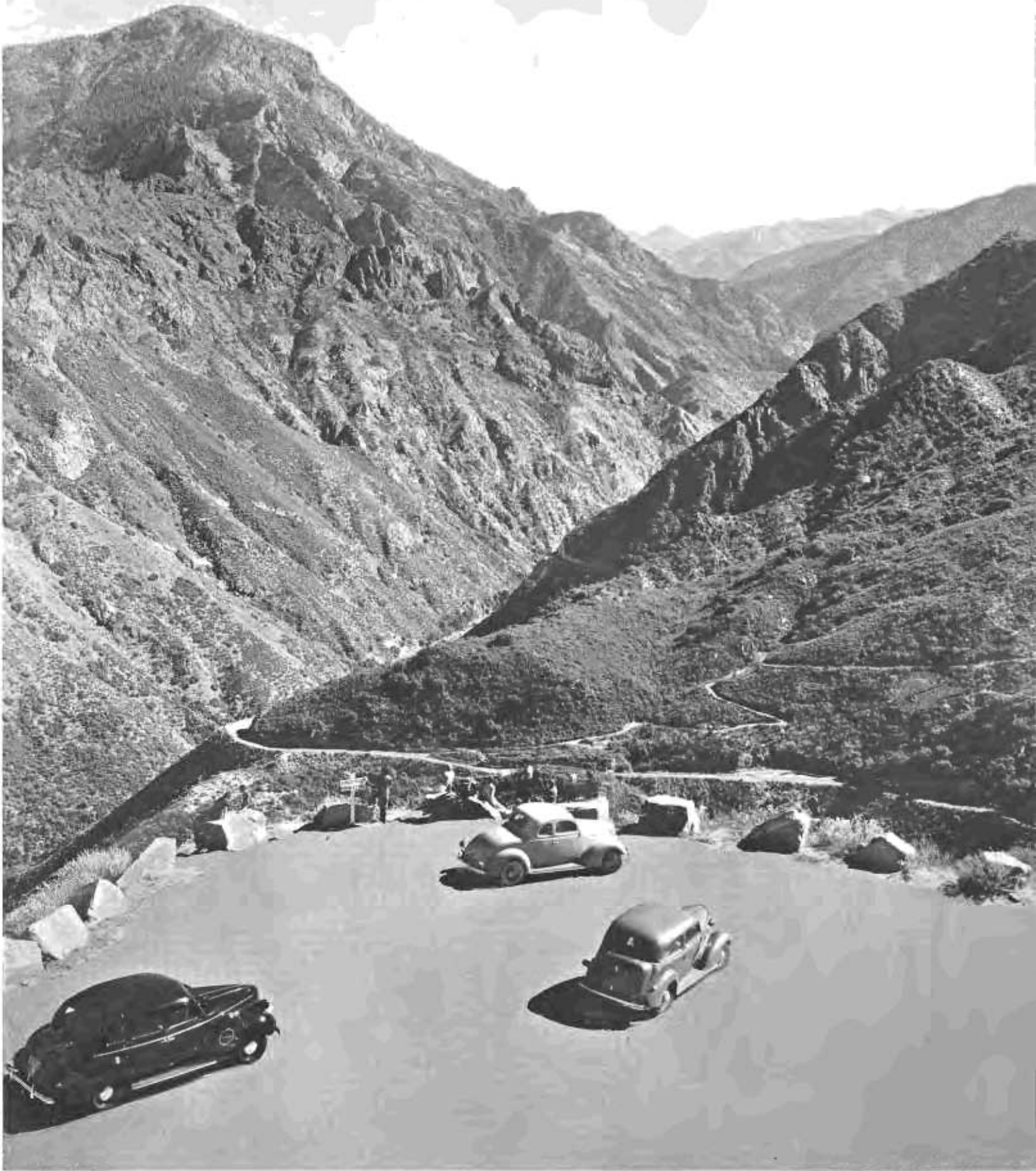
Parking area at confluence of North and South Forks of Kings River showing new highway winding down into South Fork Canyon.
