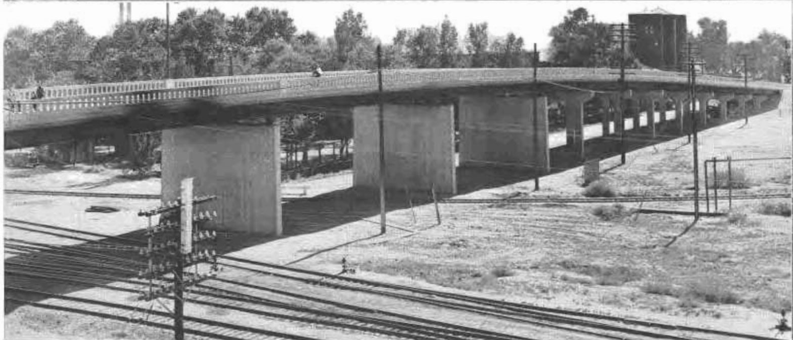
This grade separation structure on Oak Street in Bakersfield carries State Highway 141 over tracks of The Atchison, Topeka and Santa Fe railroad yard. It has an overall length of 1607 feet with a 26-foot roadway and sidewalks and is designed for future widening.
