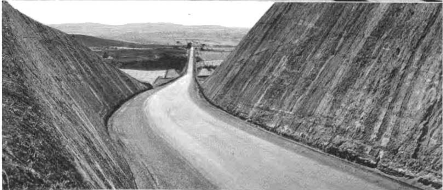
At top—Section of new 22-foot "Industrial Highway" between Willow Pass and Franklin Canyon in Contra Costa County. Center—Grade separation structures carrying county road and railway. Bottom—View looking westerly through deep cut near east end of Willow Pass.
