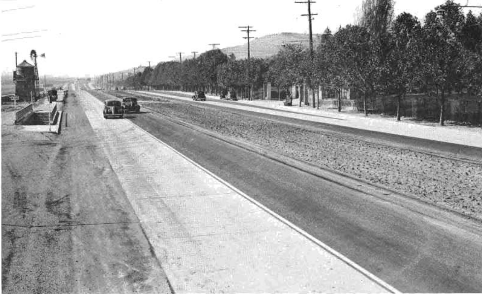
Three and a half mile stretch of four-lane divided highway recently opened with appropriate ceremonies on Foothill Boulevard in Alameda County has 23 feet of roadways on each side of 24-foot, planted division strip
