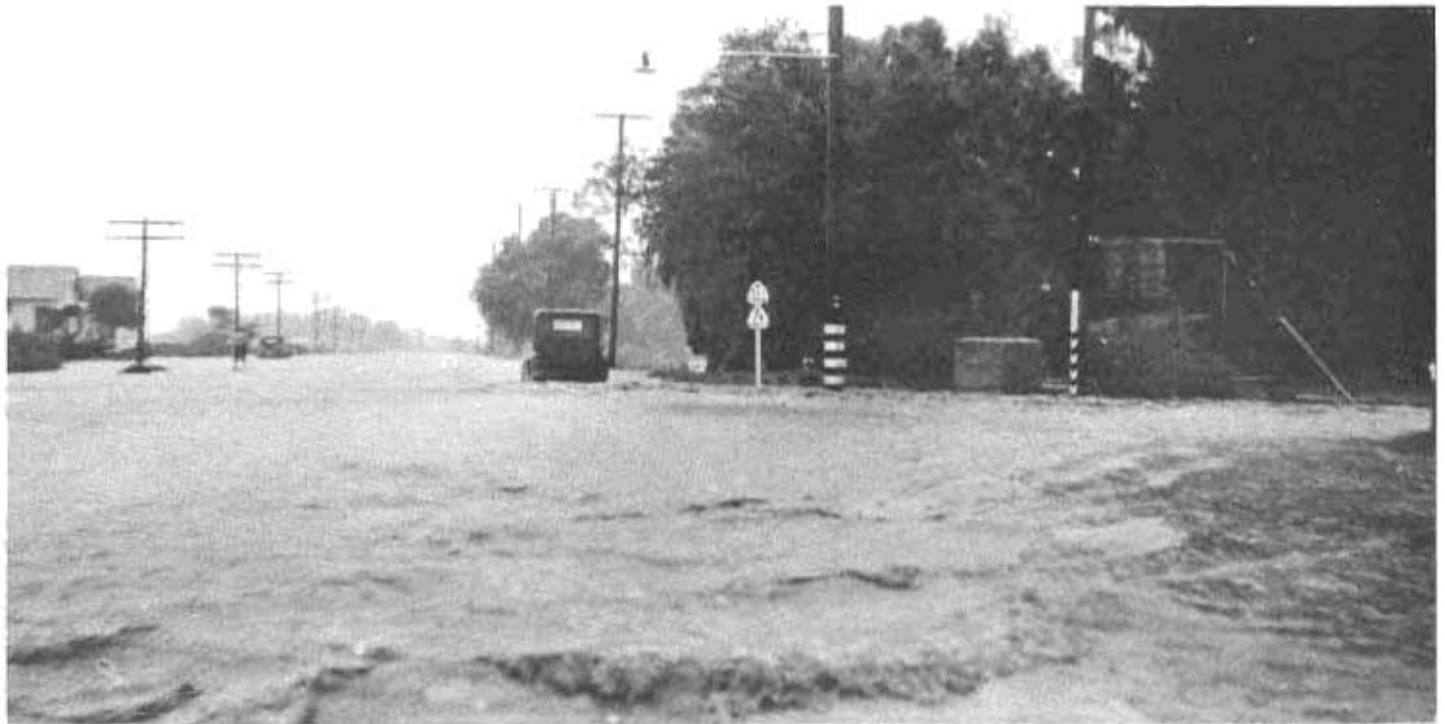
Cloudburst flood scene on Jackson Street in City of Indio, Riverside County, during storm of September 4th
