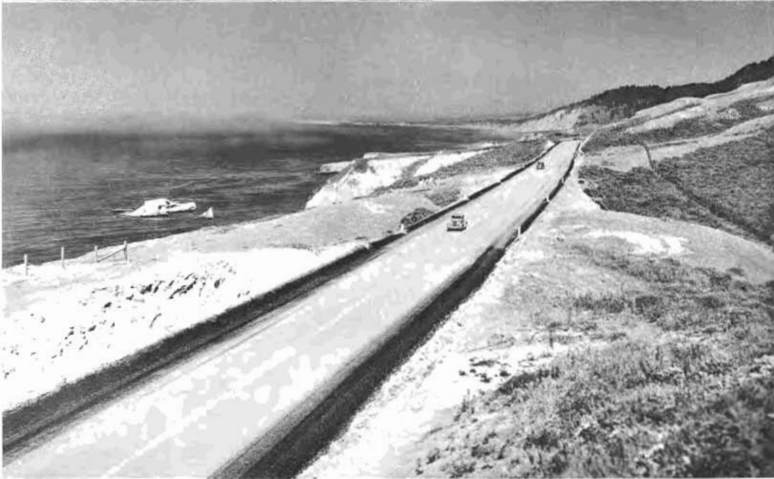
Two views of sections of new State highway along the ocean north of Santa Cruz between Davenport and Waddell Creek.
