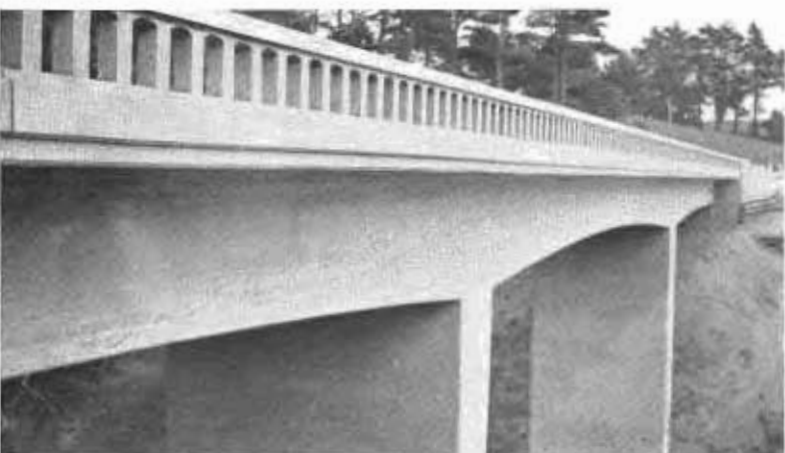
Timber truss bridge, frequently strengthened across Jack Peters Creek replaced by modern concrete box girder span
