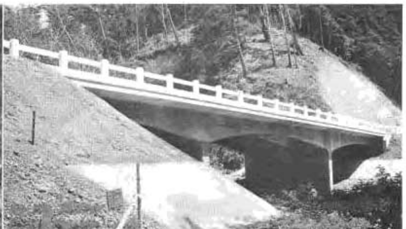
The old timber bridge across Elk Creek with sharp left turn approach was replaced by concrete girder bridge on new alignment.
