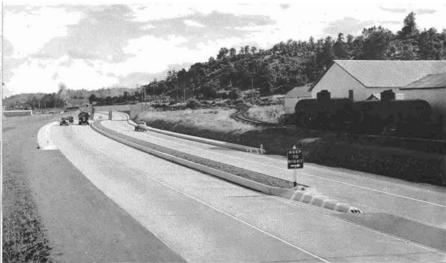
Four lane divided highway underpass with 8-foot division strip near Redding on State Route 3 (U. S. 99) in Shasta County.
