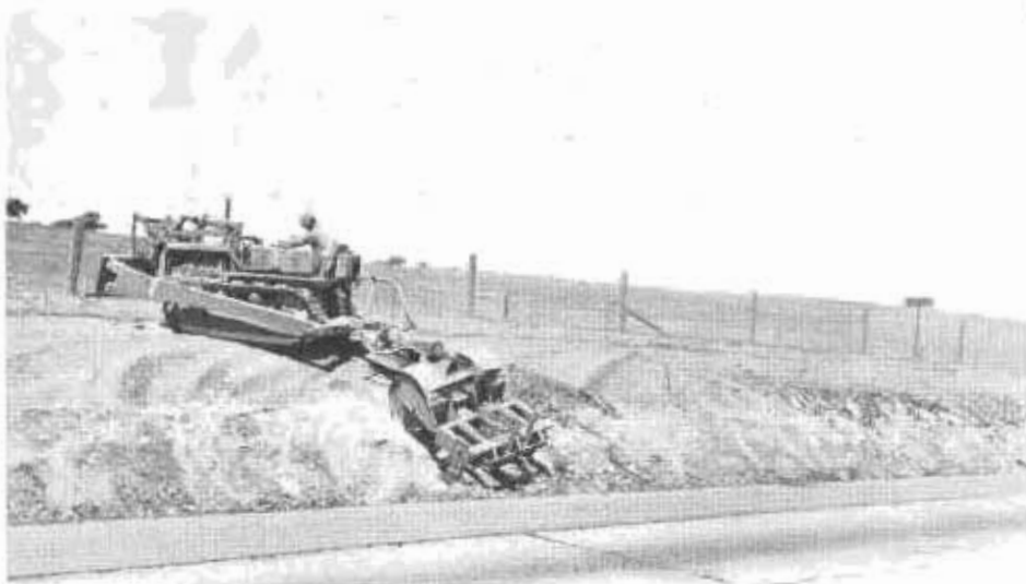
Scarifier attachment behind scraper aids in working rocky formations.
