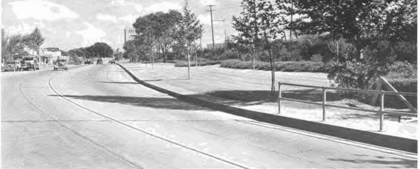
Improved appearance of U. S. 40 approach to M Street bridge, Sacramento, by tree and shrub plantings. Inset shows former conditions.
