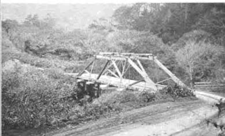
The old timber bridge across Elk Creek with sharp left turn approach was replaced by concrete girder bridge on new alignment.
