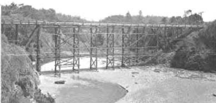
Old timber truss bridge across Jug Handle Creek on State Highway 56 replaced by reinforced concrete arch span at right.
