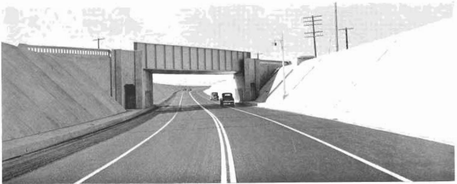
Grade separation at Famosa in Kern County on Golden State Highway (U.S. 99) carrying 2 railroad tracks over a 4-lane highway.
