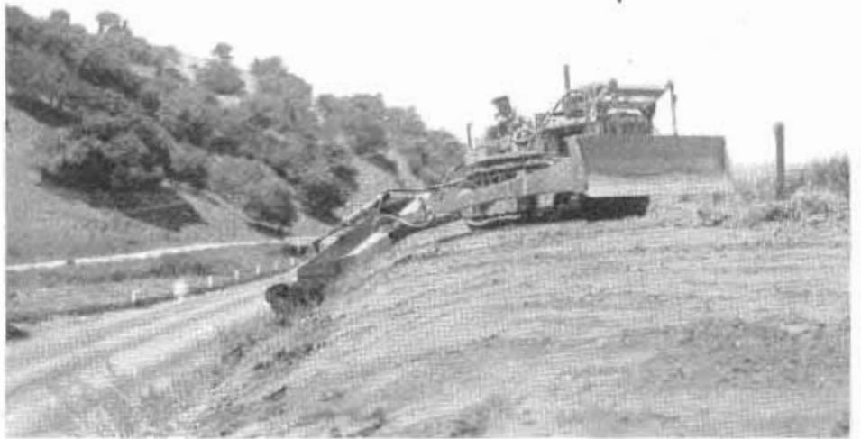
Scraper and bulldozer rounding and leveling top of cut slope.
