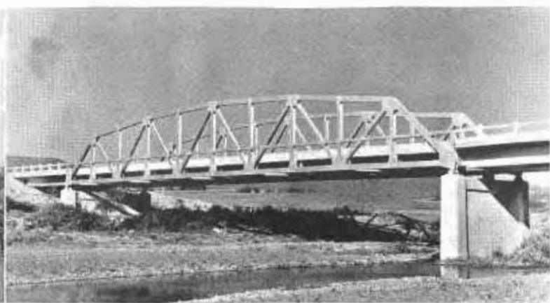
Ancient Garcia River bridge with timber trusses and approaches replaced by 120 foot steel truss span with steel beam approaches
