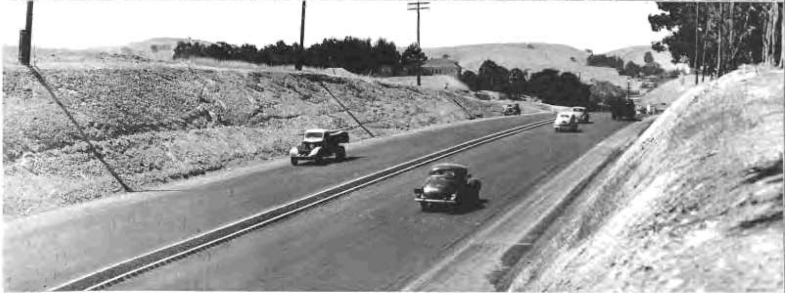
Views of new grade separation on U. S. 40 near Pinole in Contra Costa County where the highway formerly crossed over the railroad tunnel. At top—New divided highway bridge over railroad. Center—New railroad cut. Bottom—Divided highway approach.
