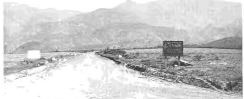
County road to observatory site before rebuilding.
