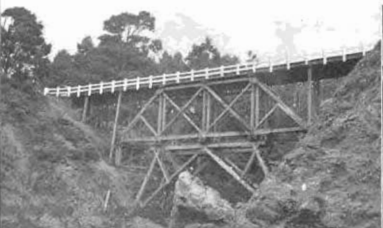
Timber truss bridge, frequently strengthened across Jack Peters Creek replaced by modern concrete box girder span
