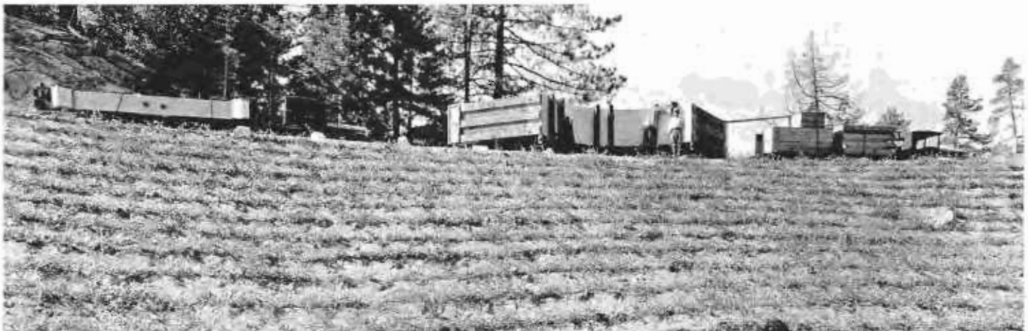
Heavy loads on mountain grade. Center is part of telescope horseshoe weighing 54 tons. Behind it is a large girder.
