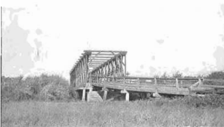
Ancient Garcia River bridge with timber trusses and approaches replaced by 120 foot steel truss span with steel beam approaches
