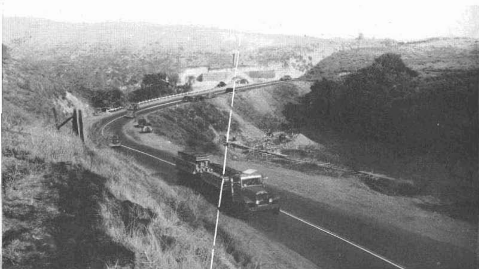
This view of Roosevelt Highway improvement project was taken at Escondido Creek looking easterly.
