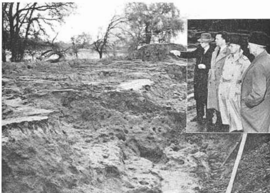
Governor Olson and officials view levee break north of Princeton. In group, Governor Olson, Director of Public Works Frank W. Clark, E. Vayne Miller, Reclamation Board, State Engineer Edward Hyatt (pointing).
