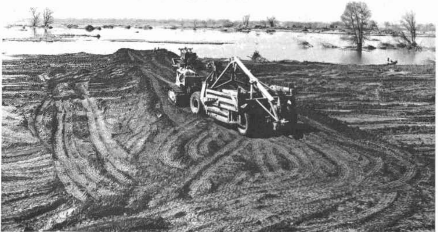
Equipment engaged in repairing levee break along Sutter By-pass near Meridian.
