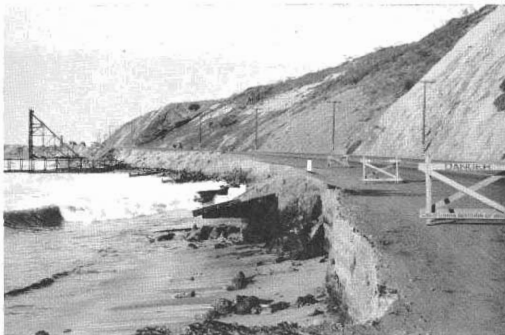
While "Minnie A. Caine" was forming sand bar, tidal currents threatened highway.
