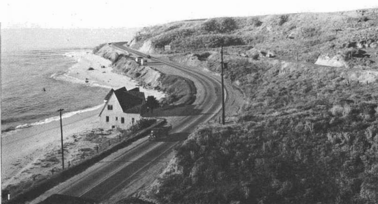
Line change at Latigo Canyon road. New center line shown along right edge of picture eliminates sharp curve around point.
