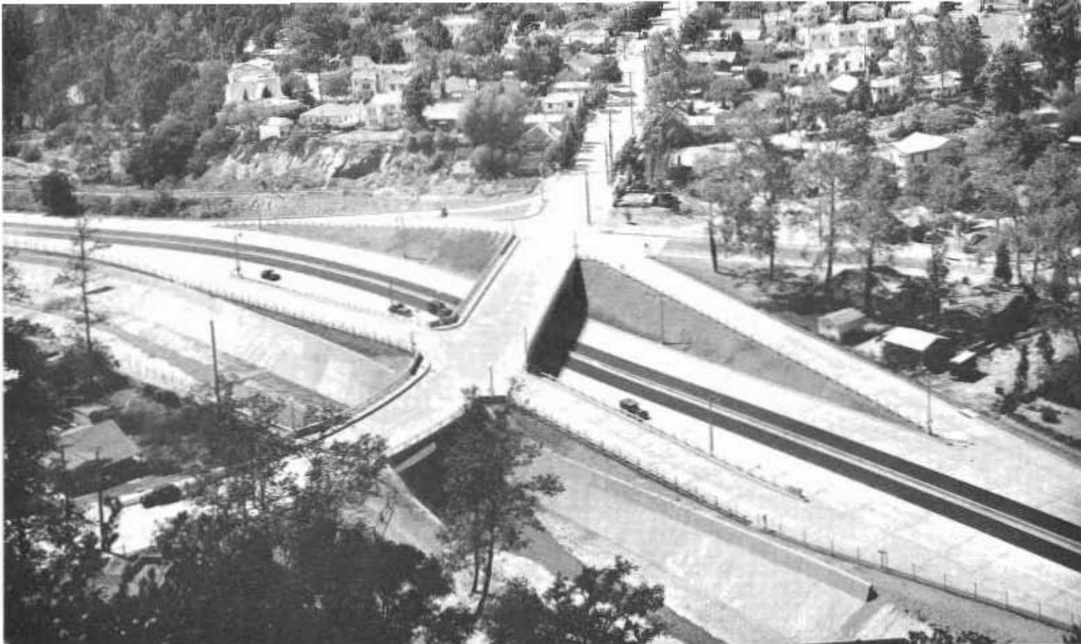
Arroyo Seco Parkway at Avenue 52 is crossed by 2 bridges, one with ramps and other over paved stream channel.
