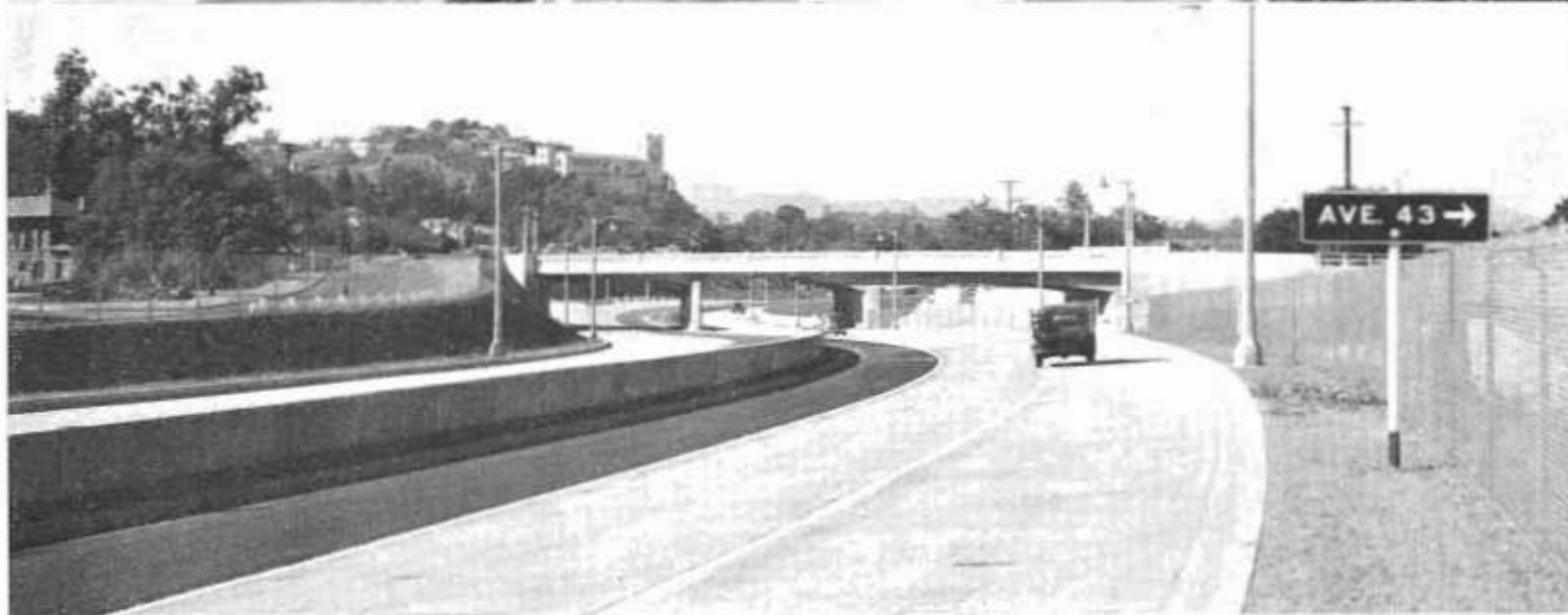
Arroyo Seco Parkway sections between Pasadena and Los Angeles recently opened showing 35-foot divided lanes, bridges and service roads.
