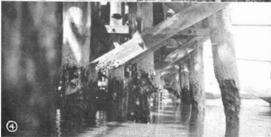
No. 1—Light, narrow bridge posted and likely to collapse if struck by a vehicle out of control. No. 2—Inadequate expansion detail in concrete girder span caused serious cracking. No. 3—Poor concrete in pile coupled with abrasion by floating drift resulted in serious weakening. No. 4—Support piles weakened by marine borers.
