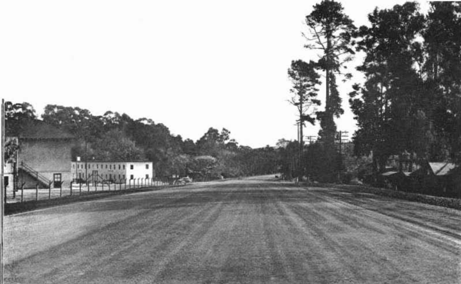
Four-lane approach highway on new alignment to connect with north end of San Rafael Viaduct
