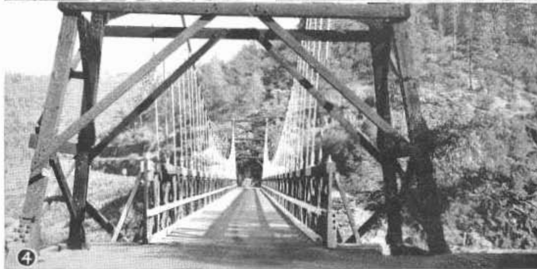
Pictures 1 and 2 show decay in bents of this timber overhead structure evidenced by settlement of the deck. No. 3—A defect in expansion detail of concrete girder structure resulted in disintegration of beam. Note temporary timber supports on shallow footings. No. 4—One-way timber suspension span posted and reinforced by adding additional hangers between originals
