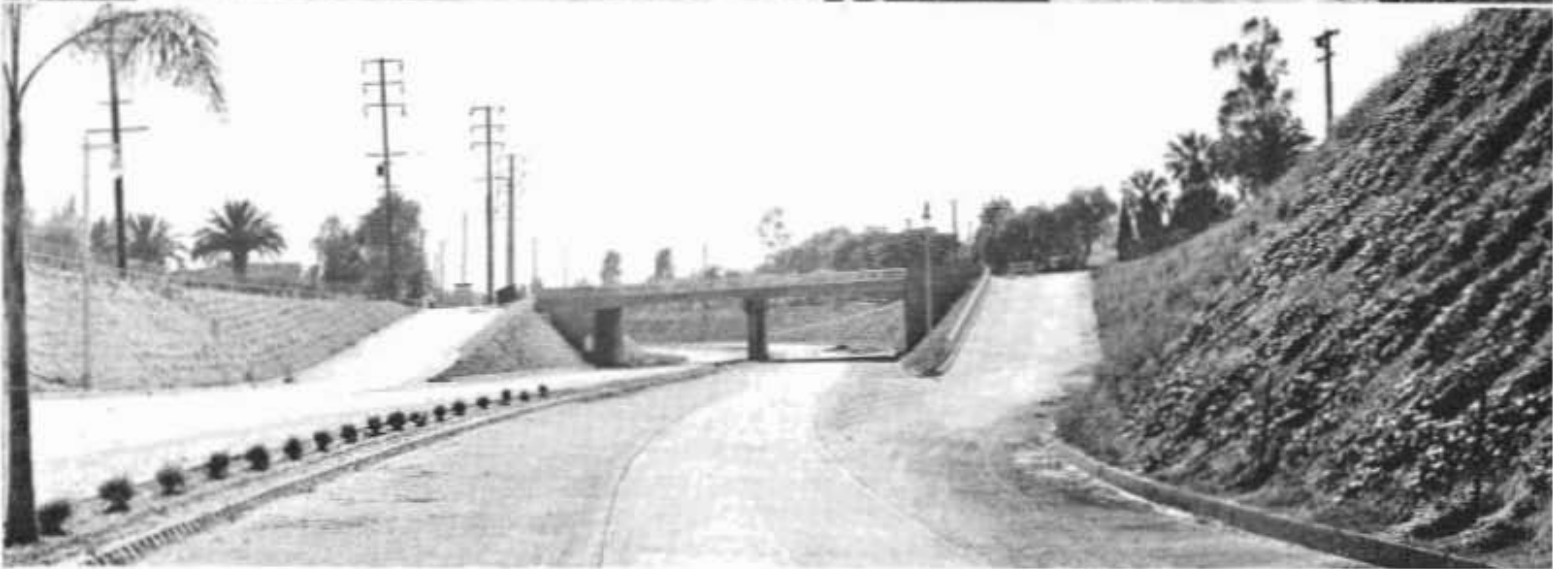
Top and bottom pictures show plantings on slopes of Arroyo Seco Freeway including blue dawn flower, catsclaw, wild grape, trailing lantana, and honeysuckle, with Boston ivy on structure abutments and piers and oleanders and toyons in groups on slope tops. On dividing strips are compact myrtle and ice plant with cocos palms placed at center piers and close to structures. Center picture shows stages of slope planting and application of top soil
