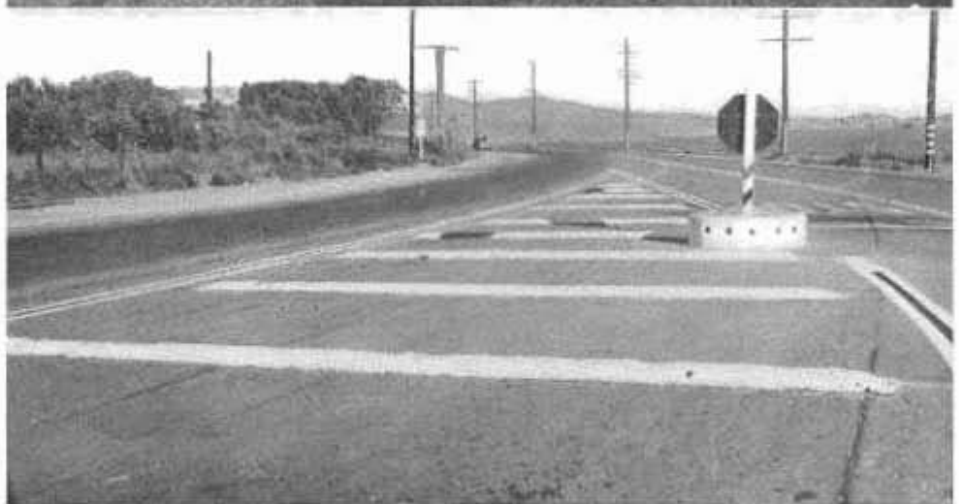
Control and guidance of traffic by raised white bars proves effective for intersections, wyes, neutral strips on divided highways and protection of central placed signs
