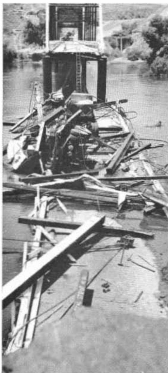
An old timber truss bridge that collapsed under a truck and trailer loaded with a power shovel, both vehicles being considerably over the posted weight limit. The truck and fallen span lie in shallow water.
