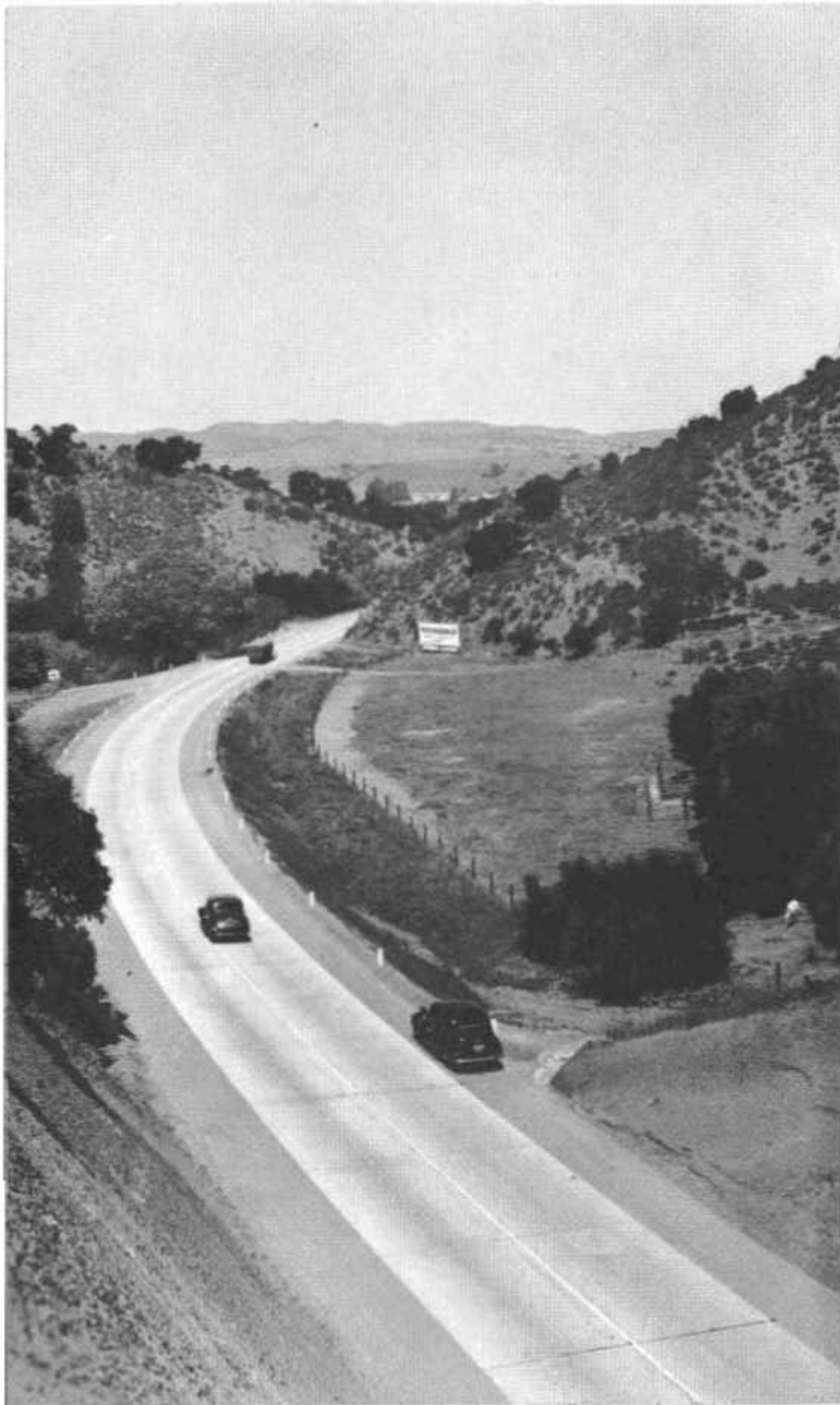
Twenty-two foot portland cement concrete pavement between Gaviota Pass and Santa Ynez River on State Highway Route 2 in Santa Barbara County. The record for cement control was made on this contract, the average variation being only 0.28 per cent. The average variation on State contracts during the year 1939 was 0.58 per cent.
