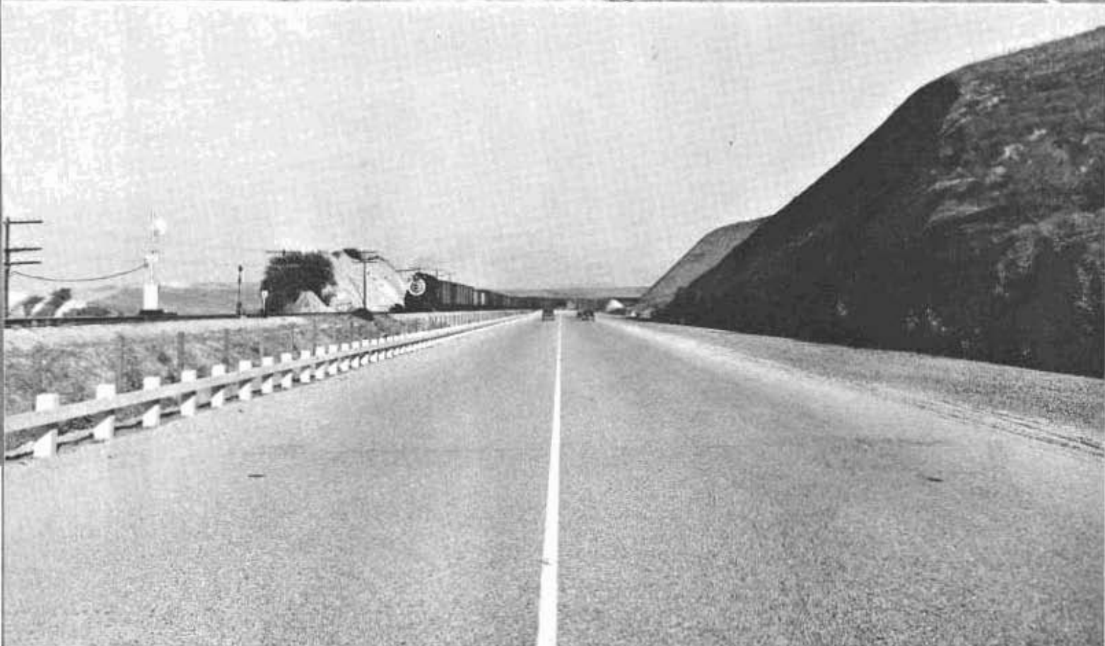
Relocation of the Santa Ana Canyon Highway necessitated by construction of Prado Dam across the Santa Ana River for flood control in Orange County between Corona and the Orange County line, takes the highway and Santa Fe Railroad, both of which were flooded in 1938, high above the river. In addition the more direct route shortens the distance about a mile and eliminates many sharp and dangerous curves.
