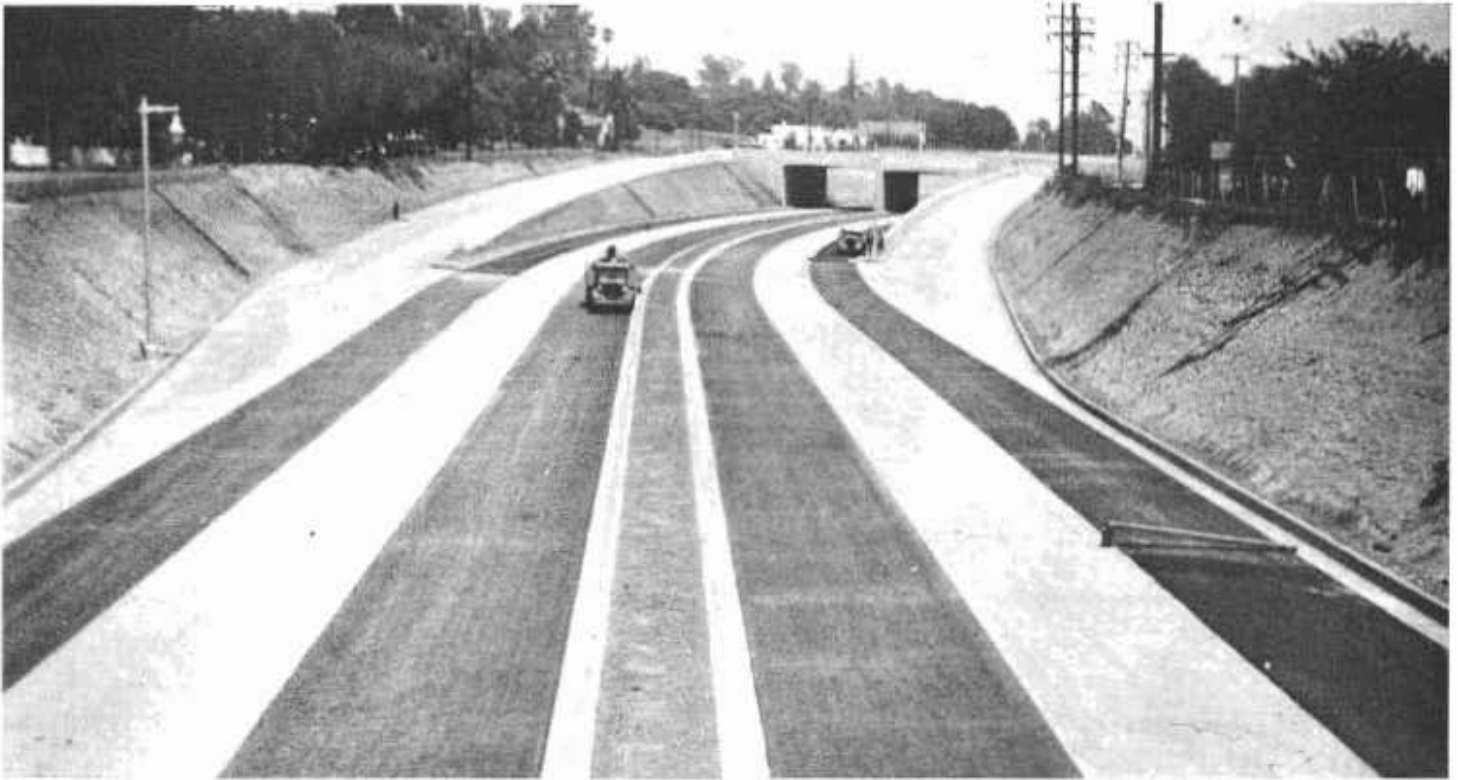
Six-lane free-way with 11-foot asphalt concrete, portland cement concrete, and plant-mix pavement strips on Arroyo Seco Parkway between Los Angeles and Pasadena.
