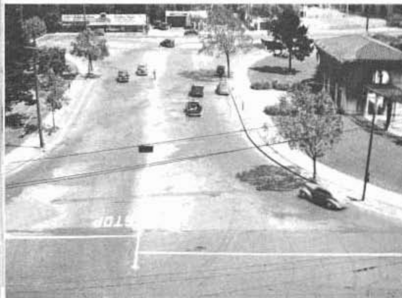
El Embarcadero between Grand Avenue and Lakeshore Avenue, a wide, high traffic count street transformed into 2 lanes separated by a small park.
