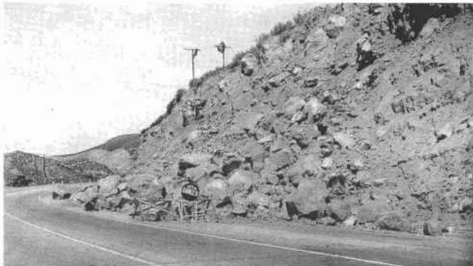
Slide on Ridge Route, Los Angeles County, in 1938 storm.
