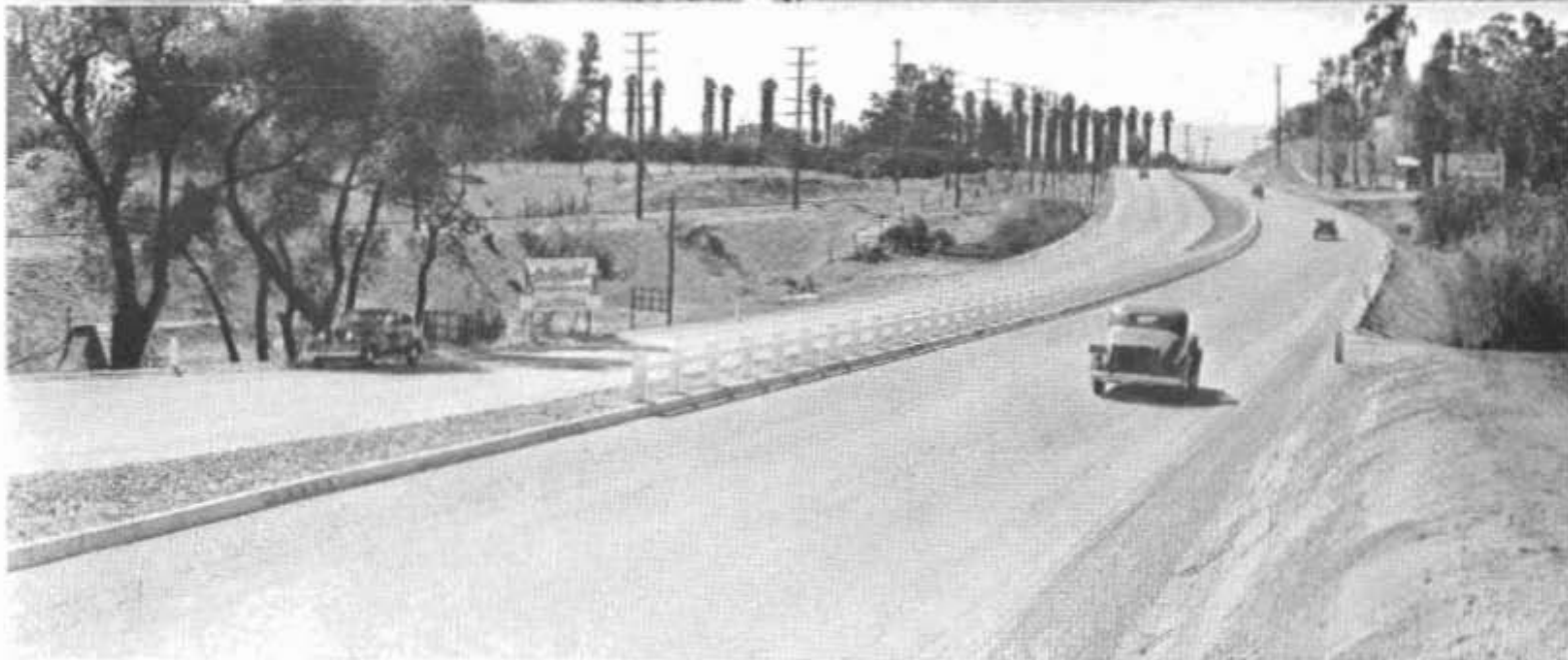
Divided highway with two 23-foot road-mix surfaced lanes between Colton and Riverside on Route 43 in Riverside and San Bernardino Counties.
