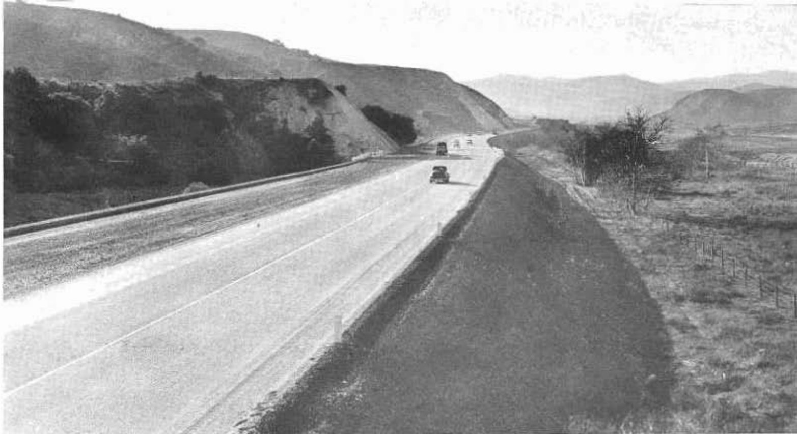
New highway in Santa Ana Canyon graded for ultimate 4-lane divided highway section with surfacing for two lanes completed. Oil-mix berms on right prevent slope erosion.
