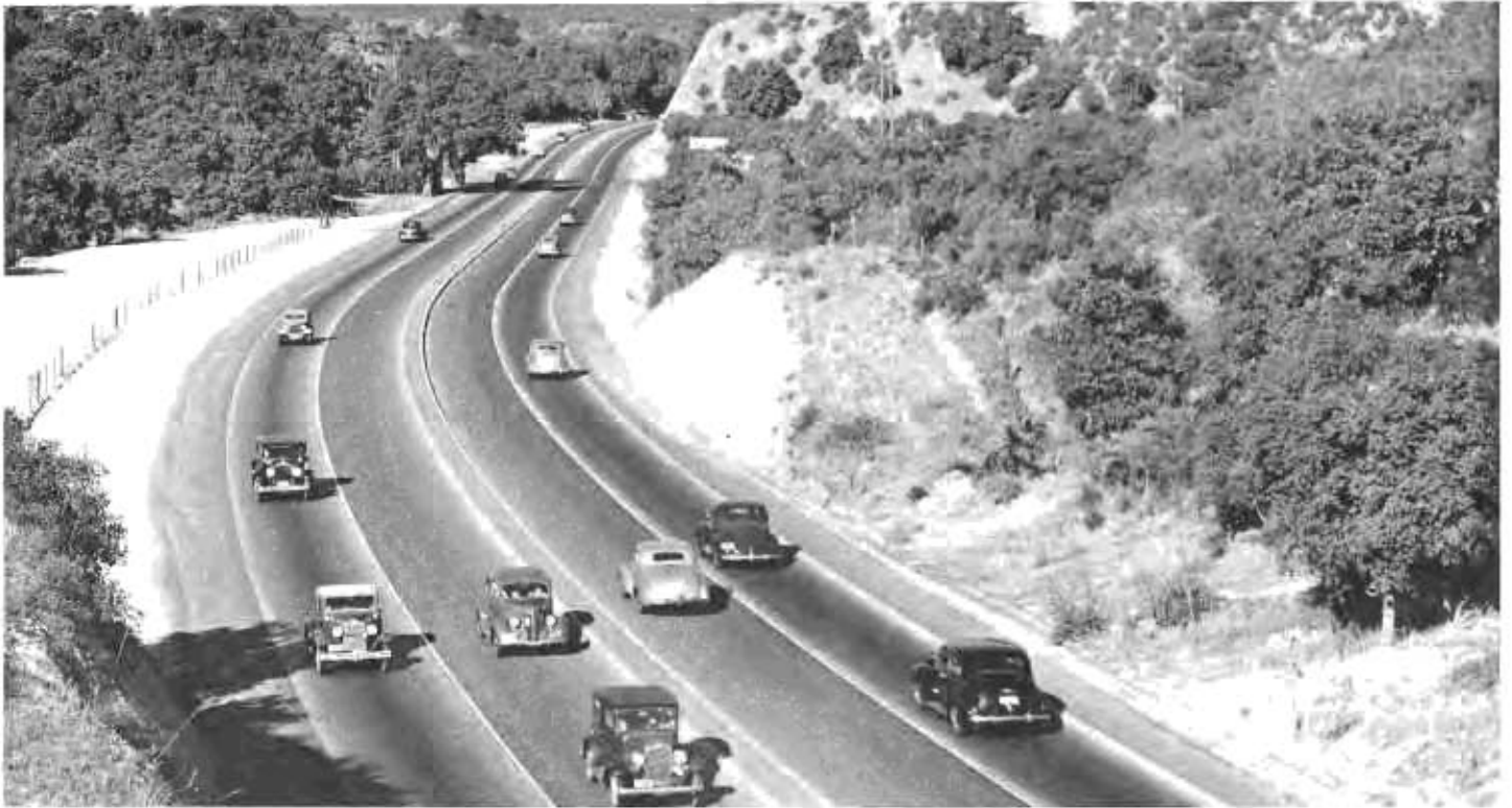
Modern 4-lane section of Newhall Tunnel highway has a raised central dividing strip covered with plant-mixed surfacing.
