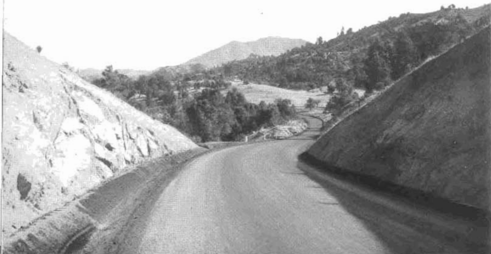
Portion of recently completed section of State highway realignment through Tehachapi Pass between Bakersfield and Tehachapi.
