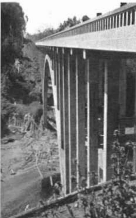
Russian Gulch Bridge, a graceful spandrel arch structure 526 feet, 9 inches long on the Mendocino Coast highway was dedicated June 9 when Secretary of State Paul Peek cut the ribbon. The old structure was a timber trestle built 30 years ago.
