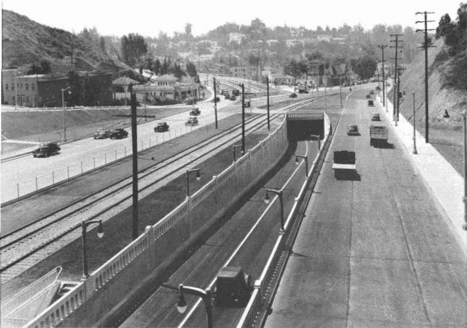
View of Cahuenga Freeway looking southeasterly, showing underpass beneath Pacific Electric tracks at intersection of Highland and Cahuenga avenues.
