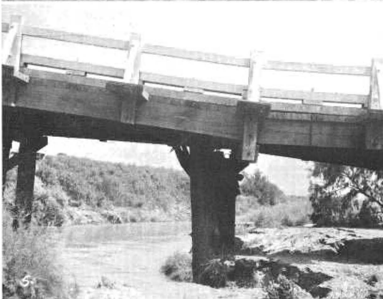
Pictures of earthquake damage to the State highway system in Imperial County. No. 1—Settlement of 18 inches in the approach to New River bridge. No. 2—Pavement shattered west of Brawley. No. 3—Pavement cracked east of Ash Canal. No. 4—Sixteen-inch offset in pavement on Route 27. No. 5—Timber piles shoved from beneath caps of New River bridge. No. 6—Horizontal shift of nine feet where fault line crosses Route 202.
