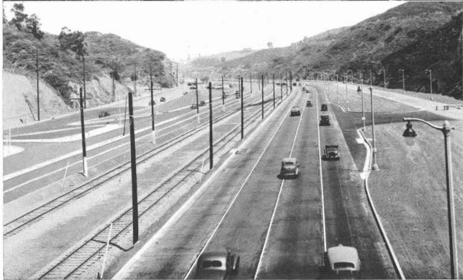
Views of Cahuenga Freeway with 8 traffic lanes divided by Pacific Electric tracks. At top—looking north from Cahuenga-Highland intersection showing Pilgrimage Play bridge in background and subway underpass to Cahuenga Avenue. At bottom—looking north from Pilgrimage Bridge. Note entrances to service roads on right and left with intersectional islands.
